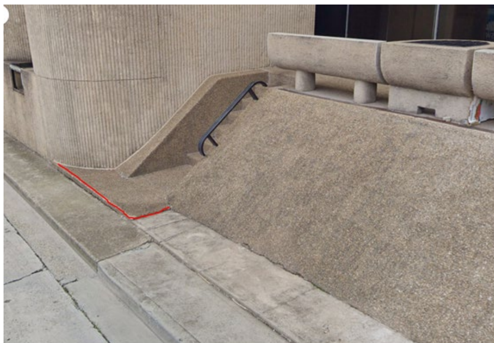
Figure 2 – Area of works, note red marking
