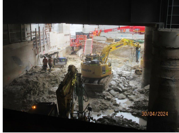
Figure 3.2 Pymont East: Excavation of sandstone using rock hammers under sttel deck
