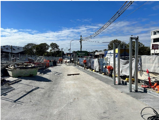
Figure 1 5 Hardstand in place between station box and Parramatta Road (Burwood North).
