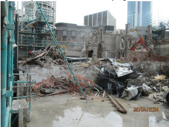
Figure 3.5 Hunter St East: Demolition works ongoing.
