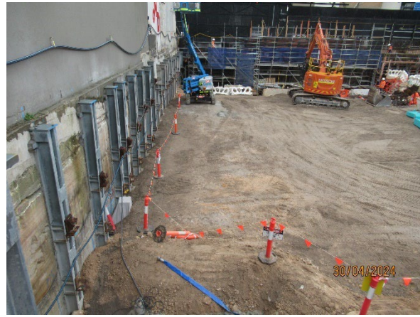
Figure 3.4 Pymont West: Piling pad completed for piling.
