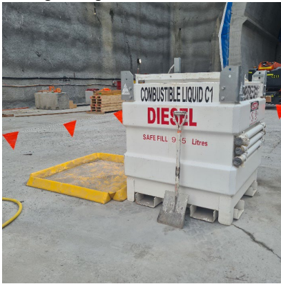
Figure 2.15: SOP Site – station box refuelling
