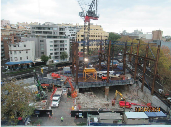
Figure 3.1 Pymont East: Ongoing installation of the acoustic shed.
