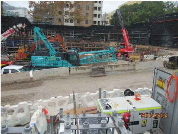
Figure 3.3 Pymont West: Crane on site for piling works.
