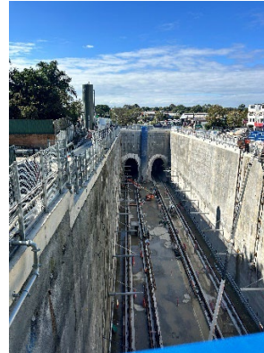
Figure 1 4 Preparation for TBM arrival (Burwood North).
