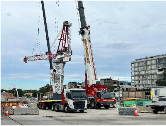
Figure 2.5: Clyde Dive site – Tower crane assembly
