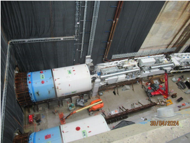
Figure 3.7 The Bays: Assembly of the TBM sections into the station box
