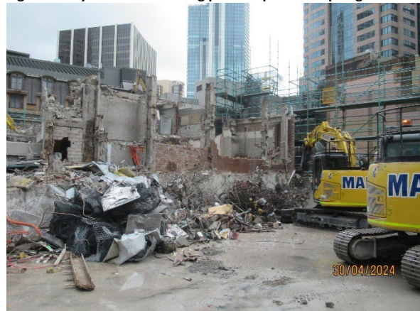
Figure 3.6 Hunter Street East: Demolition of 33 Bligh Street Building.
