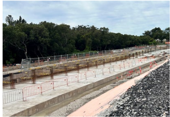
Figure 2.14: Clyde MSF Site – Utilities retaining wall excavation after rainfall event
