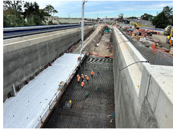
Figure 2.6: Clyde Dive site – Dive base FRP
