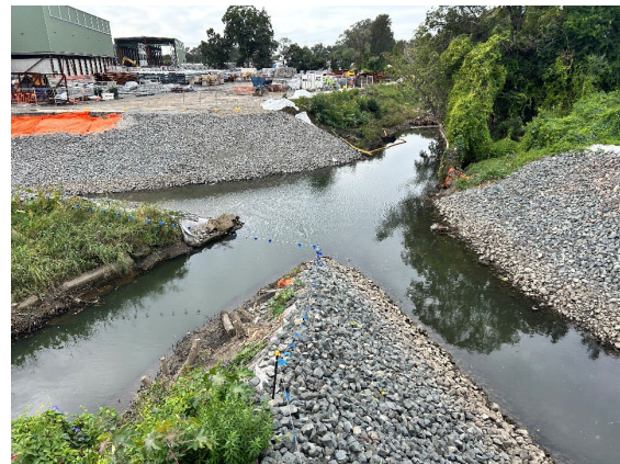
Figure 2.12 – Clyde MSF Site – A'Becketts and Duck Creek tie works
