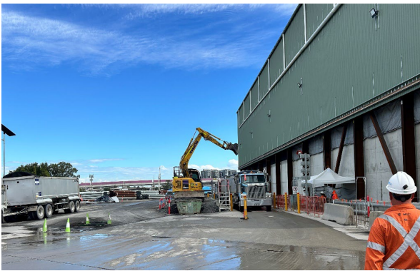
Figure 2.7: Rosehill Site – Internal haul roads and wheel wash
