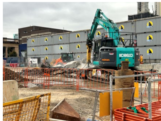
Figure 2.4: Parramatta site – western piling pad removal
