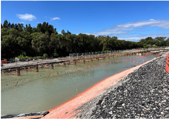
Figure 2.13: Clyde MSF Site – Utilities retaining wall excavation being used as water storage during rainfall event
