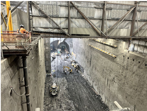
Figure 2.1: Westmead Site –Station box excavation looking west
