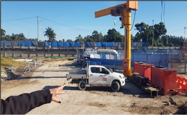
Claremont Meadows view west – Noise blankets above hoarding extended south for OOH concrete deliveries.
