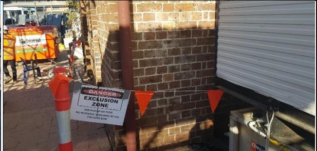
St Marys – Heritage exclusion bunting and signage around Goods Shed.
