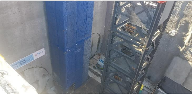
Aerotropolis Station Box north – TBM tunnel breakthrough face preparations completed.
