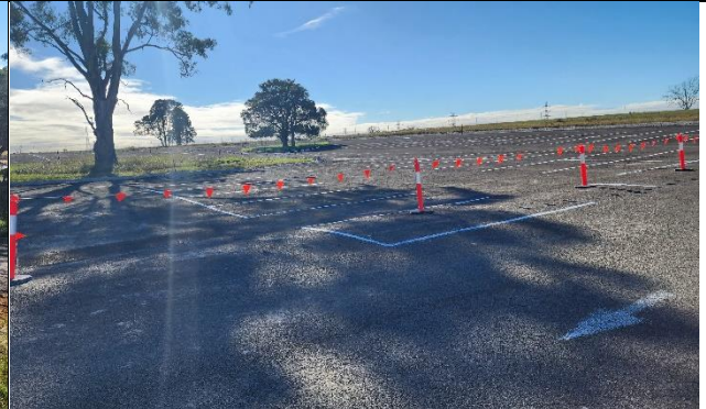
SMF – Light Vehicle car park completed
