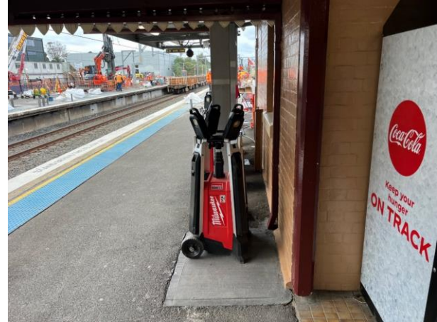
Platform 3/4 - All items were stored off the walls of existing structures
