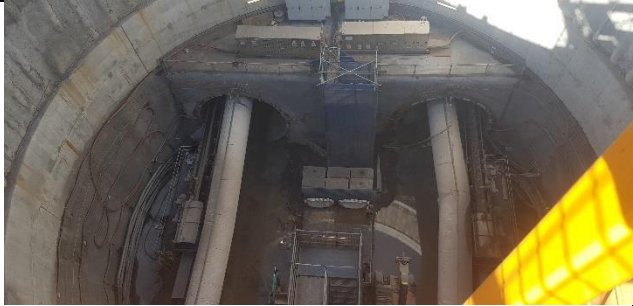
Bringingelly – Works within shaft.
