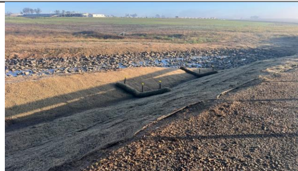
Main Haul Rd - Upstream and downstream of the culvert are now compete reducing the ERSED risk
