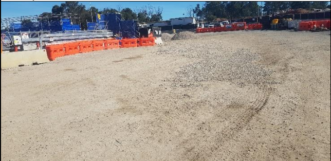
Aerotropolis view west – TBM retrieval working/loading area.
