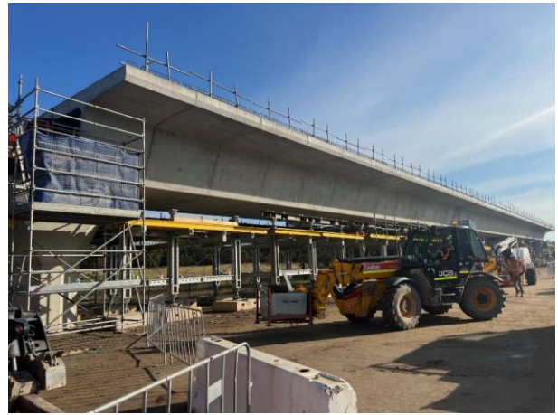
Defence - Viaduct construction using falsework continues
