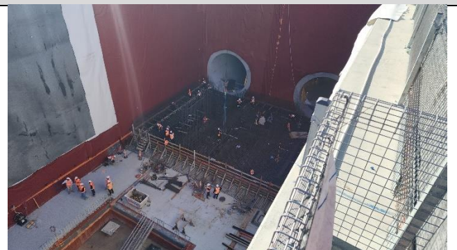
STM – Box formwork preparation for concrete pours
