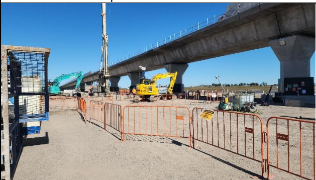
LUD –Piling works had commenced
