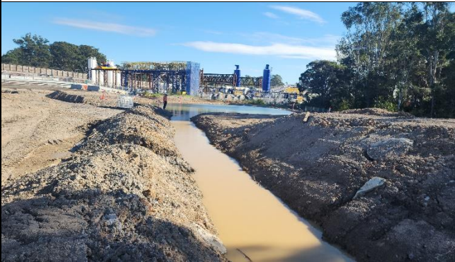
ORH –The turkey nest was approaching maximum capacity after an earth plug was removed from a swale.
