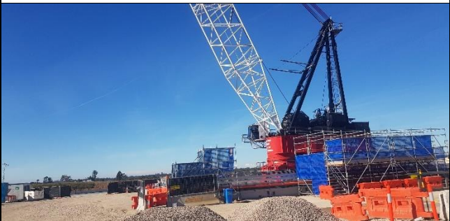
Aerotropolis view east – Mobile crane erection completed.
