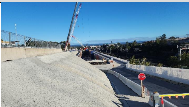
STM – View of box and cranes operating from Glossip St gate
