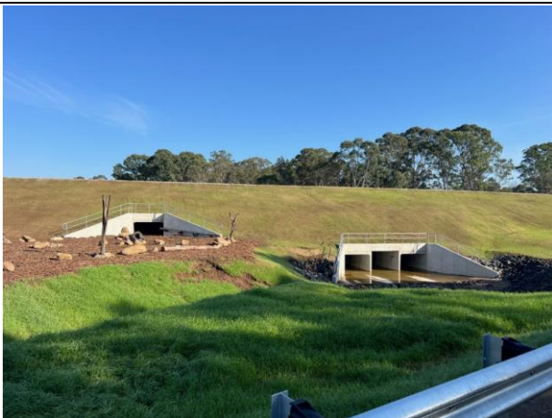
Unnamed Tributary - Finishing works at the unnamed tributary are largely complete
