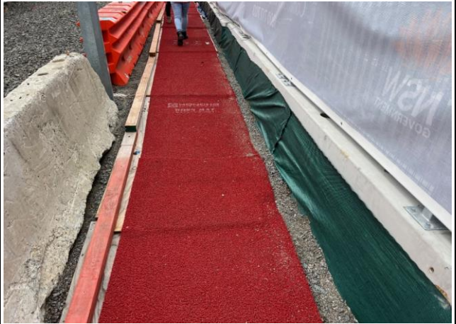
Compound - The red carpet walkway was again utilised to minimise foot tracking of mud
