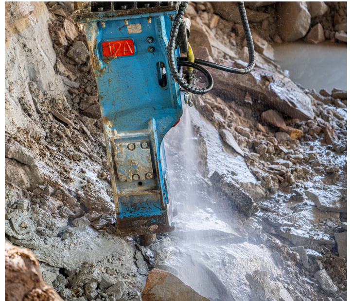
Water mist is used to control dust during hammering activities.
