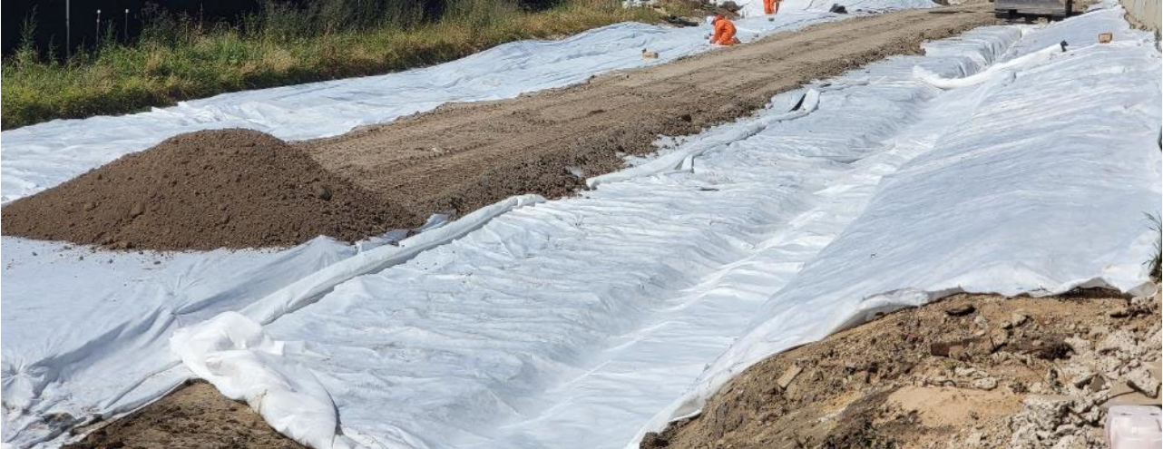
Image 6.2.1.2 View of subgrade material placed across public road portion.
