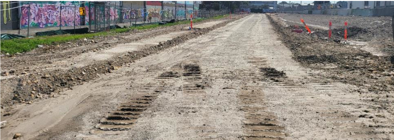
Image 6.2.1.3 View of asphalt emulsion placed across road portion.
