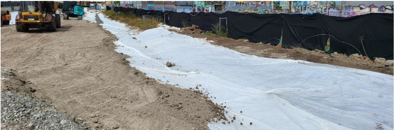
Image 6.2.2.2 View of subgrade material placed across landscaped area.
