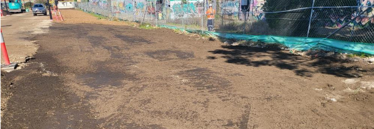
Image 6.2.2.3 View of topsoil material placed across landscaped area.
