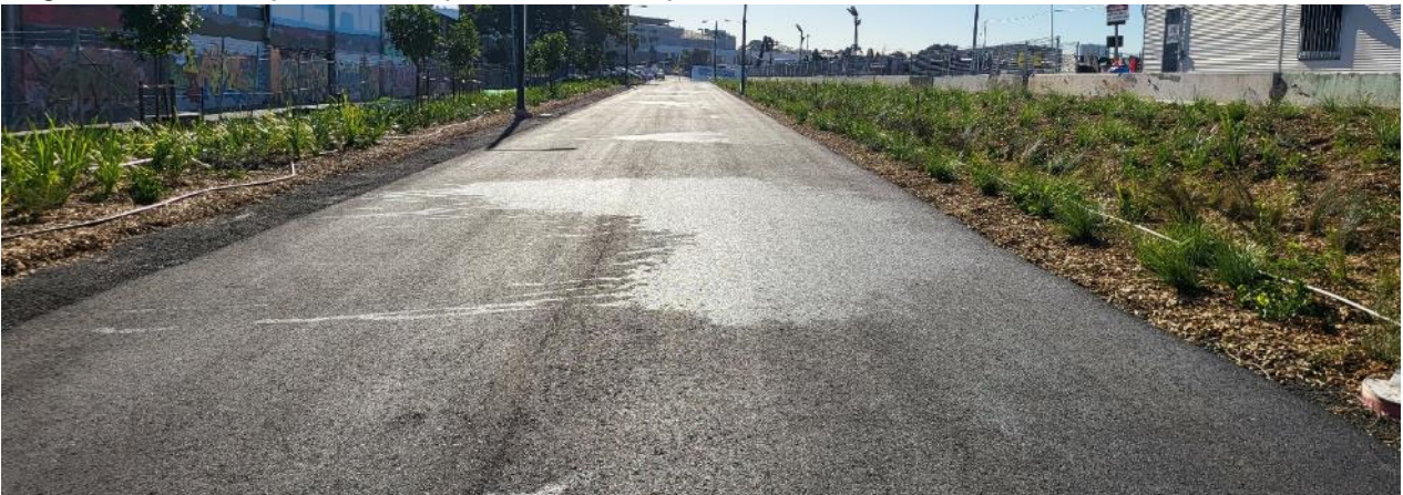
Image 6.2.1.3 View of asphalt emulsion placed across road portion.
