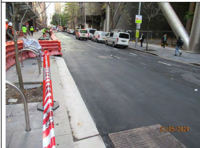
Martin Place North: New pavement installed in Castlereagh Street.
