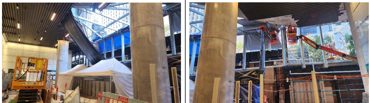
PSN – installation of façade and preparation for glazing.
