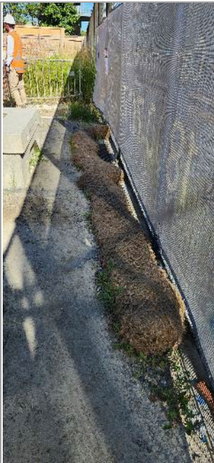
Photos 9-12: Erosion controls in place at drains
