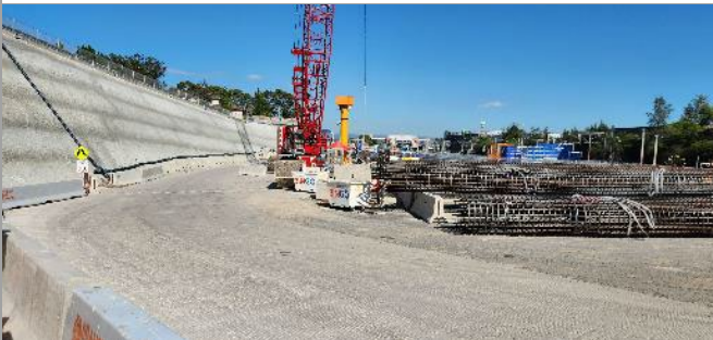
Photo 5 – St Marys station site – generally neat and tidy
