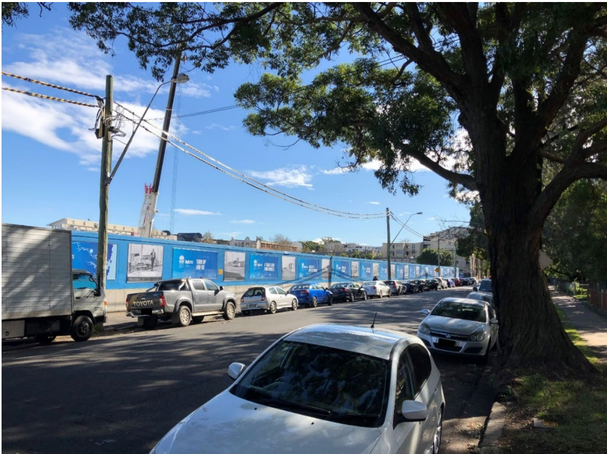
Figure 8.3.6.1: Viewpoint 6 – Existing view north from Cope Street
