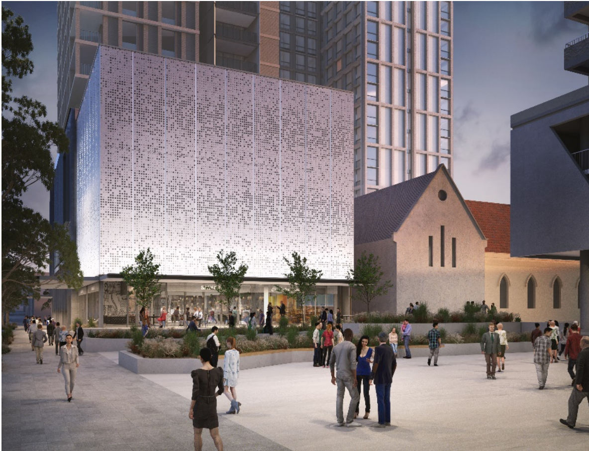
Figure 6.3.1: An artist's impression of the southern station box from Cope Street plaza
