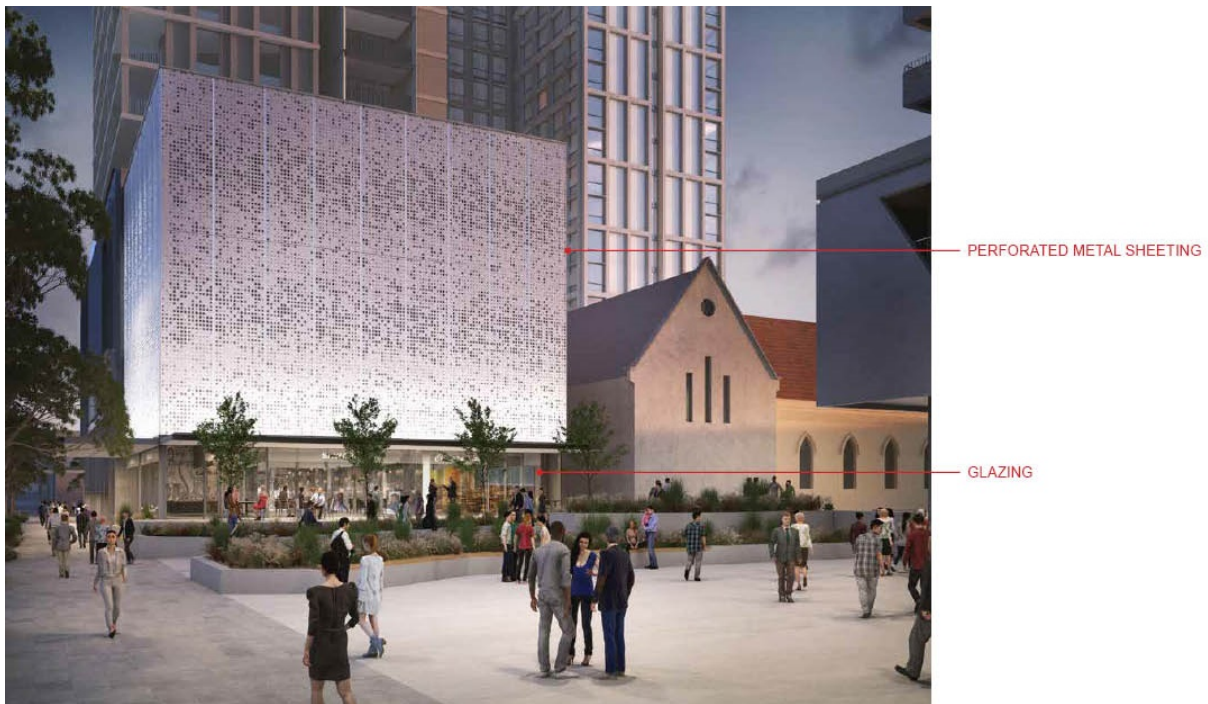
Figure 6.1.2.5: An artist's impression of the southern station building façade finishes from Cope Street plaza
