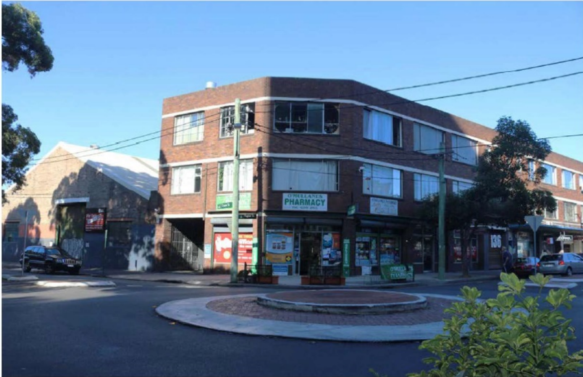
Figure 8.3.4.1: Viewpoint 4 – View southwest from corner of Cope and Raglan streets (from EIS before demolition)
