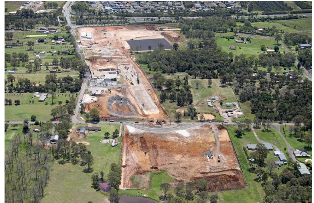
In progress: View of construction work at the new Orchard Hills Station, part of Sydney Metro – Western Sydney Airport.
