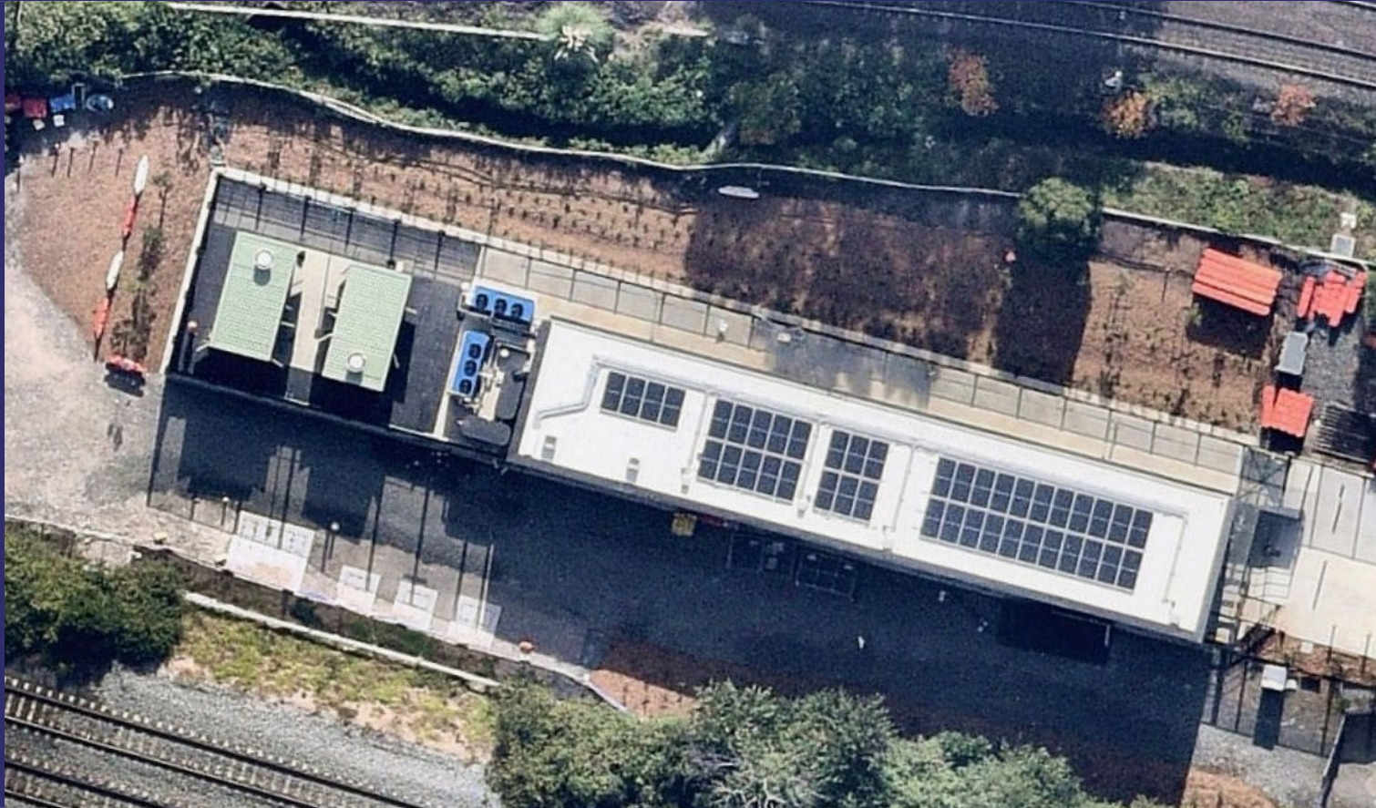
Renewable energy: Solar panels at Marrickville Station service building.
