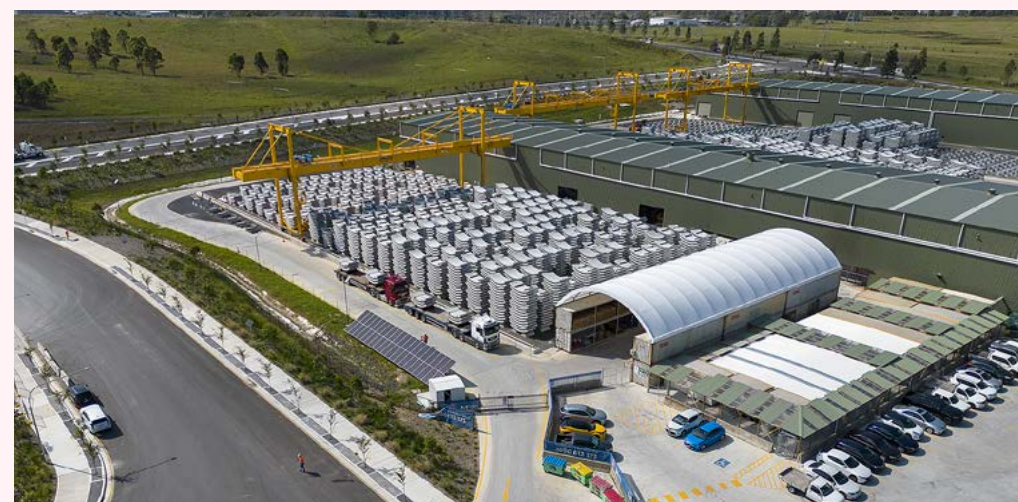
Manufacturing segments: Eastern Creek precast facility where over 60,000 segments will be manufactured.
