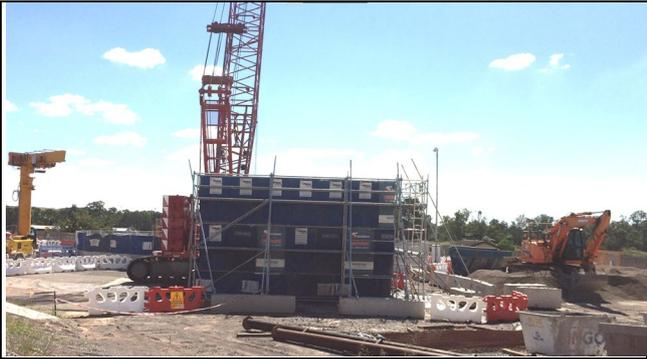
**Bringelly Facility view north west** – Crane noise mitigation structure well installed.
