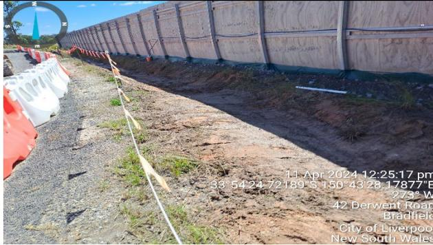
**Bringelly Facility view west** – Swales reshaped and sediment noted by ER addressed immediately.
