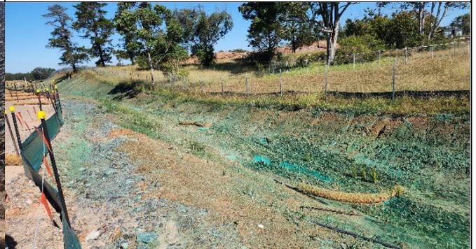
**AEC** – Soil binder applied to the clean water diversion drain
