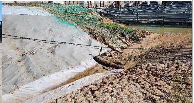
**ORH** –removal of accumulated sediment was required on the SBT boundary. Soil binder had been applied to the embankment.
