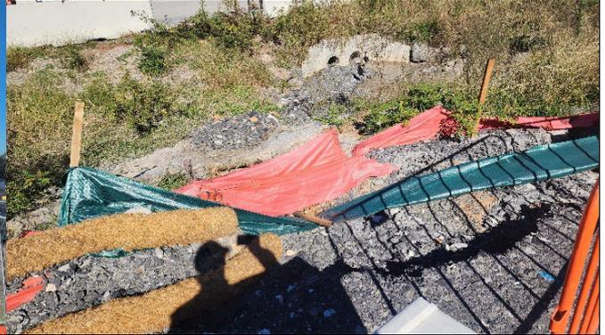
**SMF** – Maintenance of ESC and removal of sediment from internal swale was required.
