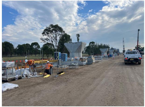
**Defence** - Installation of falsework for viaduct construction continues
