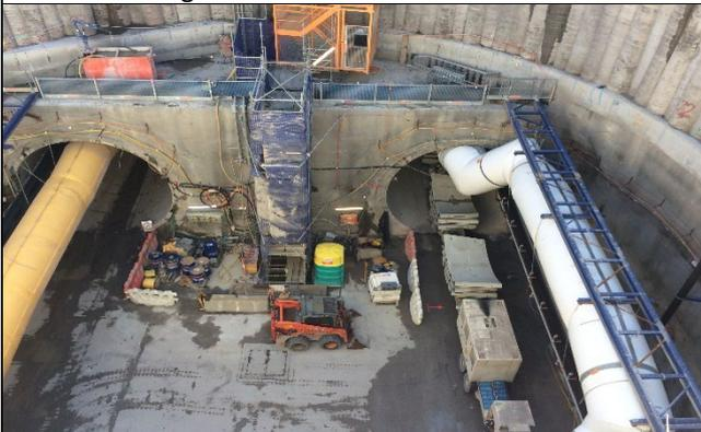
**Claremont Meadows shaft view north** – Tunnel segment loading into tunnel.
