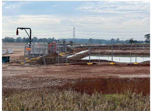
**SMF** - A designated overflow point from the SSTOM basin on the SMF is required to allow SCAW to direct this water into a drainage line
