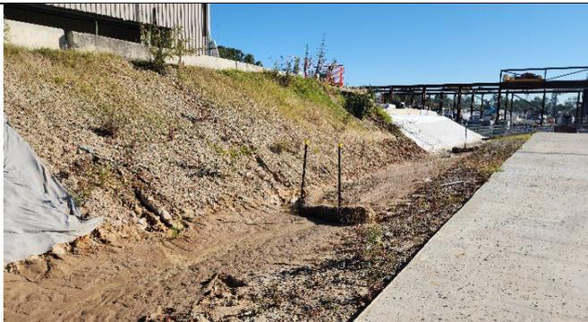
**ORH** –Erosion and sediment controls required maintenance. A 30m section of the embankment was pending the application of soil binder.
