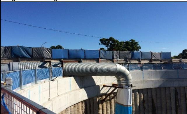
**Claremont Meadows shaft view west** – Noise blankets installed above hording in accordance with DNVIS.
