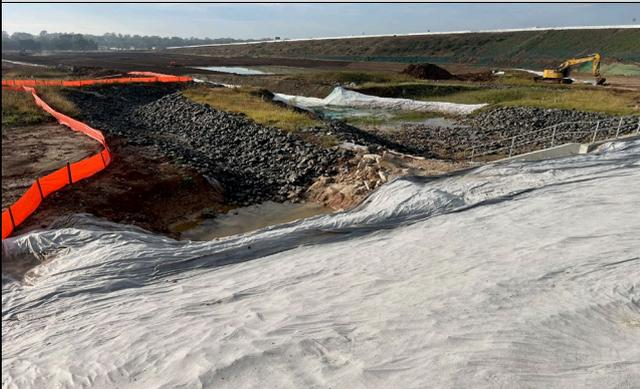
**M12 Interface** - The main drainage line has held up well following the significant rain event
