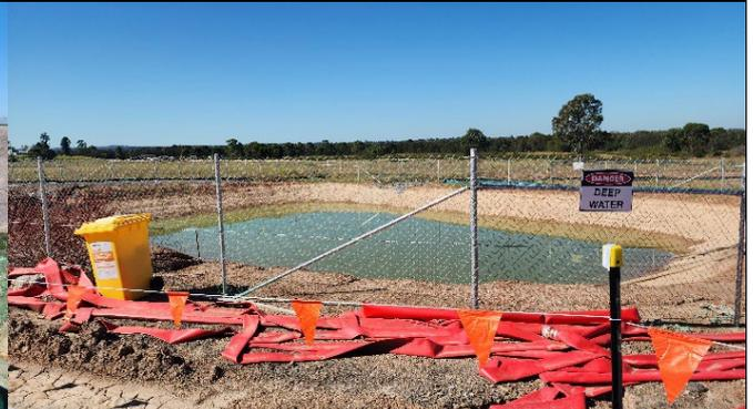
**AEC** – sediment basin was maintained and pumped out.
