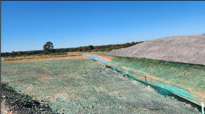
**AEC** – Soil binder applied to clean water diversion drain an area adjacent to the sediment basin
