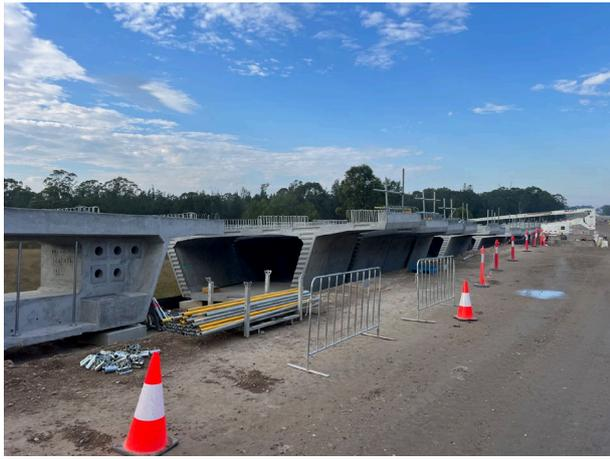
**Defence** - Viaduct segments are stored on the Defence batter for placement on the falsework
