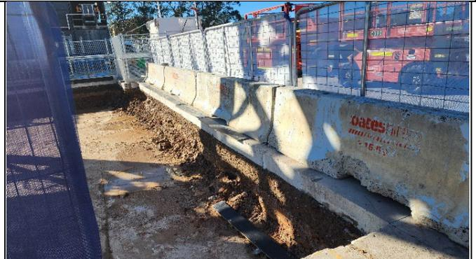
**STM** – Tower crane slab required ERSED controls. PLM noted that this area was scheduled for shotcrete
