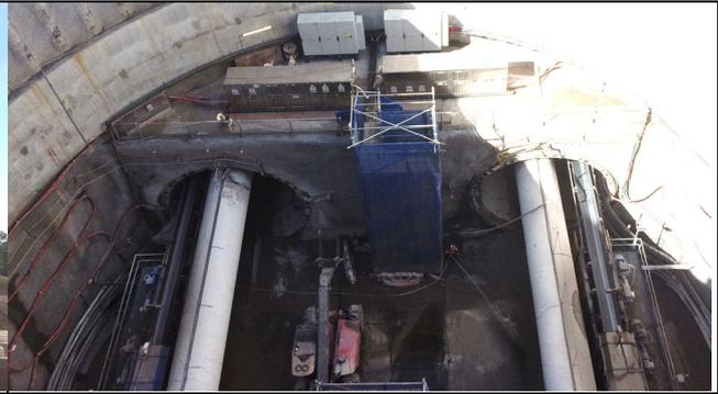
**Bringelly facility** - Installation of tunnel ventilation and spoil conveyor boosters completed.
