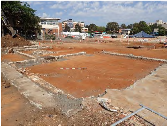
Figure 5.11 Concrete footings in the southern portion of the investigation area.
