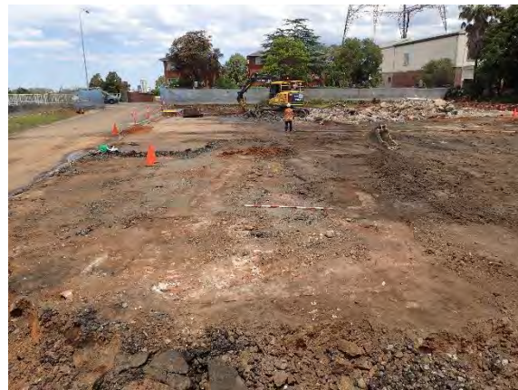
Figure 5.2 Mixed fill present across the investigation area underlying the modern surface.
