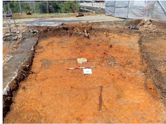
Figure 5.12 Remains of the foundation trench of the bay window for Penzance.
