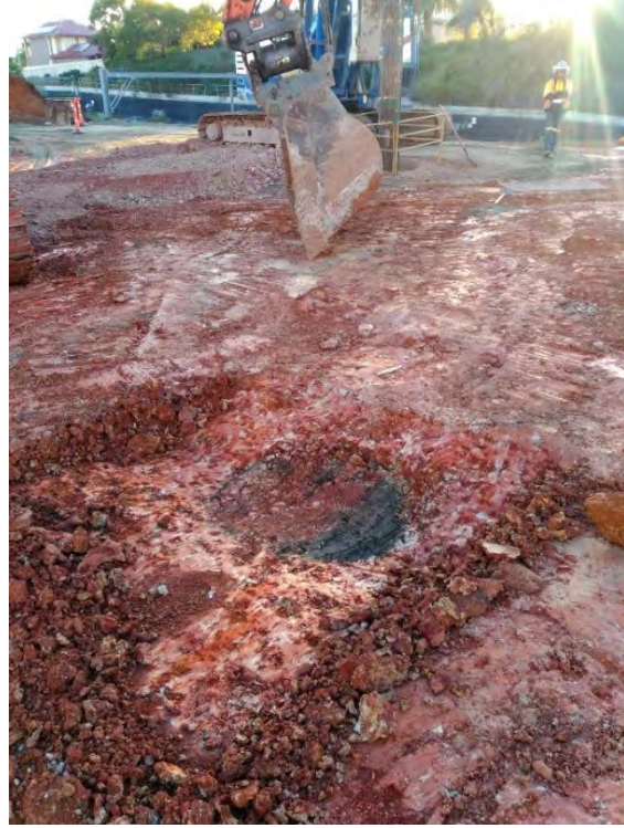
Figure 5.19 Detail of the base of the second well.
