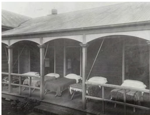
Figure 3.23 Early building re-used for dormitories identified as the 'Masters cottage' by Picture Willoughby, date unknown (Source: Picture Willoughby, File No: 6536/6536532).
