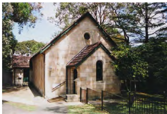
Figure 3.14 Holy Trinity Anglican Church, Chatswood West, 2003 (Source: Picture Willoughby, File No: 001/001101).
