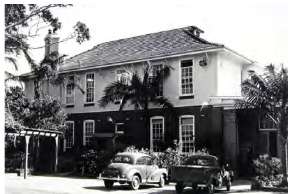
Figure 3.18 1950s view of Mowbray House School after purchase by Sydney County Council (Source: Picture Willoughby, File No: 003/003321).
