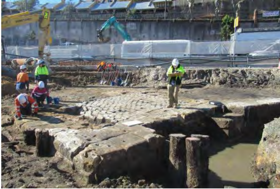
Fig. 17: View of the excavated area showing (i) the paved area at the end of Clyde Street terminating on the former foreshore of Darling Harbour and (ii) stone steps leading down onto the waterfront on the RHS of the photo (from Casey & Lowe 2019)
