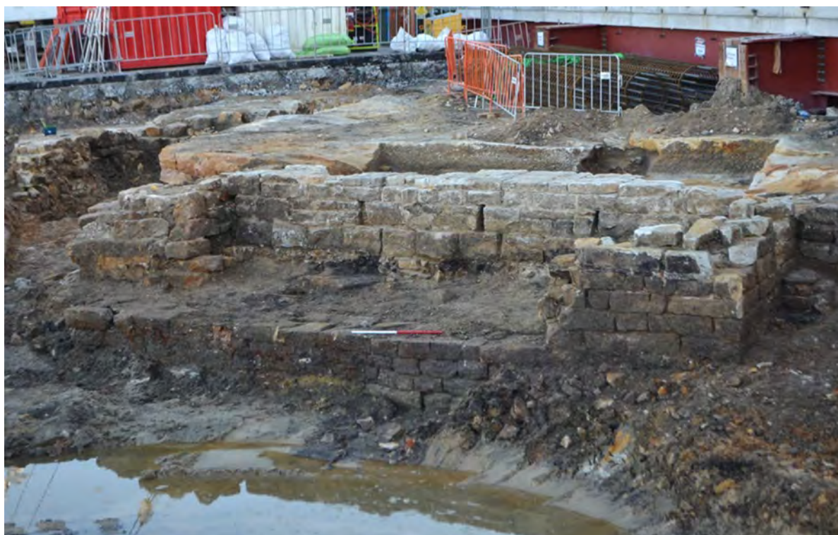
Figure 3.6: Sandstone foundations of Langford's House (1830s-1880s) at Barangaroo, Sydney. View to north, 1m scale. DSC_2585.
