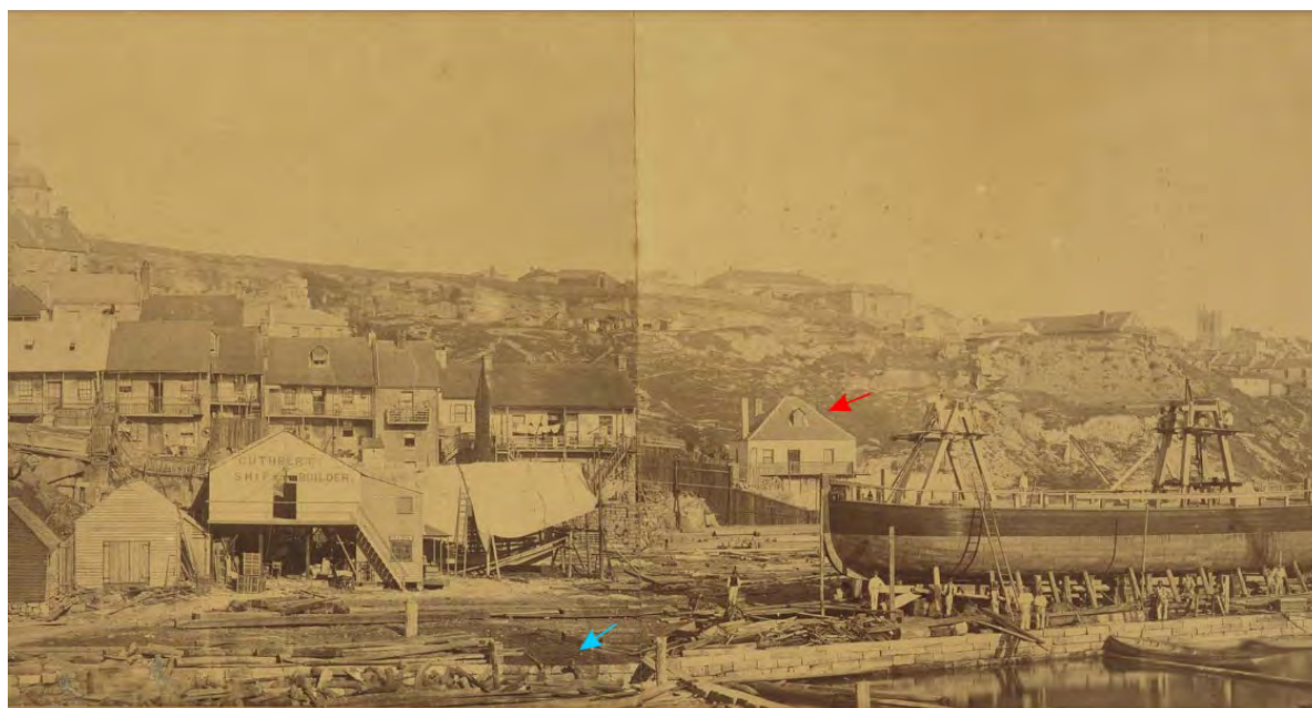
Figure 3.9: Cuthbert's Ship Build Yard Sydney, New South Wales by the Freeman Brothers. Photograph was taken looking to the east c.1870. It shows in great detail the large amount of ship building materials present on the wharf surface, including timber knees, marked with a blue arrow. The red arrow marks Langford's House. Held by the Australian Maritime Museum, Object no. 00028442.
