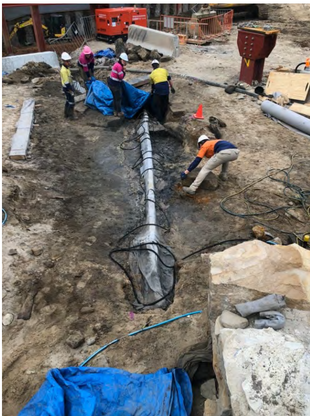
Figure 2.59: Installing soaker hose and covering wreck, in last stages of recovery.
