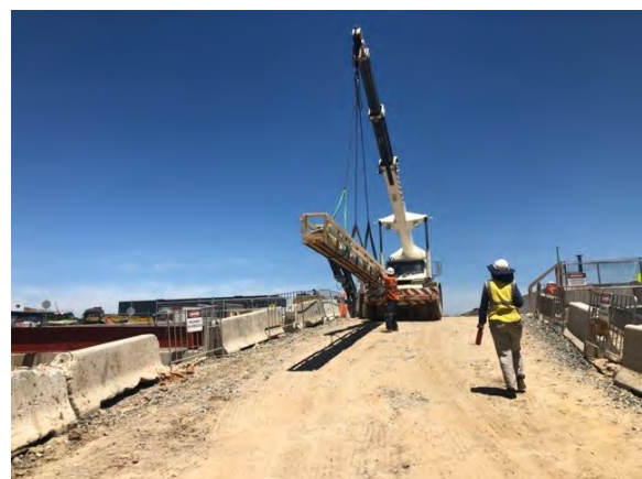
Figure 2.127: Crane lift of keel. (Source: Cosmos Archaeology).
