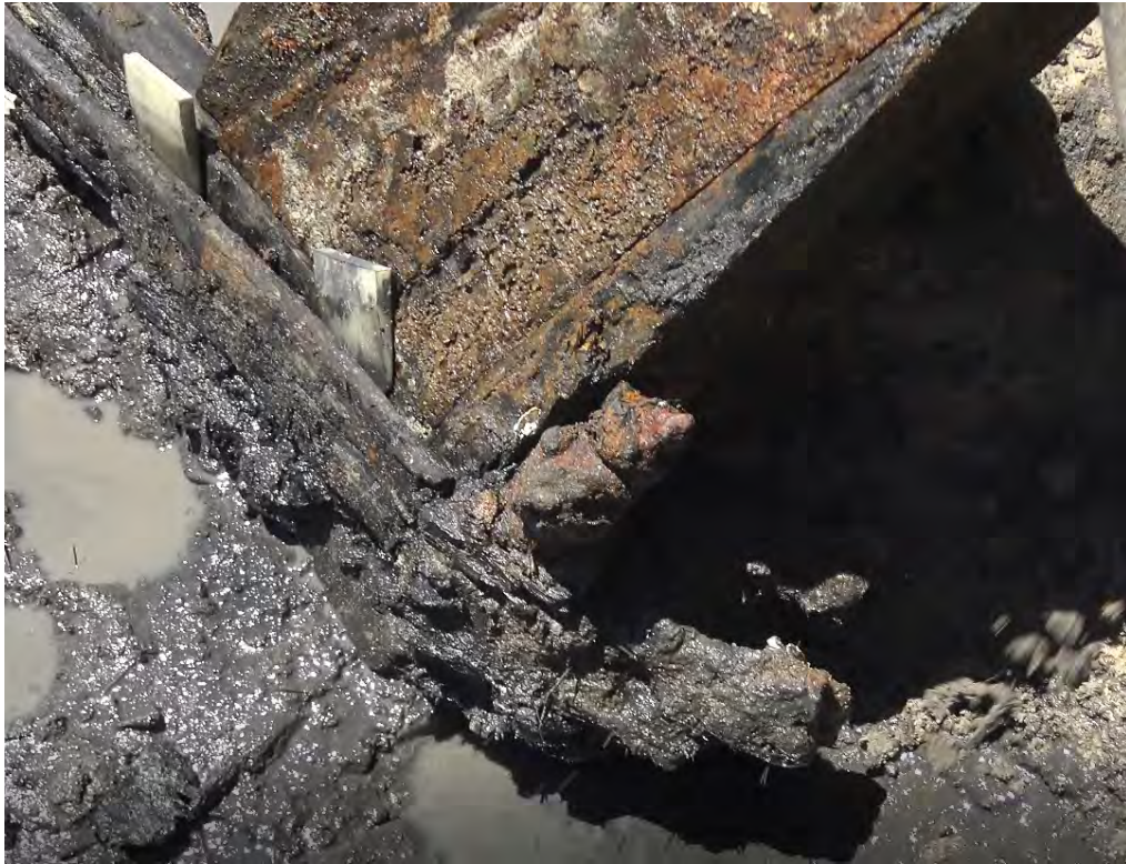
Figure 4.33: Gudgeon and pintle prior to removal. (Source: Casey & Lowe Recovery Video still, #150, 2018, 0:00:07).
