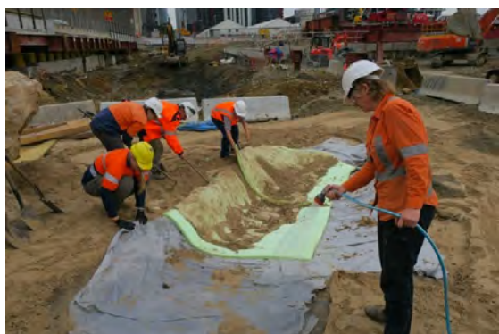
Figure 2.66: Removal of polyurethane foam and wetting geotextile.
