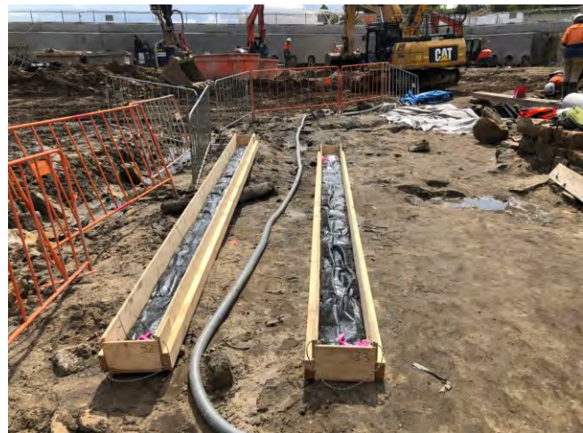
Figure 2.25: Ceiling planks inside their crates. Note the nylon rope lifting handles.
