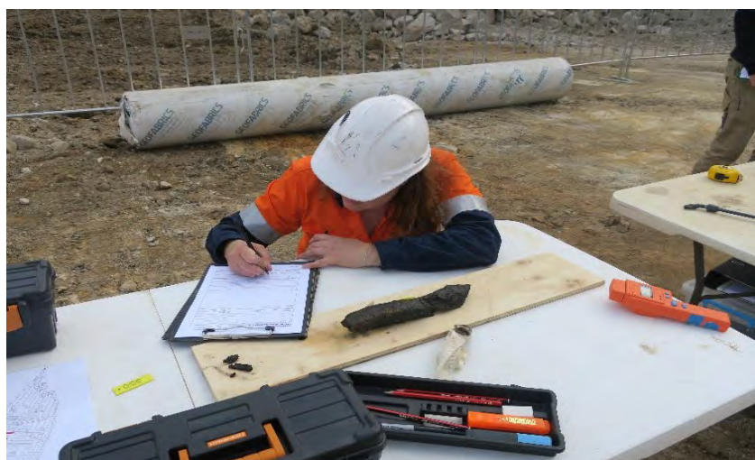
Figure 2.81: Surface moisture measurement station.
