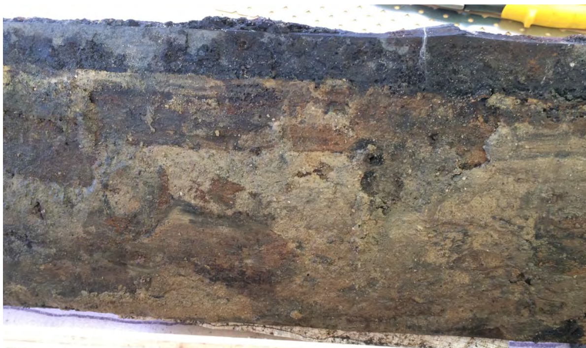
Figure 4.123: White putty between planking layers on outside of inner plank [313 S-I-S2-A]. (Source: AMBS).
