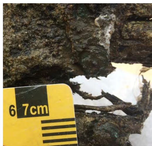
Figure 4.74: Head of copper fastener in situ. Aft-end of plank [464, SO-S09-A]. (Source: AMBS).
