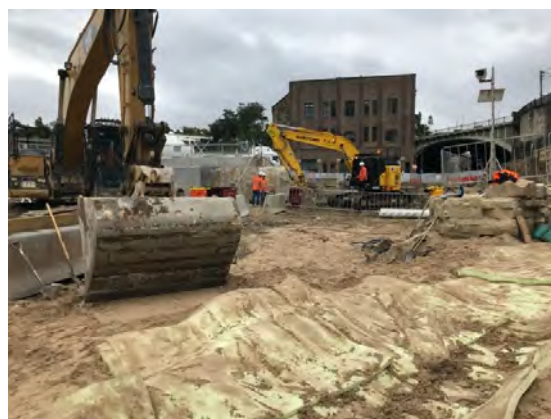
Figure 2.65: Removal of associated spoil by machine.
