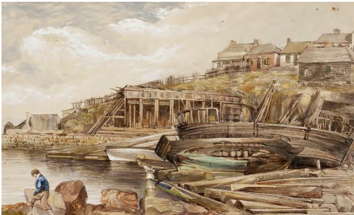
Figure 1.9: View of abandoned boats Cuthbert boatyard sometime in the 1860s, early 1870s. UDHB1 is located behind the artists position and was almost completely buried by this time.
