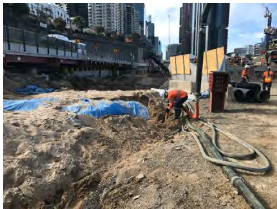
Figure 2.62: Removal of sand by vacuum truck.
