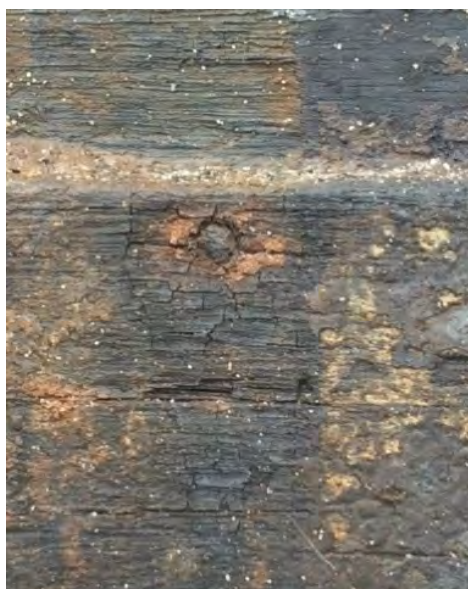
Figure 4.71: Ferrous \frac{1}{4} " framing nail in situ on plank [375 S-I-S11-M]. (Source: AMBS).
