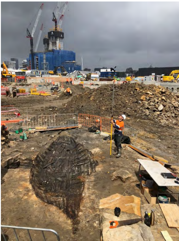
Figure 2.5: Photography with camera mounted on pole.
