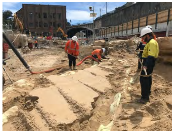
Figure 2.63: Removal of sand by vacuum truck.
