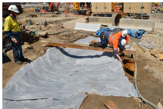
Figure 2.38: Final layers of geotextile. (Source: ICS).
