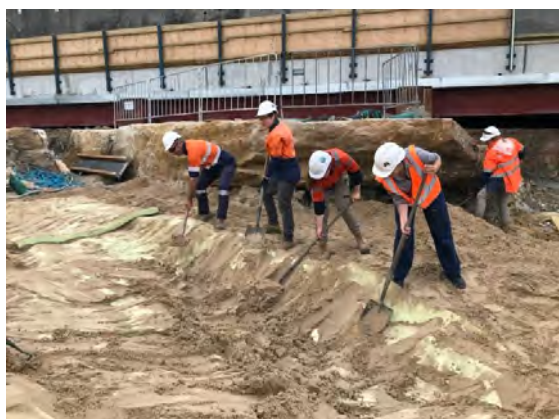
Figure 2.64: Removal of sand by shovel.
