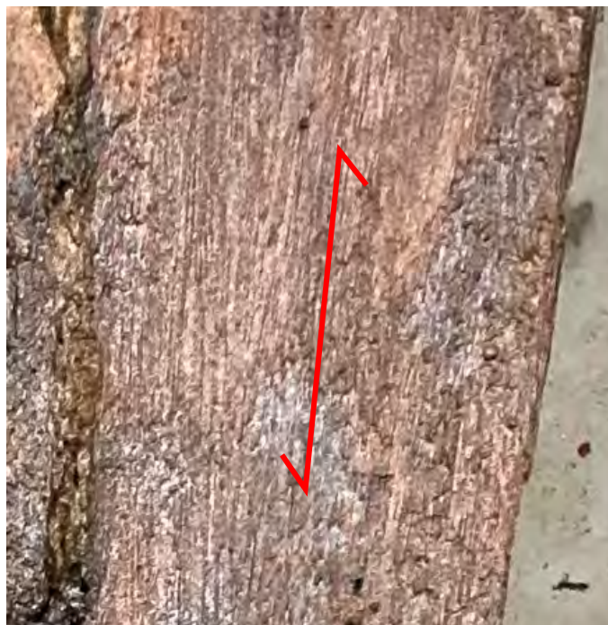
Figure 4.23: Sternpost grain orientation, port side. Aft edge on the right. Grain direction shown in red. (Source: Benjamin Wharton 2020).
