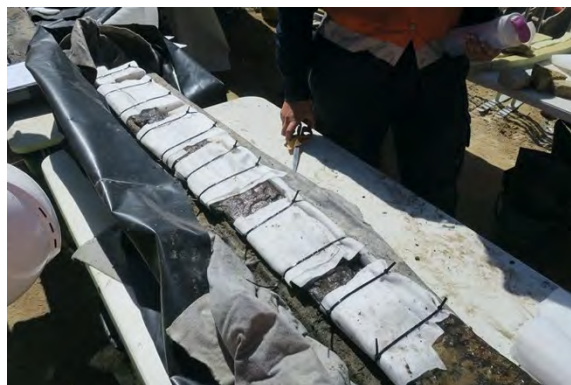
Figure 2.113: Bandaging split element. (Source: Casey & Lowe).
