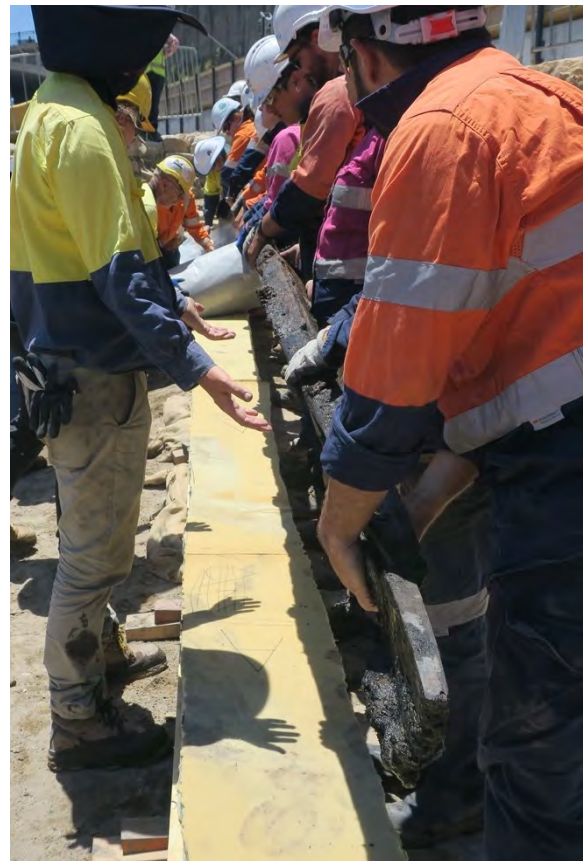
Figure 2.99: Removal of the keel.
