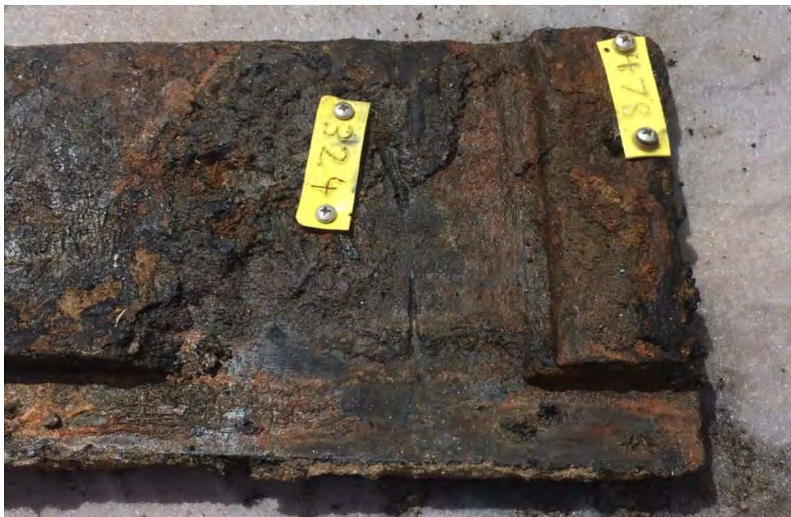
Figure 4.49: Scarf plate [478] in situ on plank [324 P-I-S3-A]. Note the length of scarf plate ends at land of overlapping plank. (Source: Casey & Lowe).
