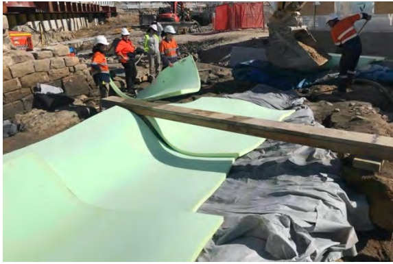
Figure 2.39: Installing polyurethane foam. (Source: ICS).
