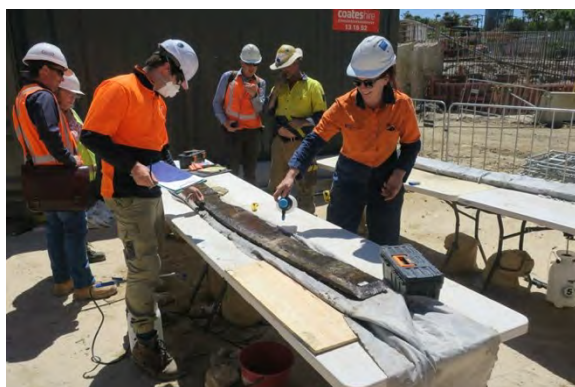
Figure 2.101: Keeping elements wet. (Source: Casey & Lowe).
