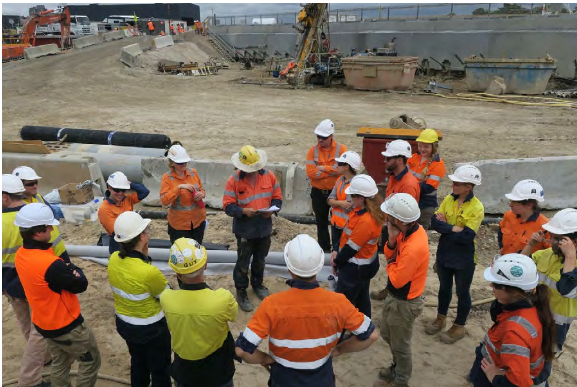
Figure 2.47 : Daily disassembly project pre-start.
