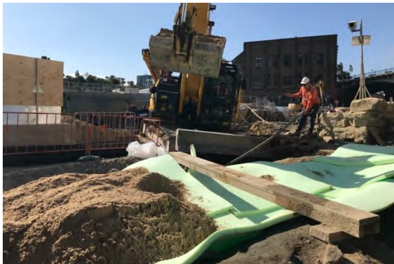
Figure 2.41: Covering with sand. (Source: ICS).
