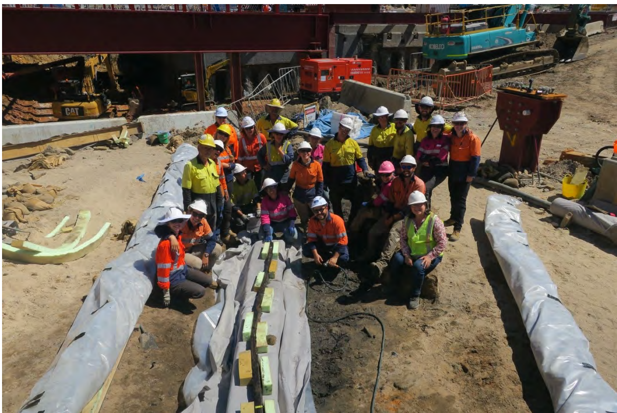
Figure 2.100: Removal of the last element. (Source: Casey & Lowe).
