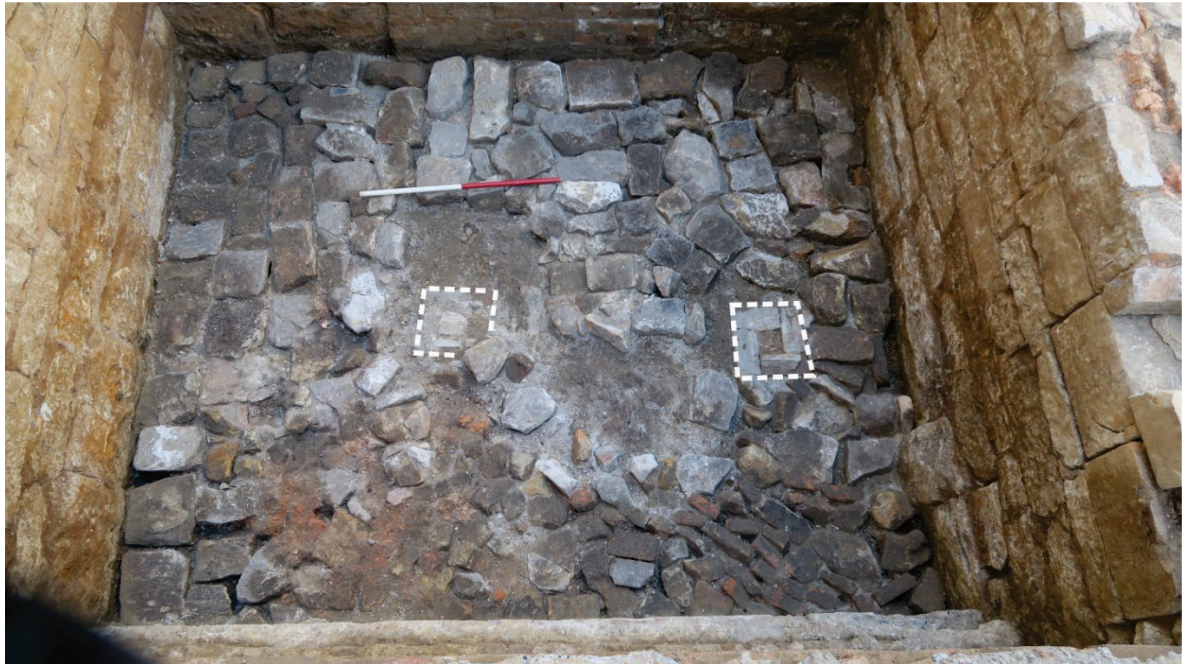
Figure 5.82: The sandstone paved floor of Cellar 2 with the later added dry-pressed brick piers (1066) outlined in white. View to the east. Scale 1m. IMG_9208.
