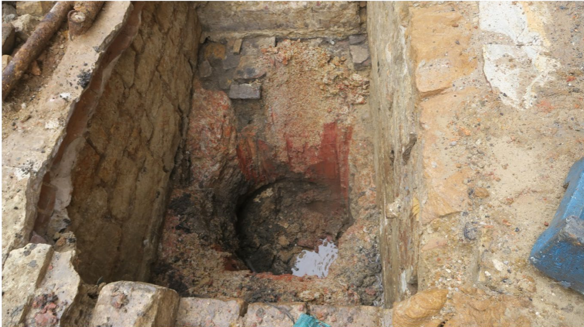
Figure 5.10: Due to ‘working at height’ restrictions the well was dug with the use of a 14-tonne excavator. Artefacts were retrieved from the fill removed by the machine. View to the west, 1m scale. IMG_9404.
