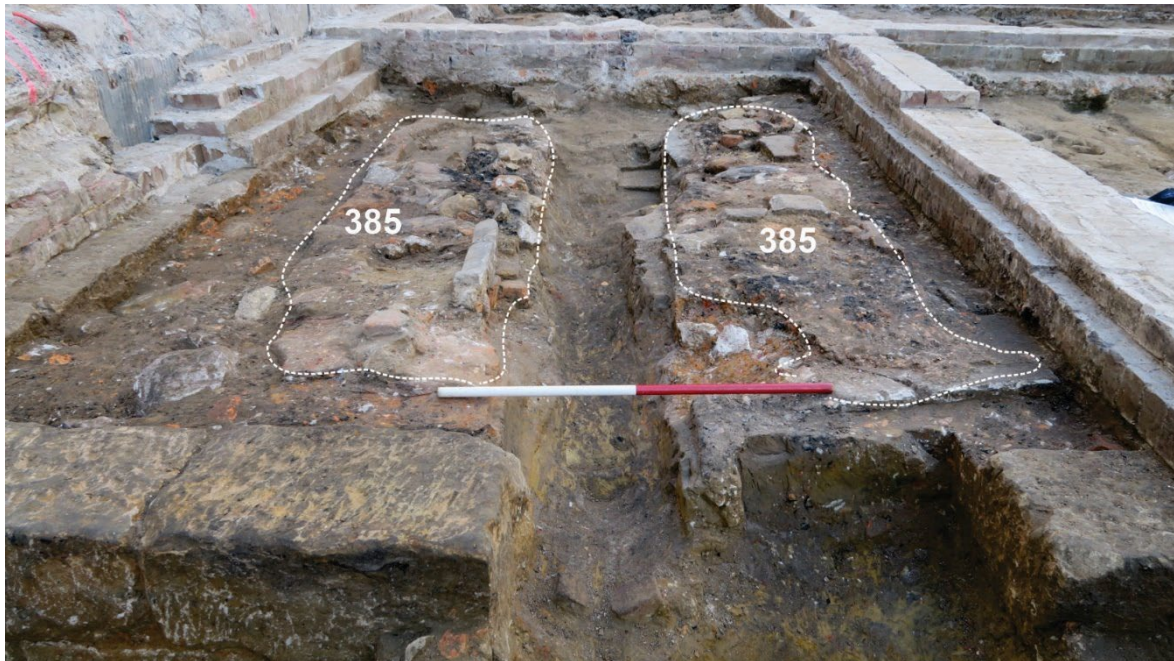
Figure 5.25: Building 6 Flooring (385) divided into two main patches by a later service cut (222). View to the east. Scale 1m. IMG_7835.
