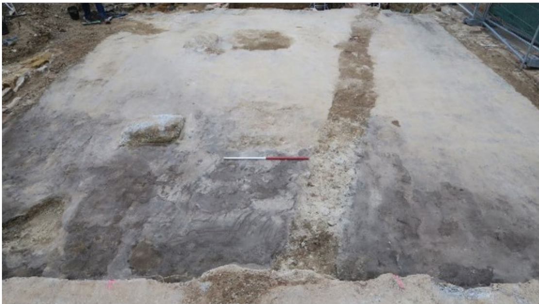
Figure 5.100: Cyclopean concrete floor of the 1909 theatre sloping down from Pitt Street towards the stage in the east (left). View to the west, 1m scale. IMG_9079.
