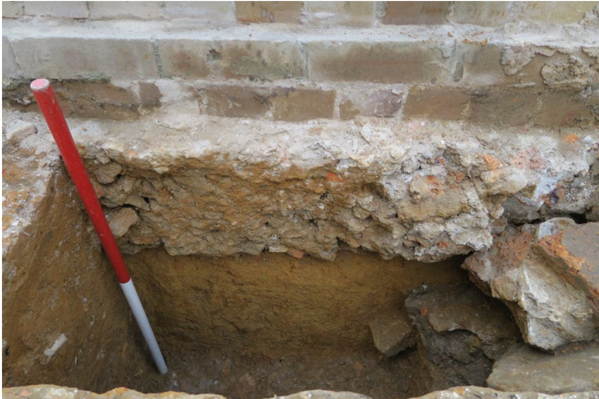
Figure 5.111: East facing section of service trench C115 revealing concrete and DP brick wall footing C015. View to the west. Scale 1m. IMG_7304.[Insert caption]
