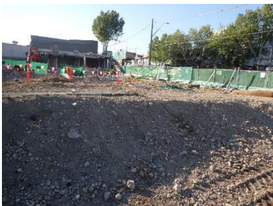
Figure 3.16 View south from Hume Street of overburden deposits pre-excavation.
