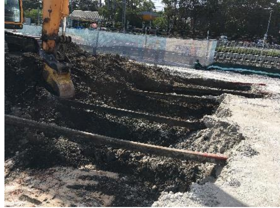
Figure 5.13 Track exposed during excavations, functioning as reinforcement.
