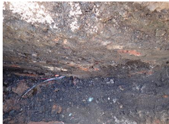
Figure 5.11 Tip lines visible in the section of TP19 as well as a buried electrical service.
