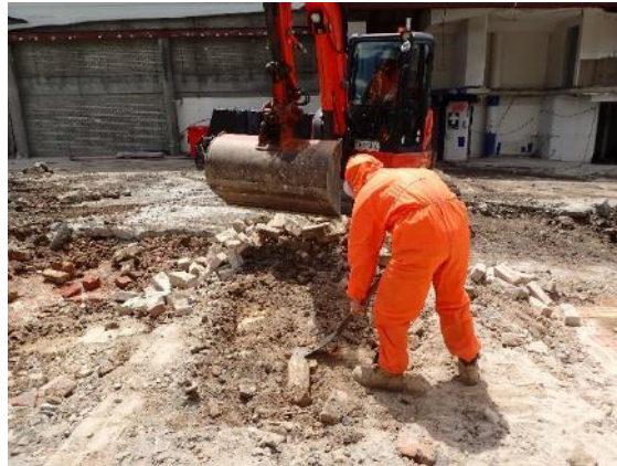
Figure 3.7 Machine and hand excavation of overburden in progress (7 December 2017).
