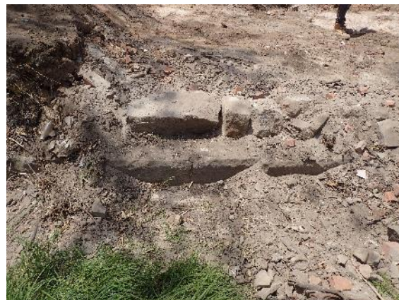
Figure 4.6 Terrace wall of re-used sandstone blocks adjacent to the eastern boundary of the Victoria Cross site.
