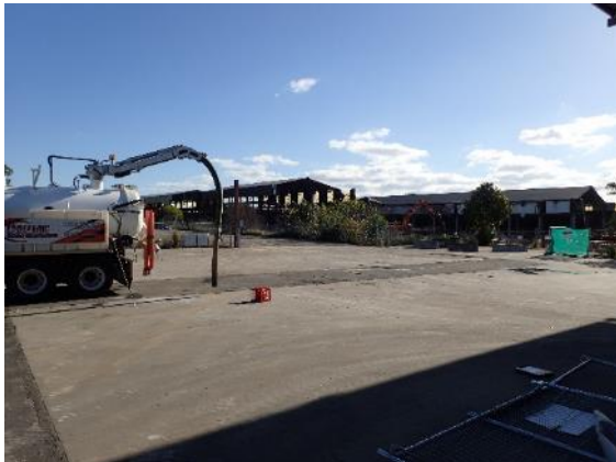
Figure 5.4 View south-west of the sucker truck undertaking the 'non-destructive' borehole investigations.
