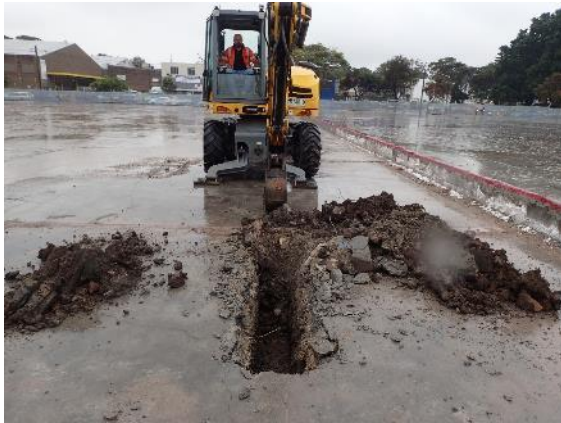
Figure 5.6 View south-west and excavation of TP12.
