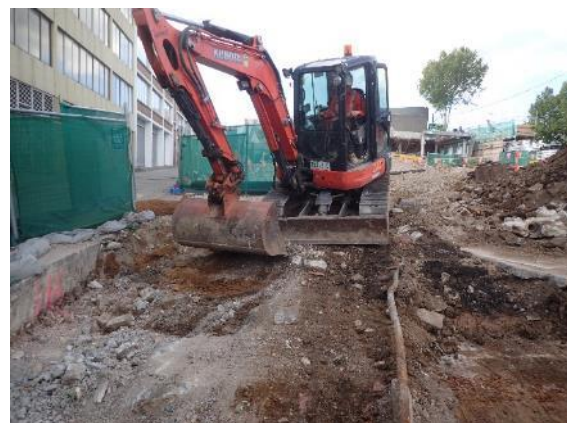
Figure 3.17 View south-east of machine excavation of contaminated deposits overlying B Horizon.
