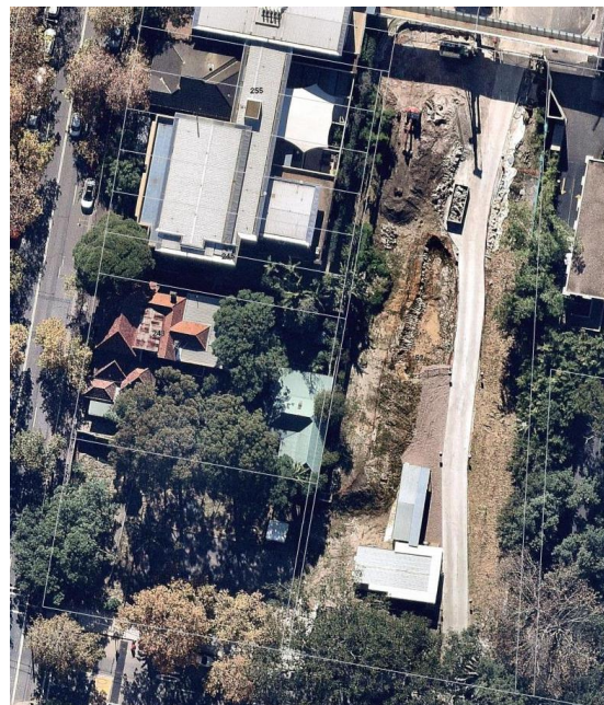
Figure 4.10 6 May 2017. The haul road was built for construction on the adjacent property.
