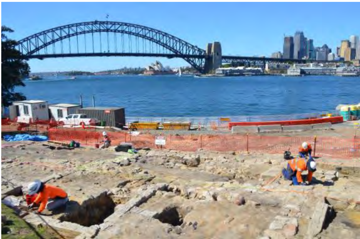
The view of the Sydney Harbour Bridge and Opera House from the former industrial waterfront of Blues Point. The foundation walls in the foreground include those of the houses built by in 1869 (image supplied by Dr. Mary Casey)
