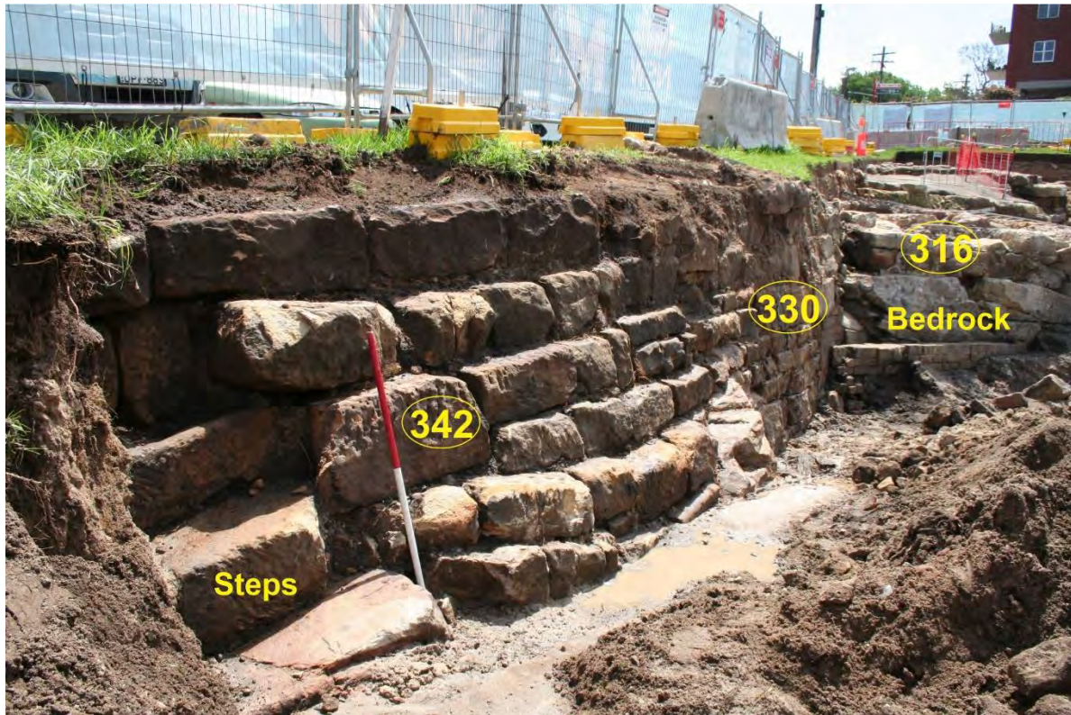
Figure 4.88: Different phases of north-south seawall and retaining wall (342 and 330) along the western edge of the site with steps in the foreground. View northwest, scale 1m. IMG_5603.
