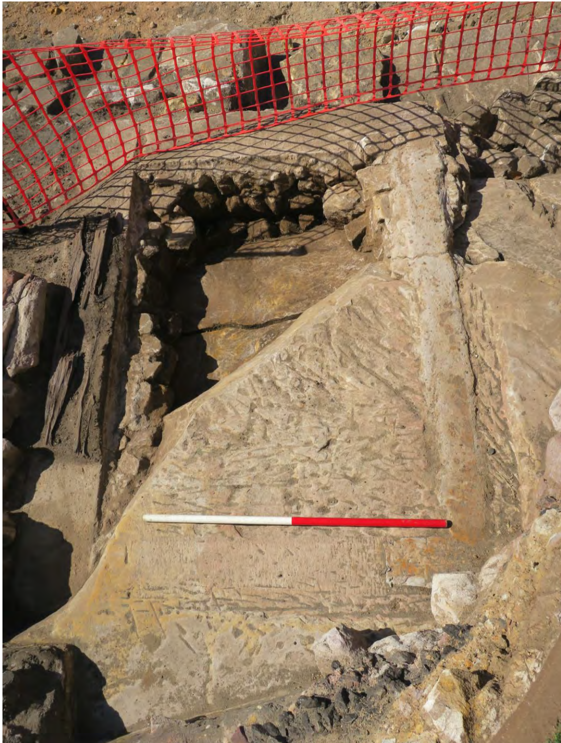
Figure 4.98: Base of weighbridge (322) cut into the bedrock with a concrete and timber frame. South retaining wall in the background (behind the safety fence). View to east, scale 1m. IMG_1310.
