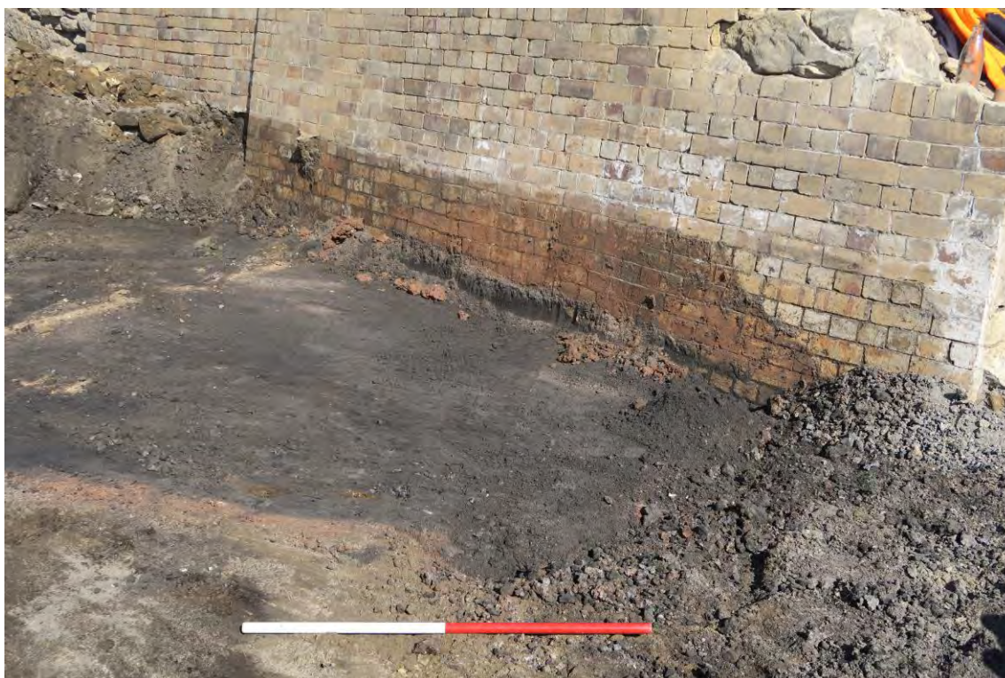
Figure 4.83: Machine excavation exposed more fills abutting the brick portion (321) of the south retaining wall. View to northwest, scale 1m. IMG_0057.
