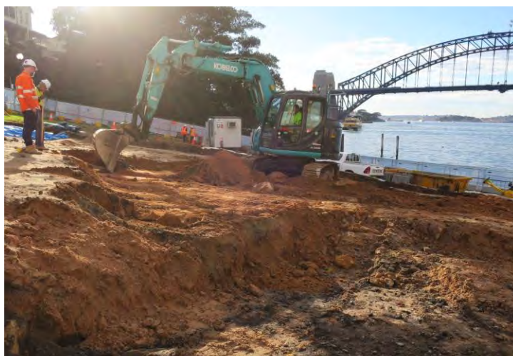
Figure 4.125: Excavation of the 20th-century bulk fills within the study area.
