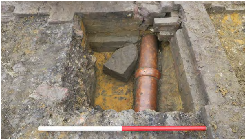
Figure 4.111: East-west service pipe (012) cutting through the brick footings of Room A, House 2 and into the bedrock, within TT 03. View to west, scale 1m. IMG_9504.
