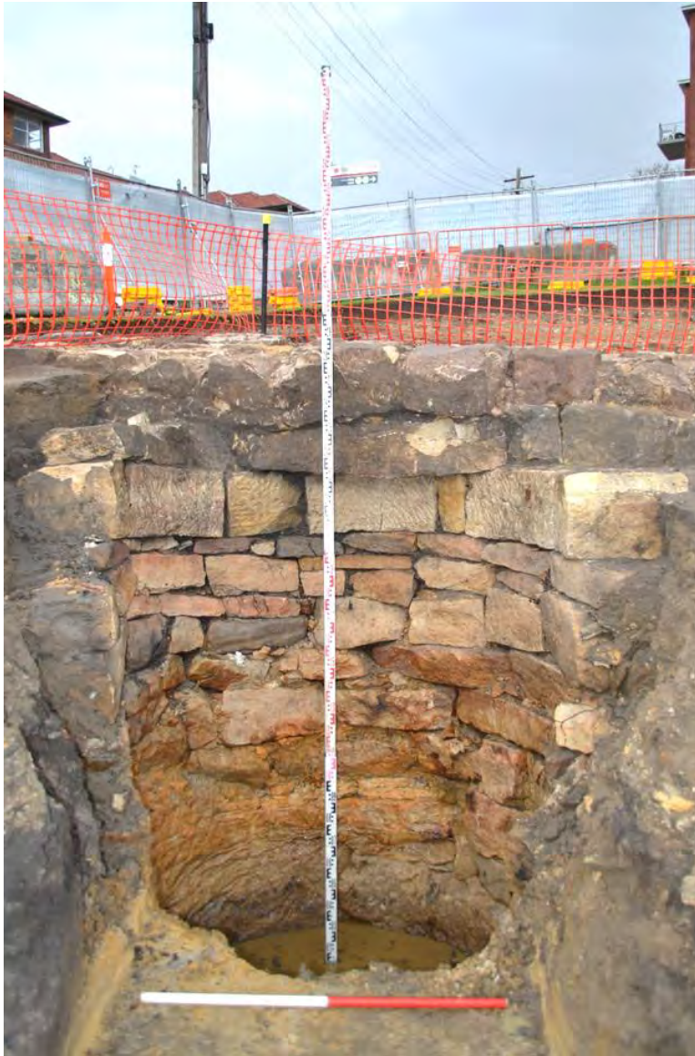
Figure 4.39: Machine excavated trench through cistern (087) cut deep into the bedrock. Note how the two courses of the verandah wall slightly overhang the cistern. View to north, scale 1m and 4m. DSC_4897.
