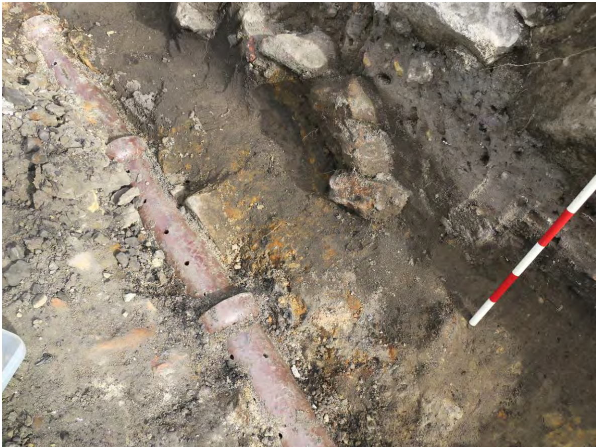
Figure 4.113: Segment of pipe with holes (327) running along the access road below the north retaining wall. Scale 500mm. IMG_1366.
