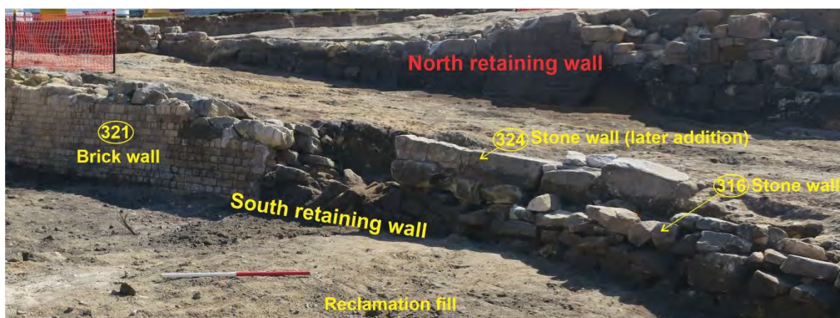
Figure 4.81: Detail of the eastern end of the south retaining wall (316) including the later modifications (321 and 324). View to northwest, scale 1m. IMG_1306.
