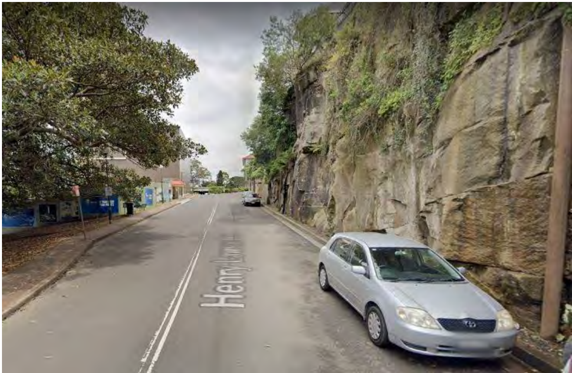
Figure 4.14: View west along Henry Lawson Avenue showing the vertical quarried rockface to the north of the road with the study area to the south, behind the blue hoarding. Google Street View April 2021.
