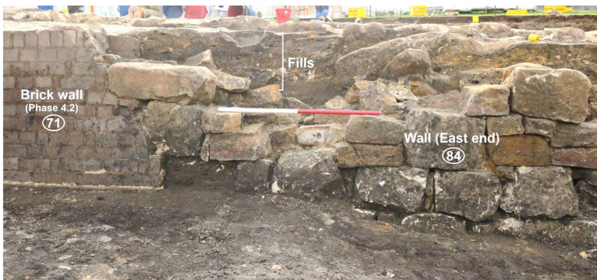
Figure 4.49: Eastern end of north retaining wall (084) with later brick wall repair (071). Behind the wall were layers of fill (collectively recorded as context 067) to raise the ground for the construction of House 2 and 3. View to north, scale 1m. IMG_1257.
