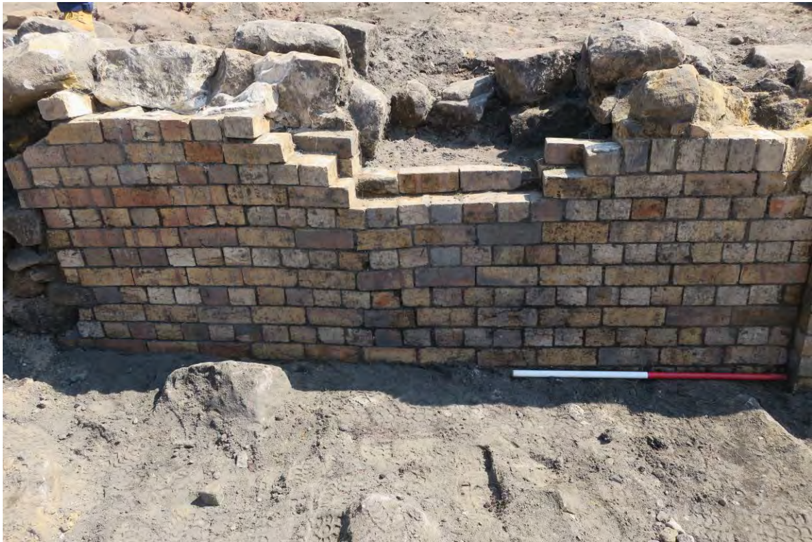
Figure 4.82: Portion of south retaining wall replaced with a later brick wall (321). View to north, scale 1m. IMG_1281.
