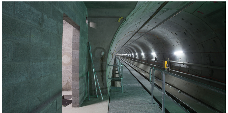
Example of a completed cross passage.
