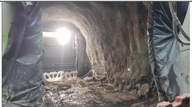
TBM Marlene Tunnel: Cross passage excavated.
