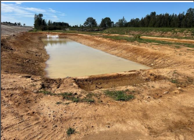
Cosgroves Creek – The sediment basin has been constructed as per ESCPs however requires a spillway
