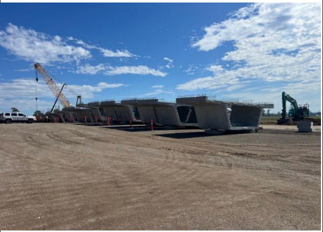
Luddenham South - Segments have been stacked to accurately facilitate the sequence and access by the crane
