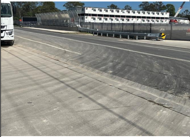
Lansdowne Road - Minor mounts of dirt have been tracked out of the site, however a street sweeper has been stationed there to clean the road
