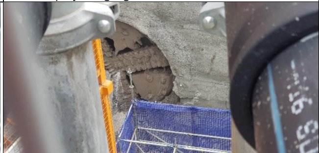
Claremont Meadows: TBM Catherine breakthrough.
