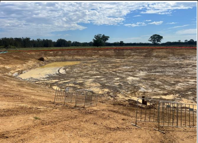
Cosgroves Creek – Work continues on excavating the 30ML flood retention basin
