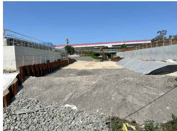
Figure 2.10: Rosehill Site – GSW and ASS stockpiles not segregated
