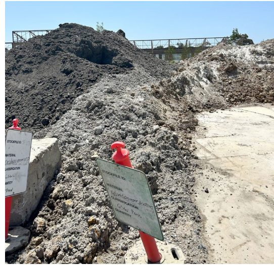
Figure 2.10: Rosehill Site – GSW and ASS stockpiles not segregated
