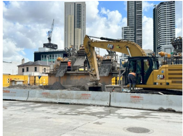
Figure 2.4: Parramatta site – Bentonite Plant de-sander material stockpile
