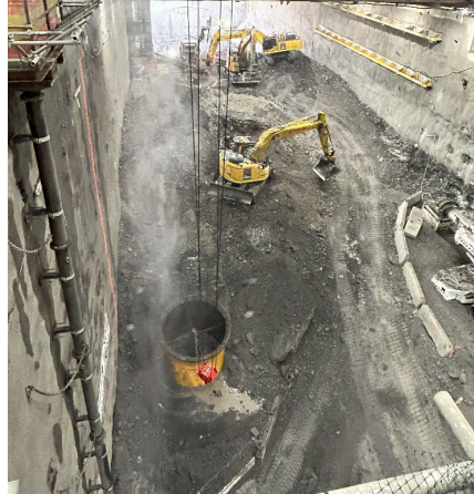
Figure 2.2: Westmead site – Station Box excavation inside acoustic shed
