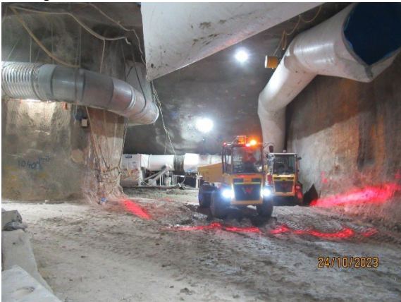
Figure 3.5 Hunter East: Road header excavation of the cavern ongoing
