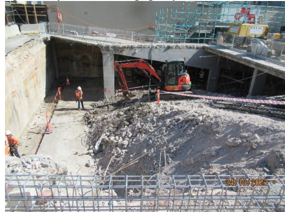
Figure 3.4 Pyrmont West: Works to install wall support around former basement
