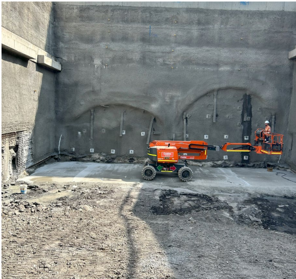
Figure 2.5: Clyde Dive site –Dive Structure excavation along the ATC boundary
