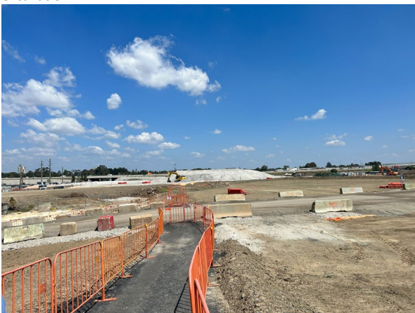
Figure 2.13: Clyde MSF Site – Parramatta Speedway backfilling
