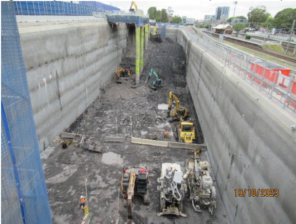
Figure 1.7 Excavation of spoil using steel platforms; wall support. (North Strathfield)
