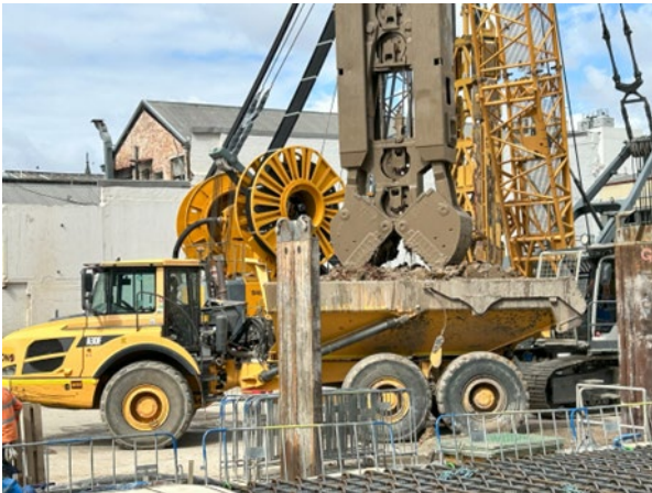
Figure 2.3: Parramatta Site – D-Wall excavation with grab loading Moxy
