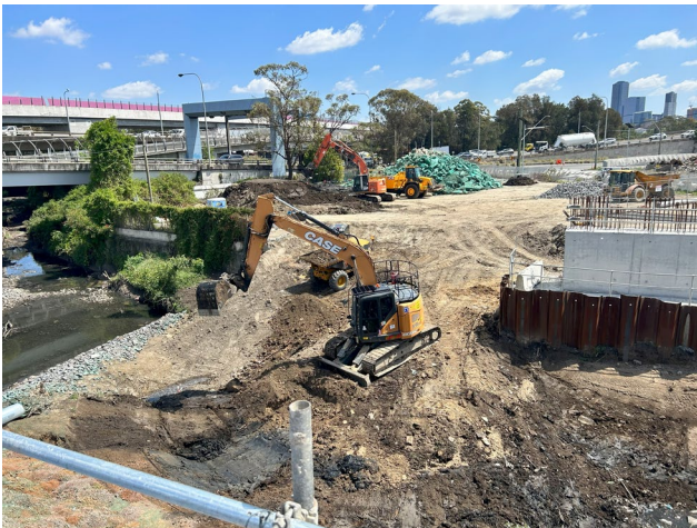
Figure 2.11: Clyde MSF Site – Duck Creek High Flow diversion excavation
