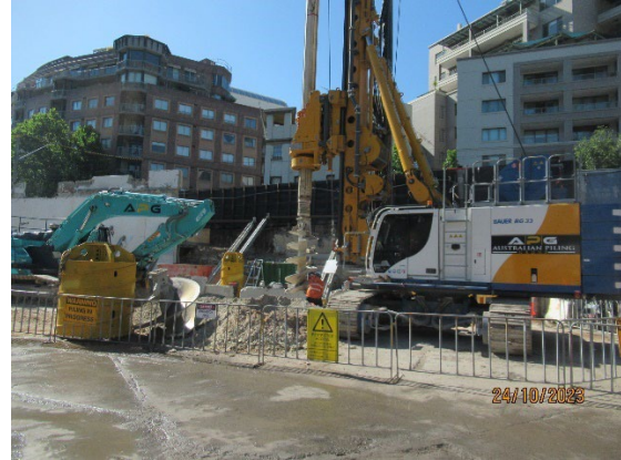
Figure 3.2 Pyrmont East: Piling rig in operation
