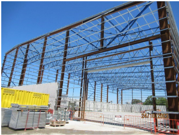
Figure 3.7 The Bays: Frame being constructed for the Spoil Shed
