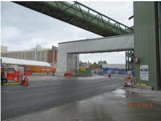
Figure 1 1 New pedestrian bridge over the Port Access Road (The Bays)
