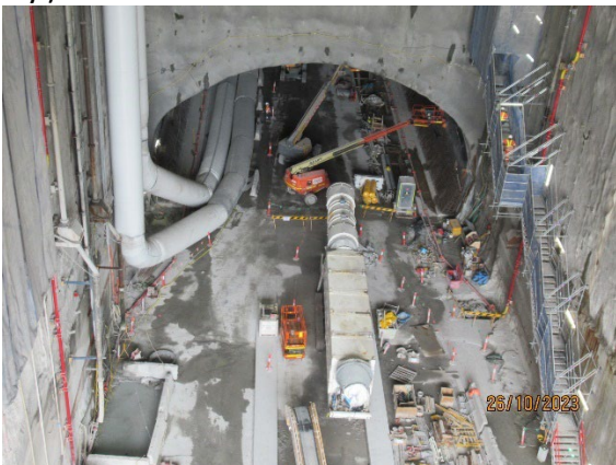
Figure 1 3 Cross Over Cavern: preparation for roof lining concrete pours (Burwood North).
