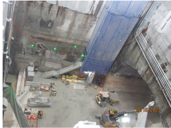
Figure 1 6 Works in the base of the East Shaft (Five Dock-east).
