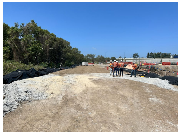
Figure 2.14: Clyde MSF Site – Utilities trench installation along Duck Creek
