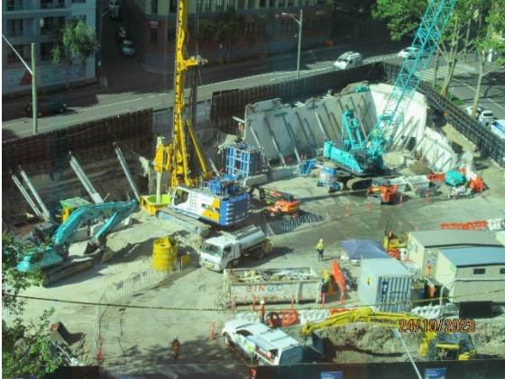
Figure 3.1 Pyrmont East: Commencement of piling works
