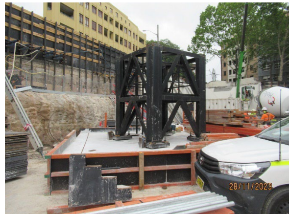
Figure 3.2 Pyrmont East: Tower Crane base and foundation
