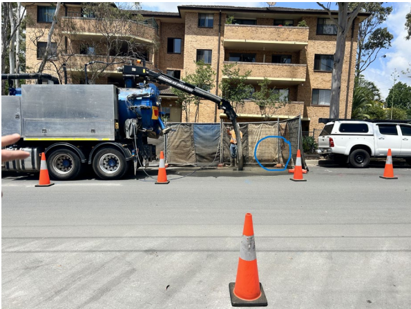
Figure 4.1 Westmead Utility Works: Utility investigations with Vac Truck
