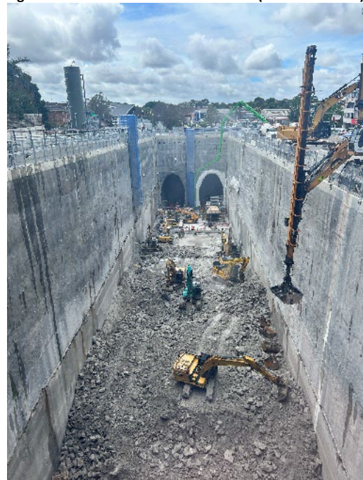
Figure 1 4 Station Box excavation and nozzle works. (Burwood North)
