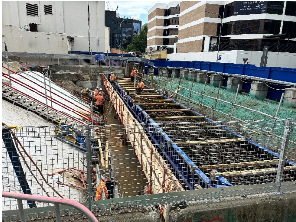
Figure 2.4: Parramatta site – Capping beam FRP works
