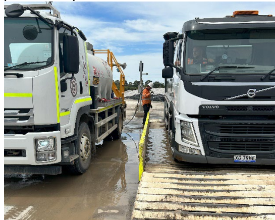
Figure 2.14: Clyde MSF Site – Gate 9 wheel wash with additional high pressure cleaning
