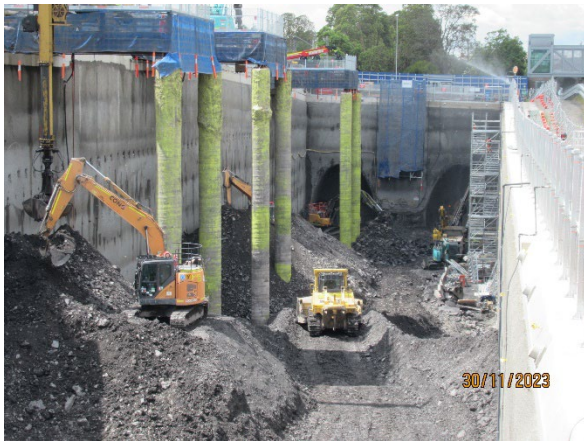
Figure 1.7 Excavation of spoil using steel platforms. (North Strathfield)
