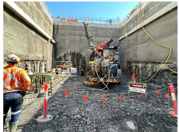
Figure 2.6: Clyde Dive site – Dive Structure excavation along the ATC boundary
