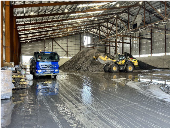
Figure 2.7: Rosehill Site – spoil shed in operation
