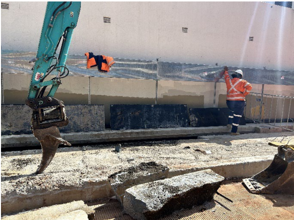
Figure 2.3: Parramatta Site – Guide wall removal adjacent to Roxy Theatre
