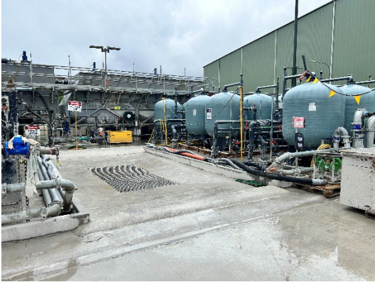
Figure 1 1 Water Treatment Plant (The Bays).
