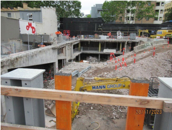
Figure 3.3 Pyrmont West: Works to install wall support around former basement
