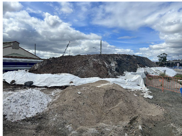
Figure 2.5: Clyde Dive site – ASS stockpile storage and treatment area
