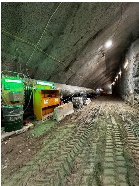
Figure 3.5 Hunter East: Road header excavation of the cavern ongoing
