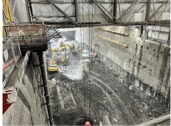
Figure 2.2: Westmead site – Station Box excavation inside acoustic shed with water sprays
