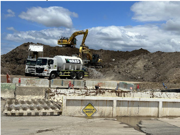
Figure 2.13: Clyde MSF Site – Spoil management and dust suppression
