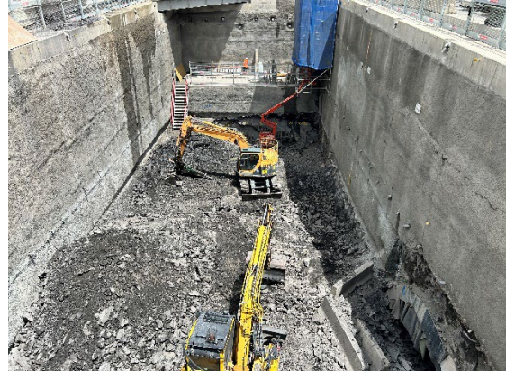
Figure 1 2 Excavation of the South Shaft (Burwood North).
