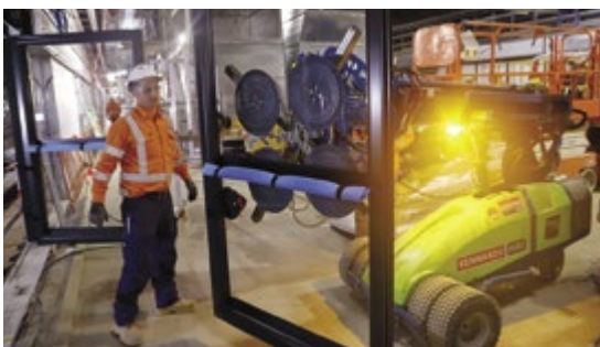
Image: Installing platform screen doors at Crows Nest Station.
