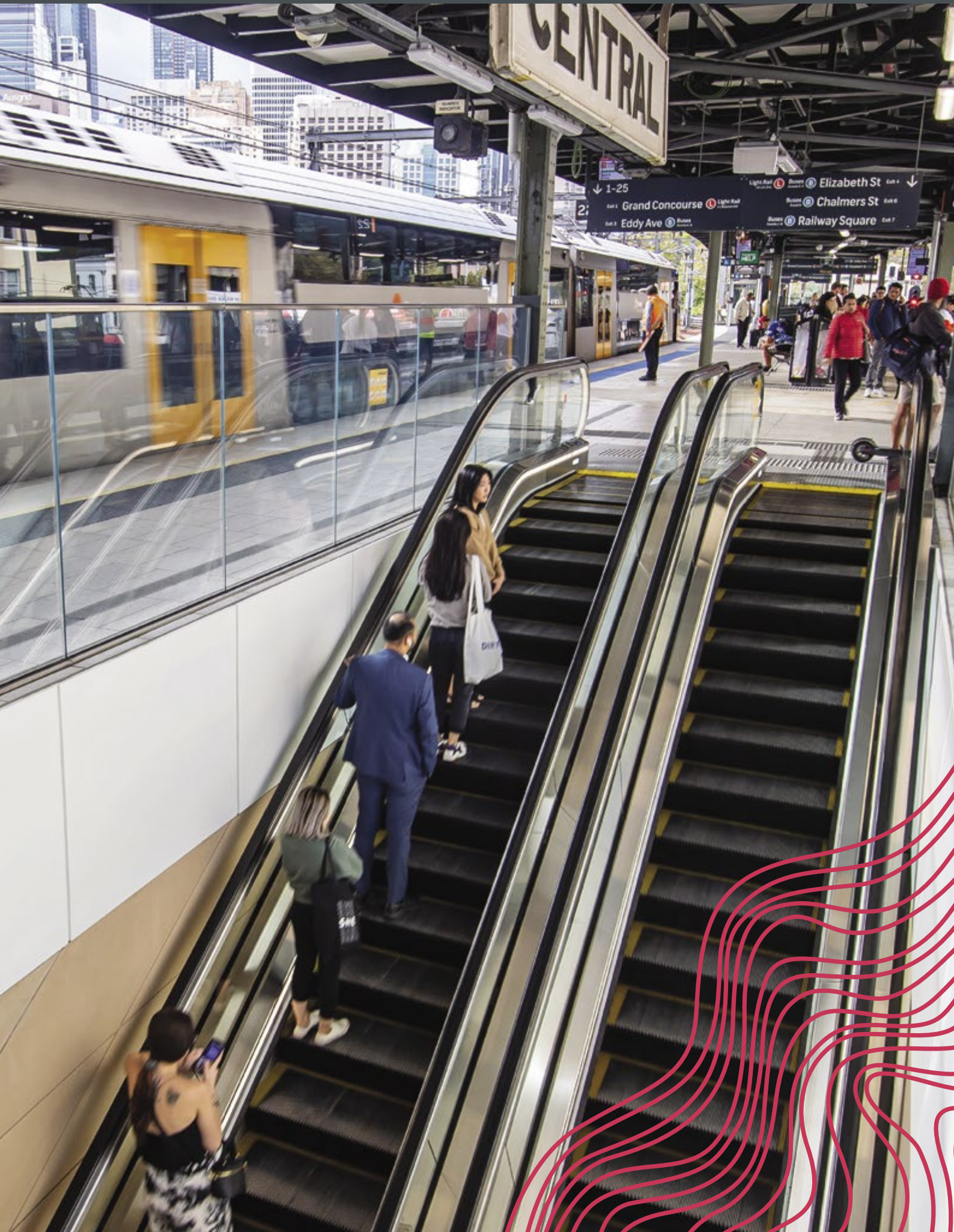
Image: In preparation for Metro services at Central Station escalators have been installed to provide convenient access to suburban platforms.
