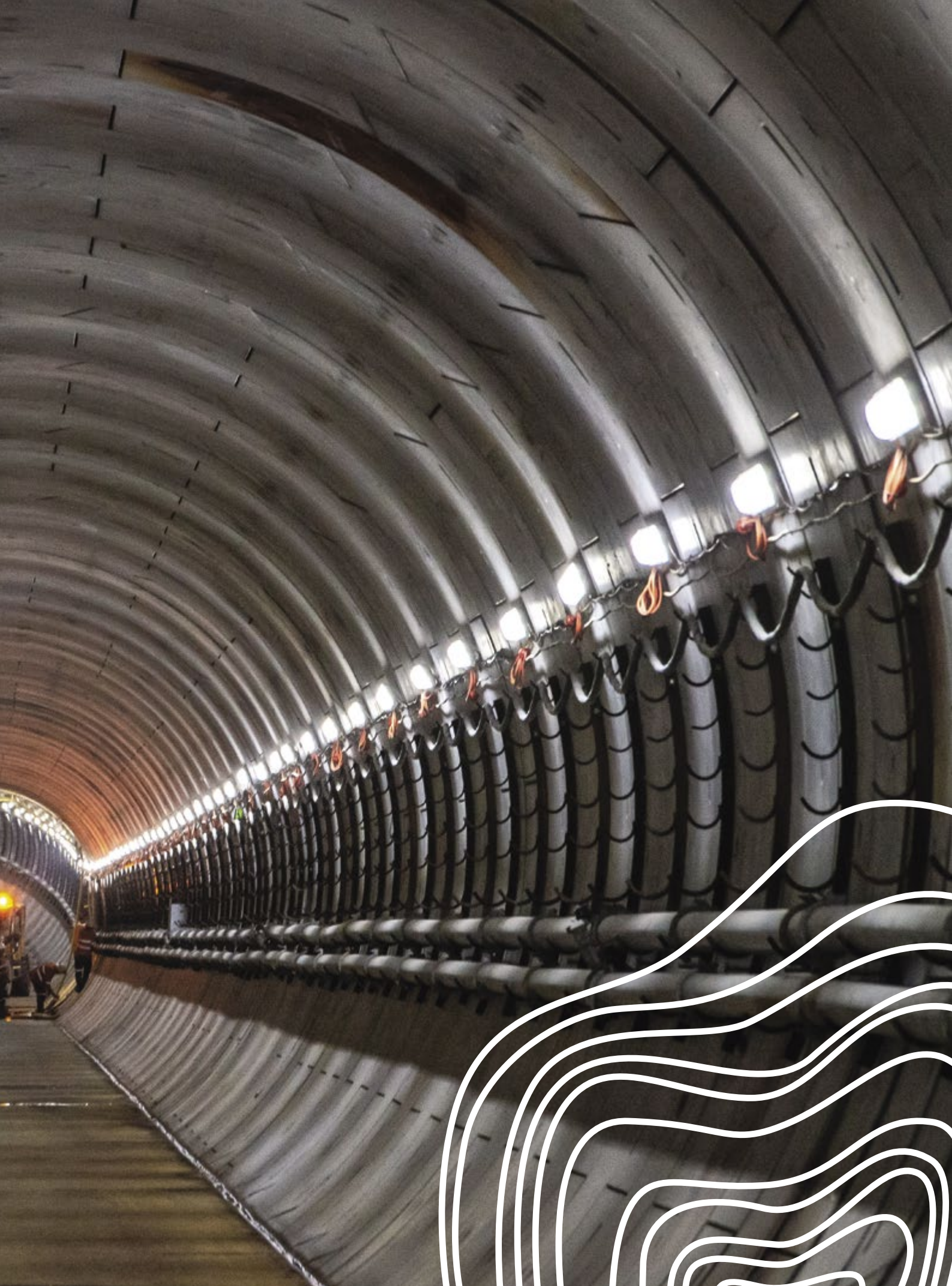
Image: Tunnel under Sydney Harbour.
