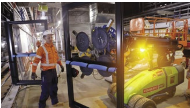
Image: Platform screen doors being installed at Crows Nest.
