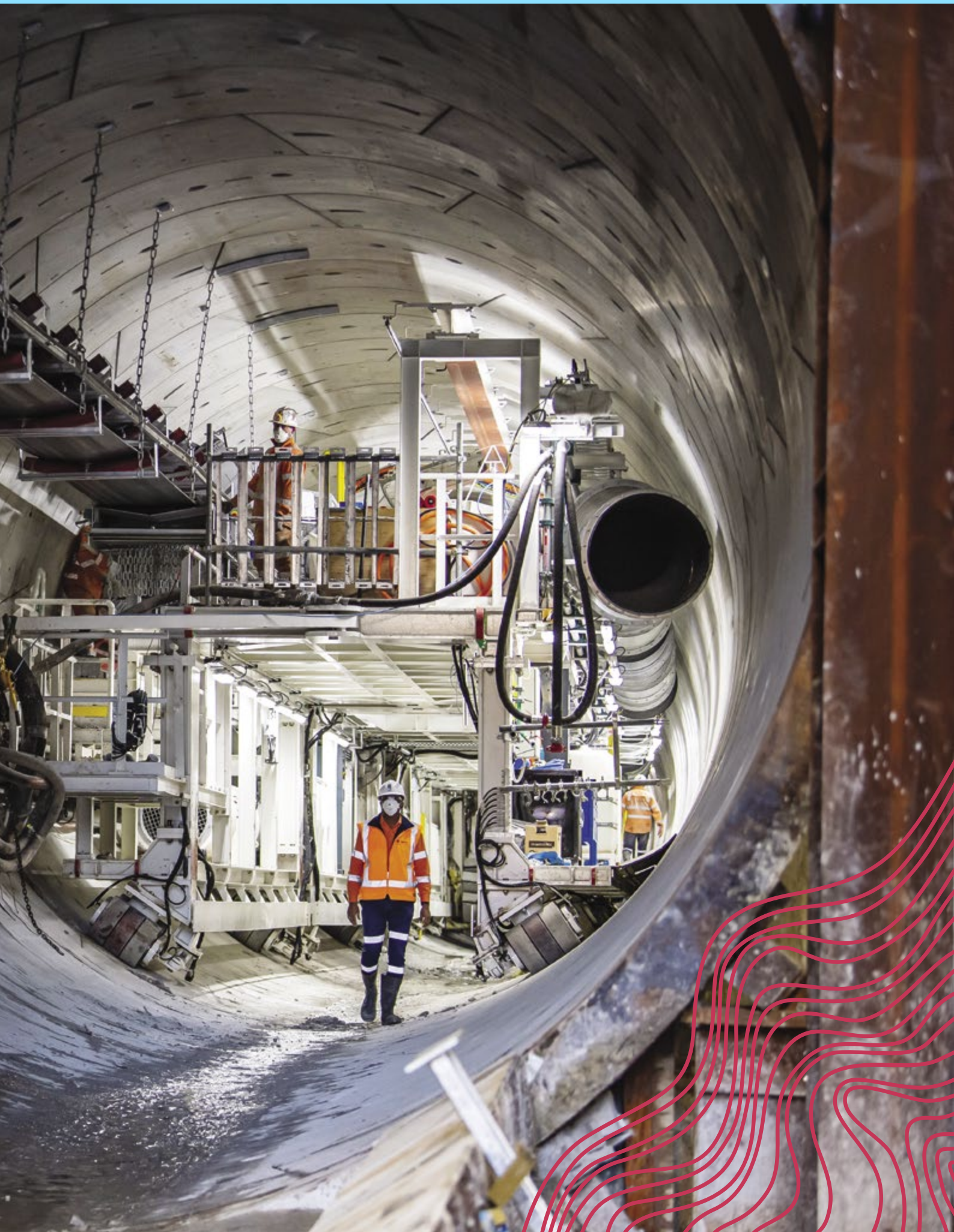
Image: Olympic Park construction.
