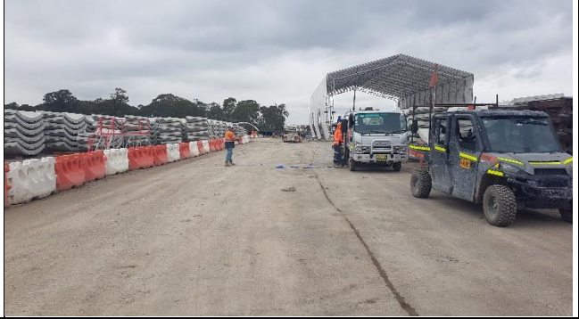
Orchard Hills view south: Improved condition of internal roads.
