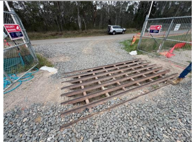
The entry exit point from the site compound is clean with no mud tracking.
