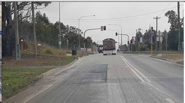
Kent Rd View north: Pothole at No. 57 repaired.
