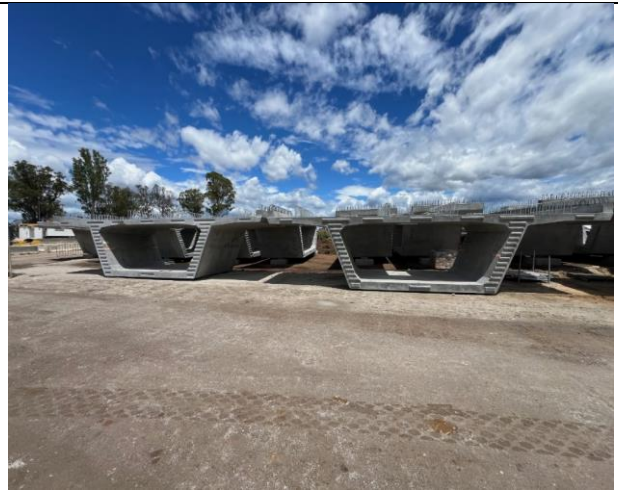
Luddenham South: Viaduct segments are stored in a specific order to be lifted into correct position.
