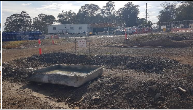
Claremont Meadows: Concrete washout area well implemented.
