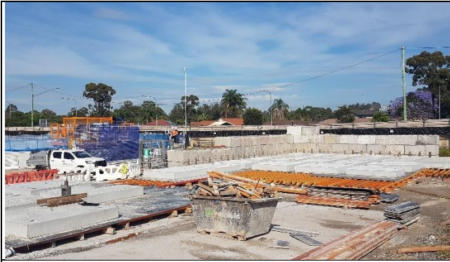
Claremont Meadows: Casting of TBM traverse support blocks.
