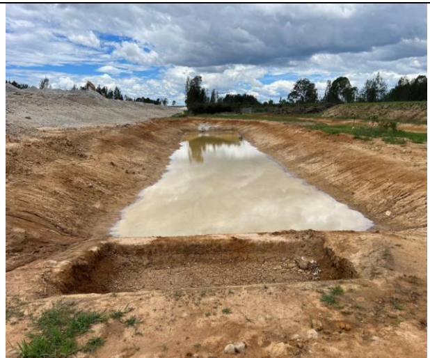
Cosgroves Creek: The downstream basin is operating well and capturing run off from the catchment.
