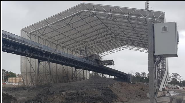
Orchard Hills view northwest: Consistency of TBM spoil material improved.
