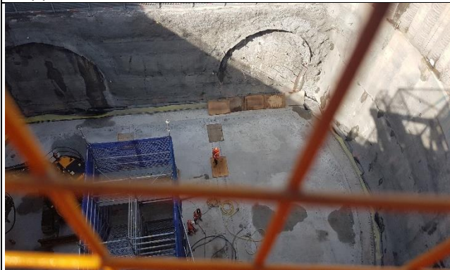
Claremont Meadows: Shaft base slab completed.
