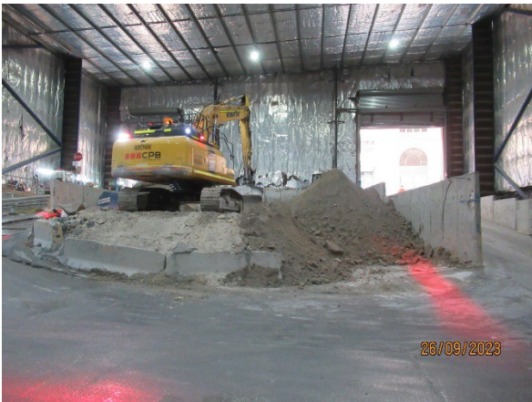
Figure 3.5 Bligh Street Acoustic Shed: Ongoing load out of spoil onto trucks
