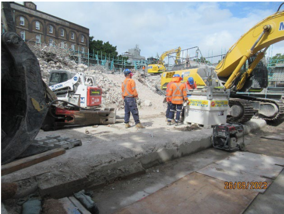
Figure 3.3 Pyrmont St West: Hard demolition near completed.
