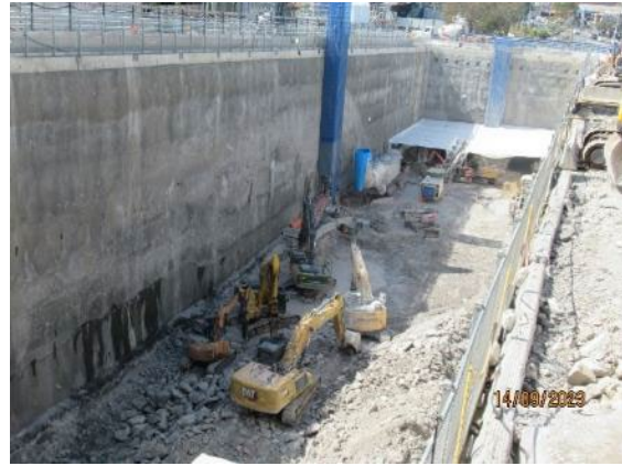
Figure 1.4 Station Box excavation and nozzle works. (Burwood North)
