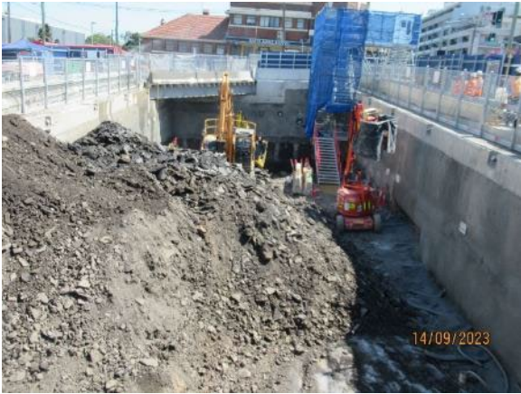
Figure 1.3 South shaft excavation ongoing, with wall support (Burwood North).
