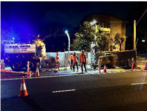
Figure 2.3: Westmead Site – Night drilling works on Alexandra Avenue
