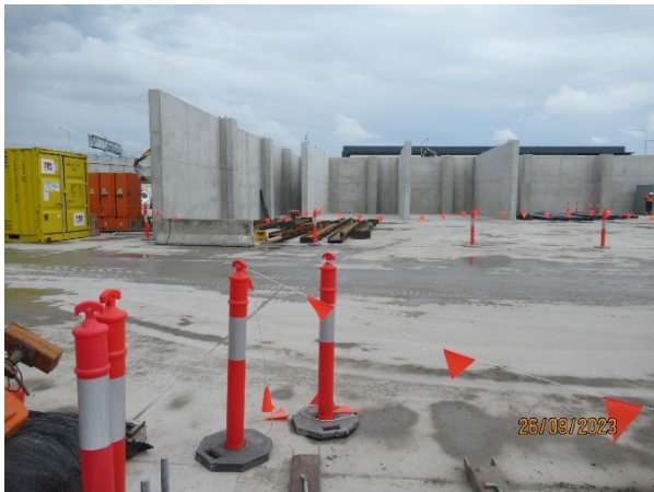
Figure 3.7 The Bays: FRP activities completed for the Spoil Shed
