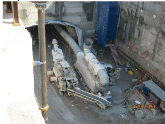
Figure 1.6 Ongoing excavation of the western cavern using road header (Five Dock-west).
