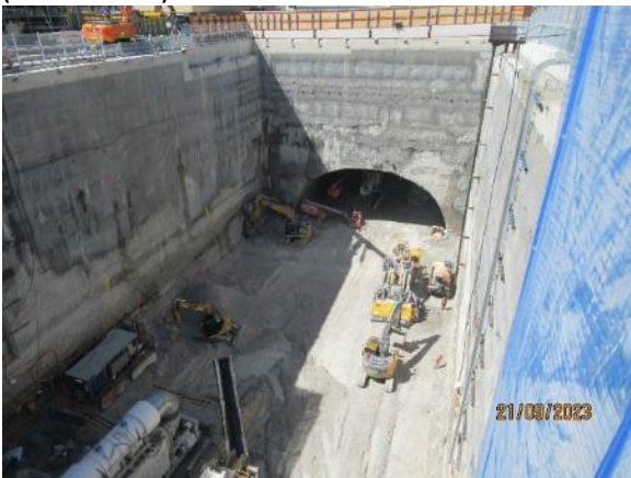
Figure 1.5 Central cavern opening into the west shaft. (Five Dock-east).
