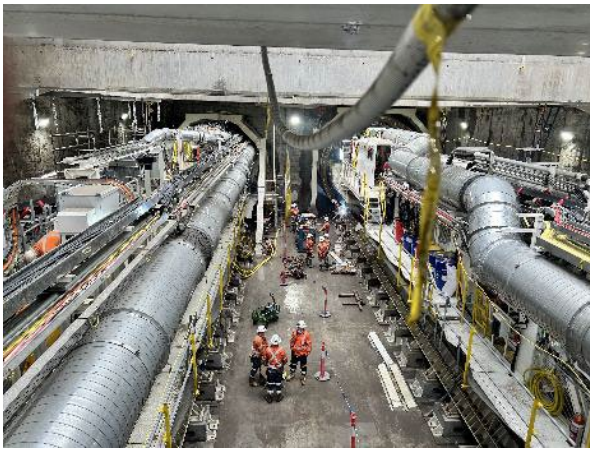
Figure 2.9: Rosehill Site – TBM 1 and 2
