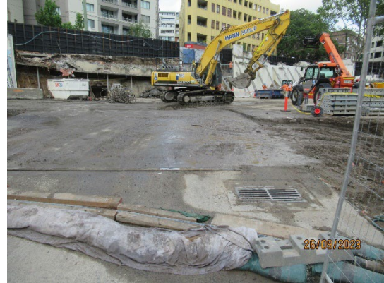
Figure 3.2 Pyrmont East: Completion of Stage 1 of hard demolition works
