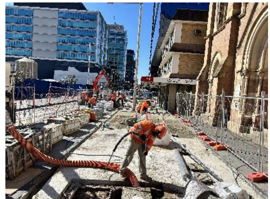
Figure 2.4: Parramatta site – Footpath paving works on Macquarie Street
