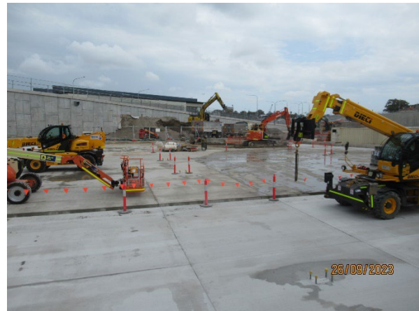
Figure 3.8 The Bays: FRP works for the haul road
