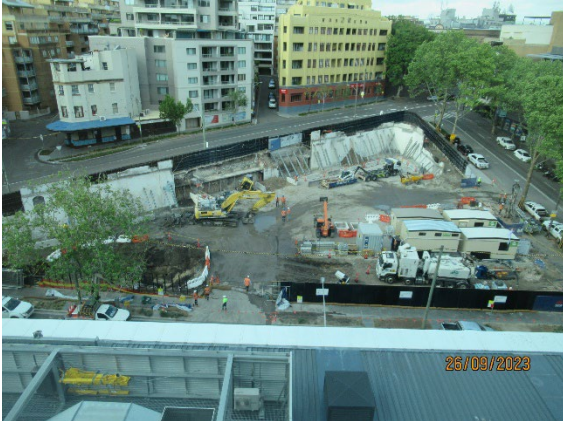
Figure 3.1 Pyrmont East: Completion of Stage 1 of hard demolition works
