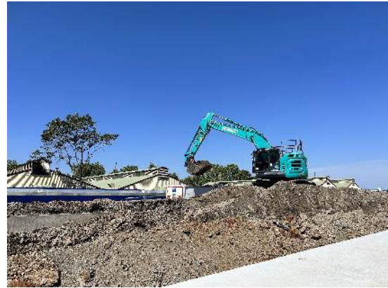
Figure 2.8: Clyde Dive site – Dive Structure excavation spoil load out
