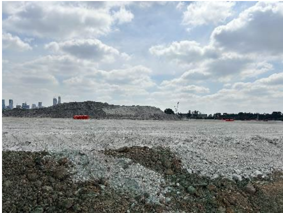
Figure 2.11: Clyde MSF Site – Earthworks
