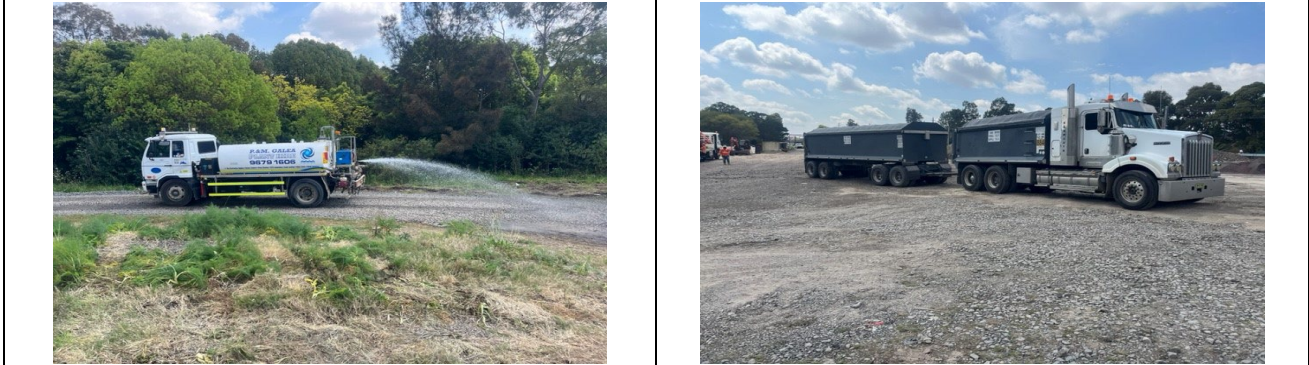
Dust suppression and covered loads in the Belmore Triangle laydown
