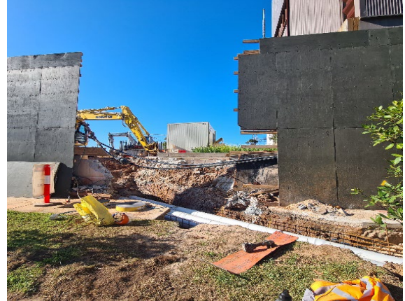
CDS: Trenching works for stormwater connection underway.
