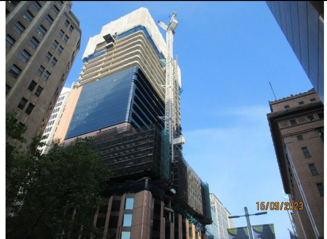
Martin Place South: View from Martin Place west of Castlereagh Street. Concrete pumping from Castlereagh Street.
