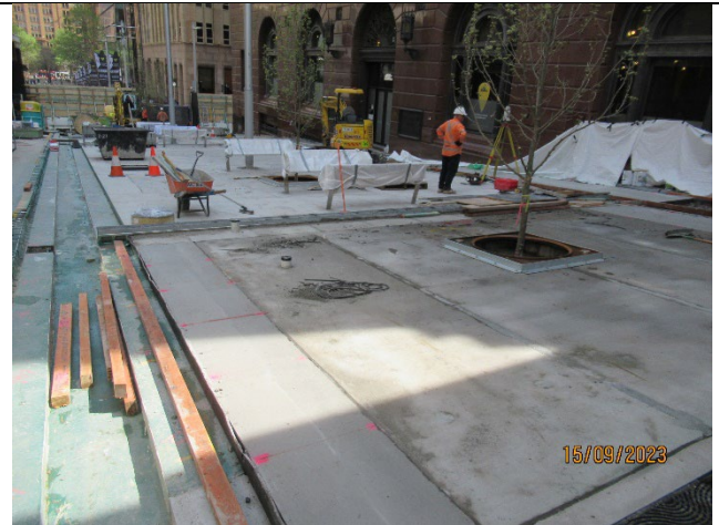
Martin Place: Ongoing works in the public space of Martin Place.
