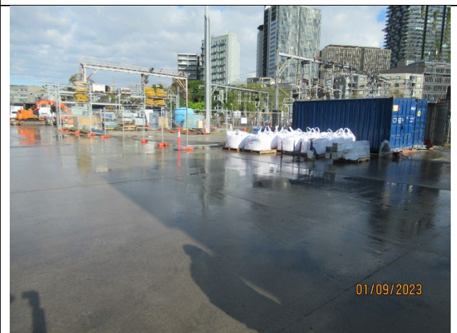
Sydney Yard: Area with temporary fencing for use by a Sydney Trains contractor, unrelated to Sydney Metro works.
