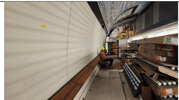
West platform installation of rest/seats
