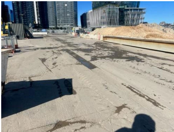
Dust generation from the hardstand an issue during high winds (water cart in use)
