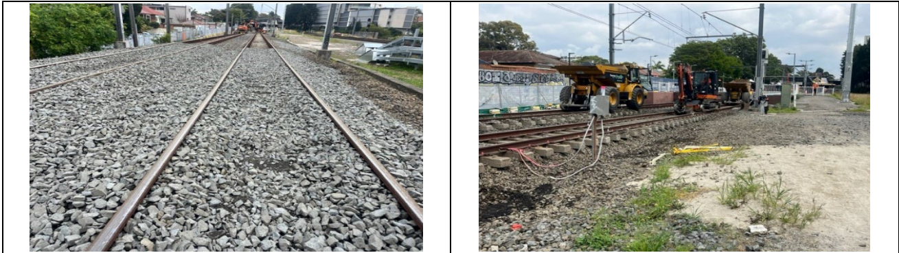
Track reconditioning including ballast skimming
