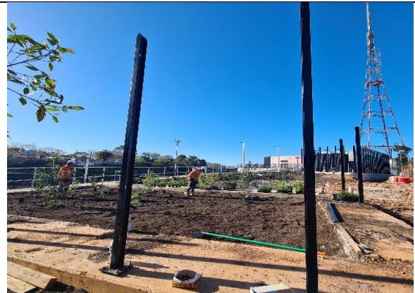
CDS: Detention basin works progressing – drainage, fencing and landscaping.
