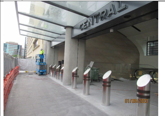
Eastern Entrance: View of entrance to Chalmers Street
