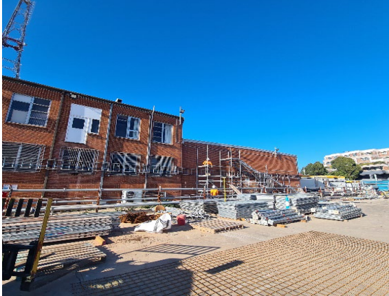
CDS: Scaffolding and light demolition preparatory works for Site workshop/crib sheds.
