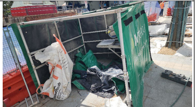
Clark Street – Noise tent installed for paving cutting (note in process of relocating during the inspection).
