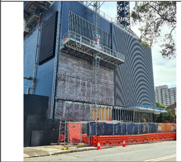
Southern Building: Façade and awning installation ongoing.
