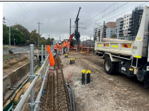
Piling for northern platform, Bankstown Station.
