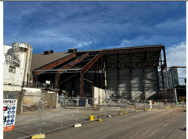
CDS: Spoil shed demolition ongoing.
