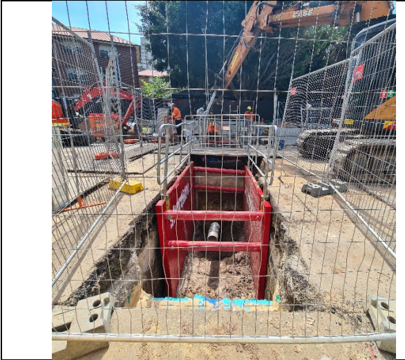
Cope St Site Compound: Stormwater works underway.
