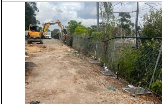
Security Fence installation, Punchbowl.
