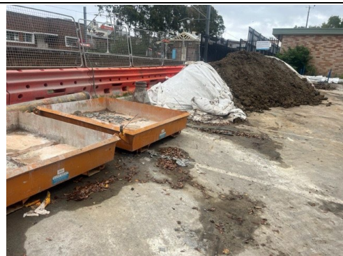
Materials storage, Bankstown Station compound.
