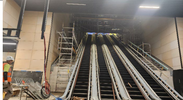
Pitt St North (PSN): public artwork and escalator installation.
