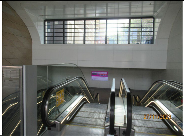
Eastern Entrance: Escalators in use by the public.
