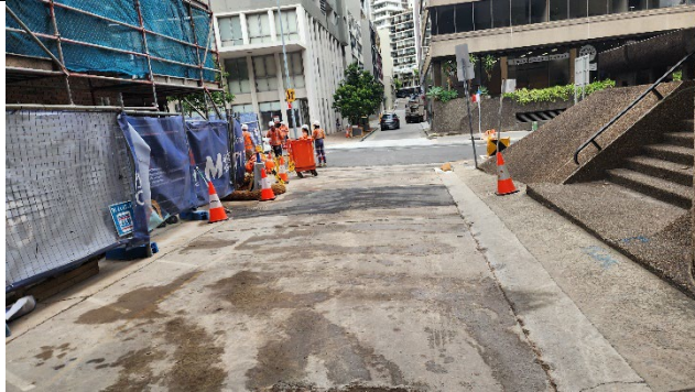
Clarke Lane North – the area was maintained with no tracking observed.
