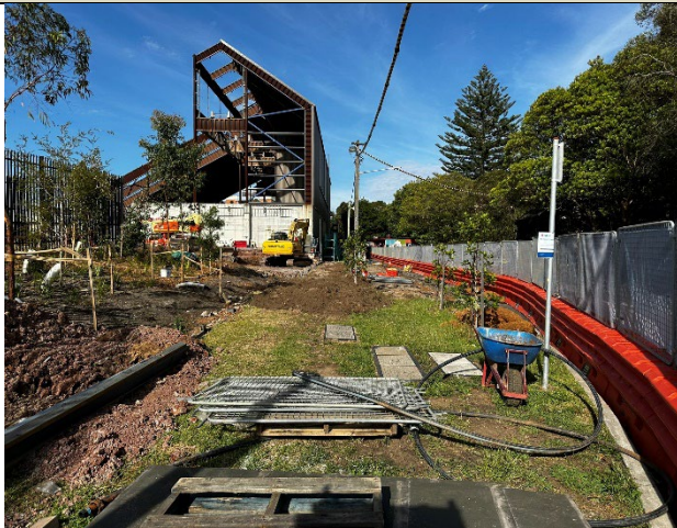
CDS: Frank Channon Walk works ongoing.
