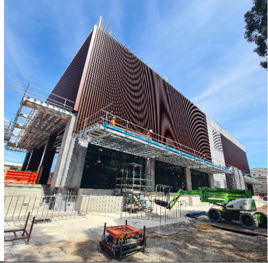
Northern Building: Waterloo signage, façade and awning installation; fit out and service works continuing.
