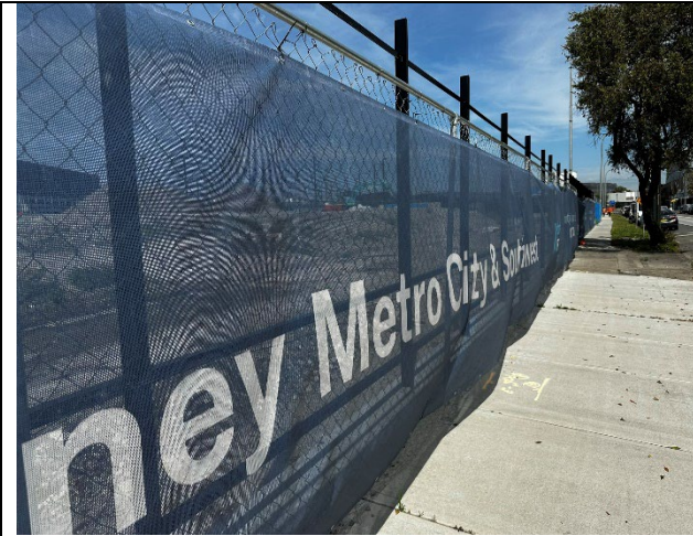
SMTF S: New fence installed on Edinburgh Rd.
