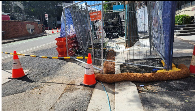
Clark Street Public Domain works – Coir logs and drain protection installed.
