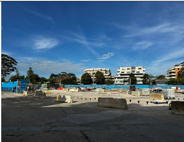
CDS: Amenities building demolished.
