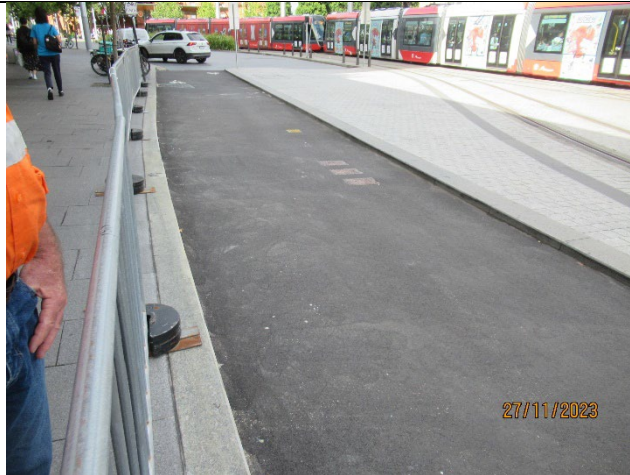
Eastern Entrance: View of the cycle path in front of the Eastern Entrance. Line marking has since occurred on the cycle path.
