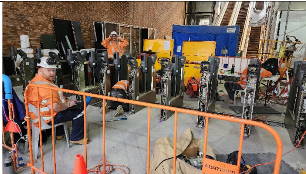
B1 concourse – Installation of opal card readers.
