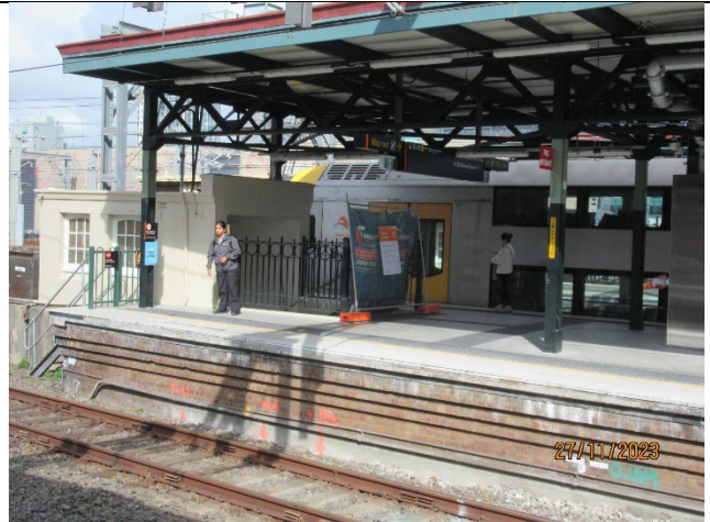
Platforms: Some remedial works in the baggage handling tunnel which was closed at the time of the ER inspection.
