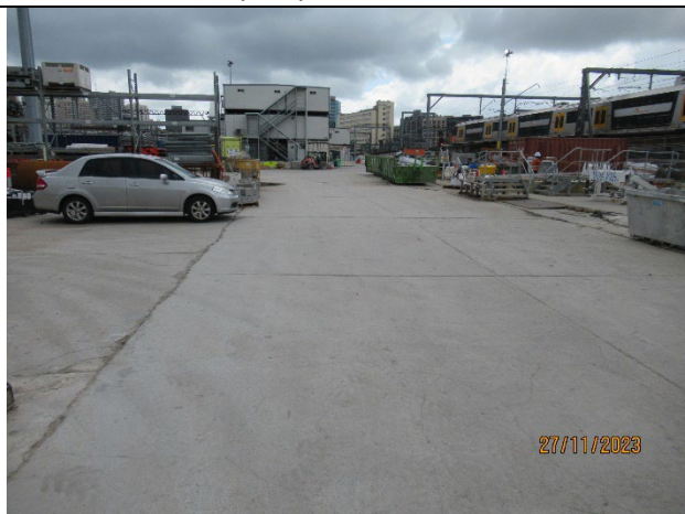
Sydney Yard: Ongoing removal of plant and equipment. Use of the Yard by a number of other contractors.
