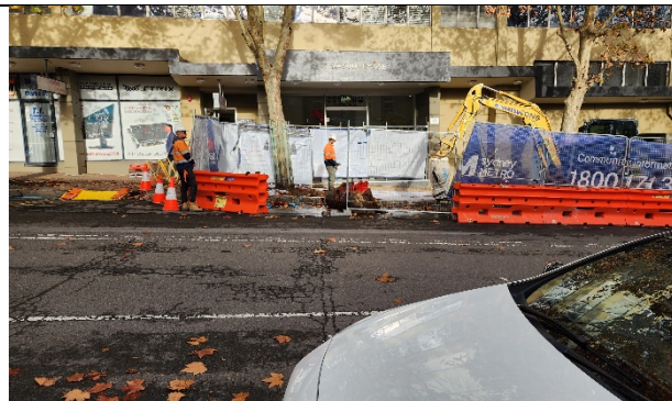
Clark Street utility works (17/5 - noise mitigation raised as ER action)
