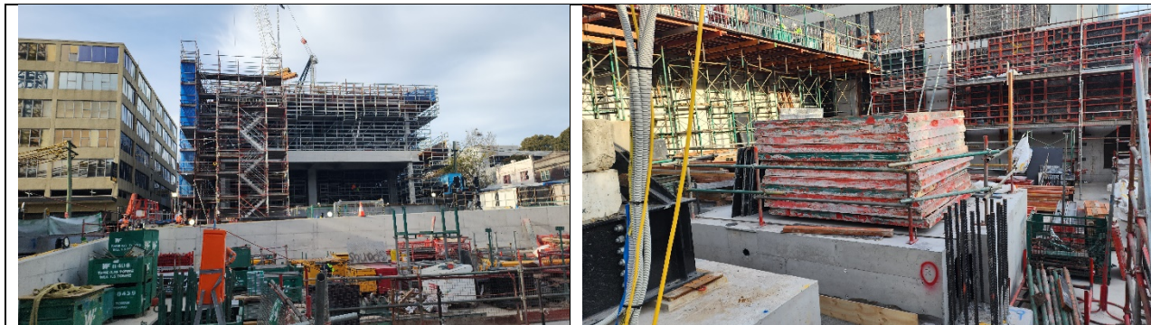
Hume Street Bridge and Site B
