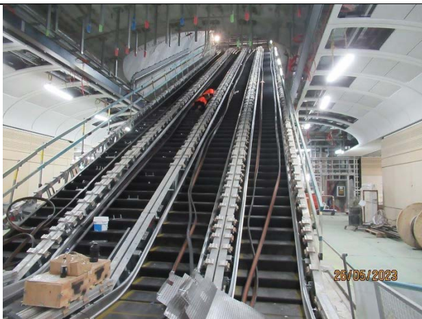
Caverns: Escalators under construction
