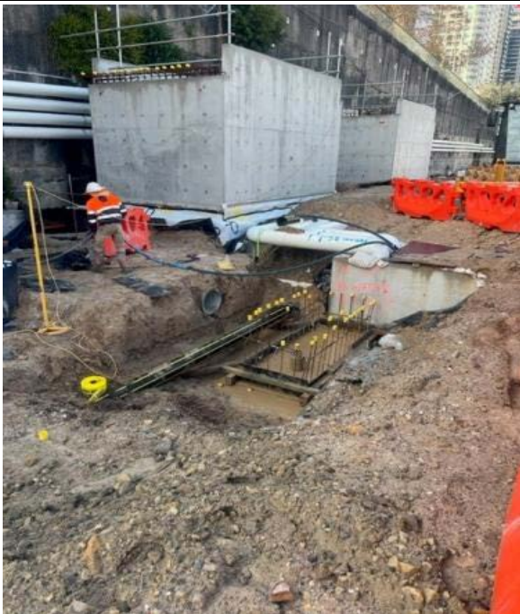
Ventilation pod installation ongoing; Backfill of services
