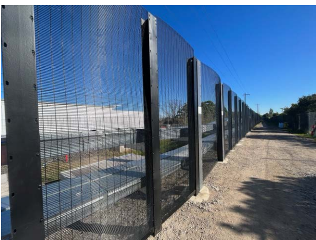
Security fencing mesh panel installation on site access, Stansfield Avenue, Punchbowl
