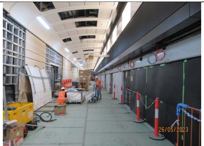
Station Platform: Ongoing fit out
