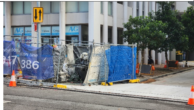
Oxley Street brick cutting noise mitigation (good practice)
