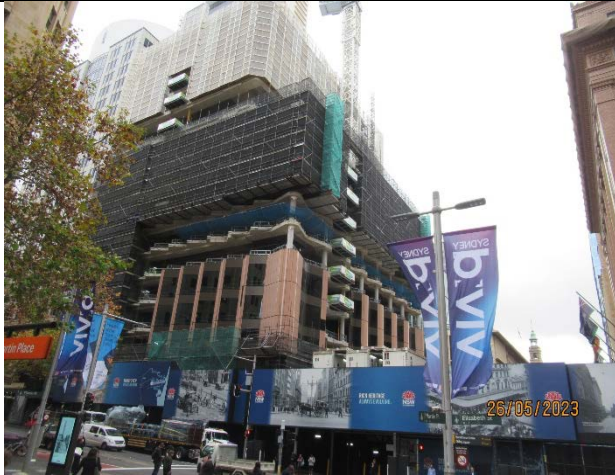
Martin Place South: View from street level. Façade under construction
