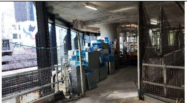
PSN: Level 4 glazing works
