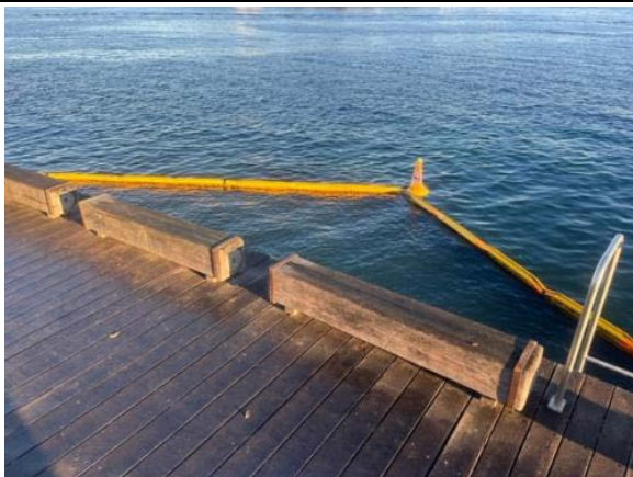
Sediment boom in place for H01-02 cleaning
