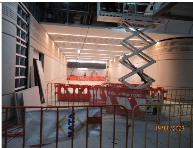
Caverns: Ongoing fit out
