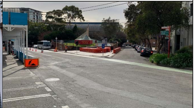
Hume St / Clark St intersection opened to the public
