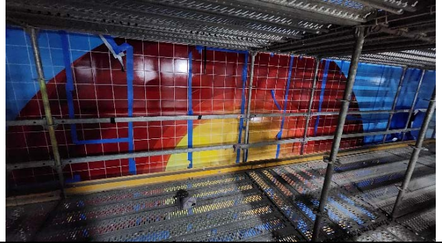
PSS: Public art installation Burke St entrance
