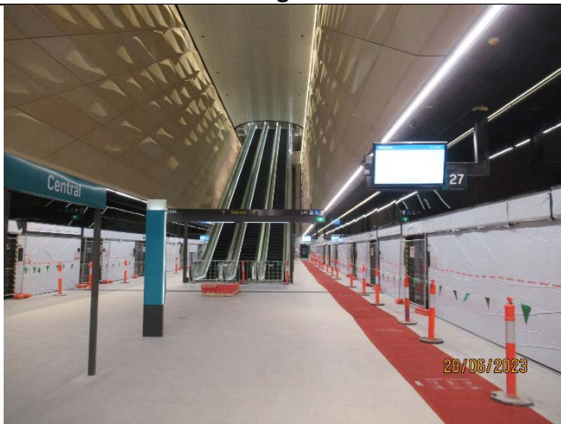
Metro Station: Completed and handed over to Sydney Metro
