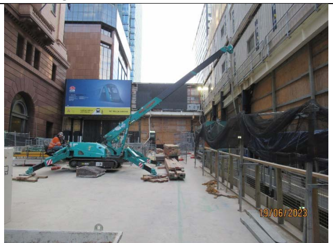
Martin Place – Public Area: Works in concrete slab
