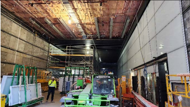
PSS Burke St Entrance wall tile and roof insulation installation
