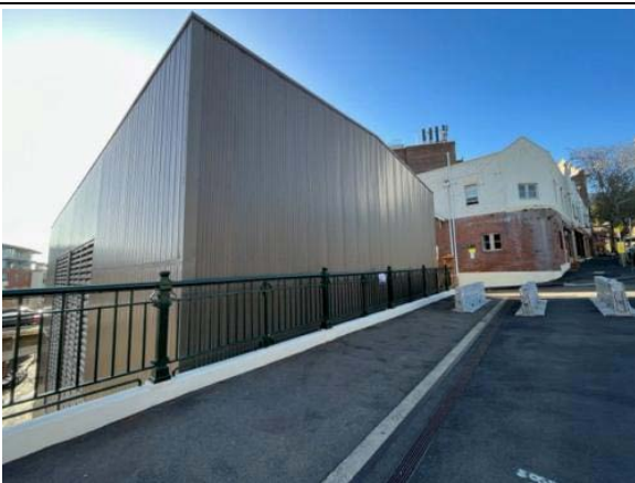
Heritage elements to be protected (bridges and fencing) during acoustic shed demolition
