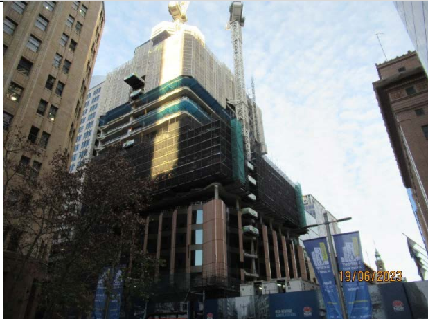
Martin Place South: View from street level. Ongoing façade construction.
