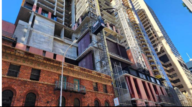
Pitt St South (PSS): façade installation - view from Pitt Street
