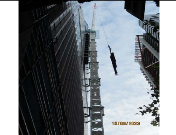
Martin Place North: Tower crane in use above Elizabeth Street
