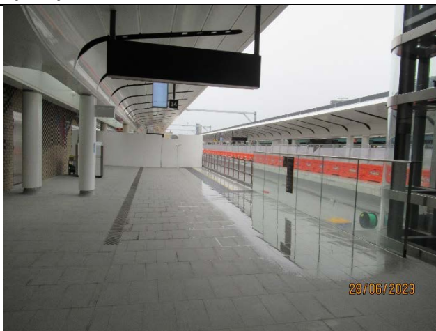
Platform 14: LOR scope generally completed
