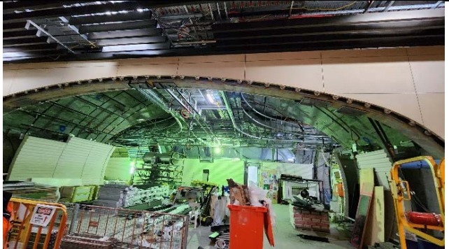
PSS Adit sandstone archway entrance from southern escalators
