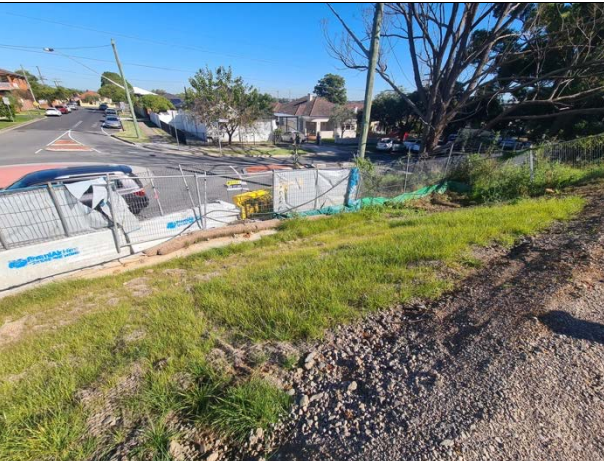
Punchbowl TSS: Noticeable grass growth continuing sections of batter previously hand seeded (positive observation). Sediment controls noted to remain.
