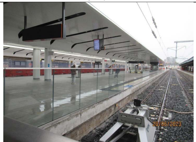
Platform 12: Handed over to Sydney Trains
