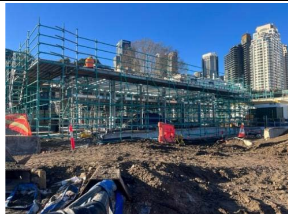
Construction of the above-ground escalator canopy
