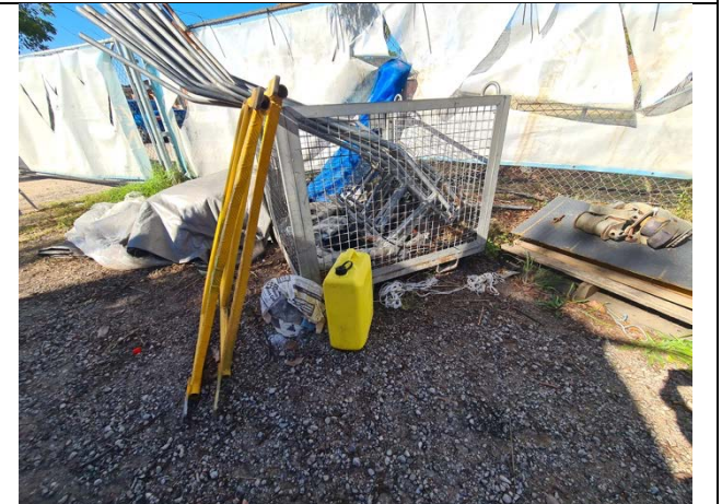
Belmore Site Compound: Jerry can without secondary containment was discussed and picked up during ER inspection, for relocation into appropriate chemical storage.
