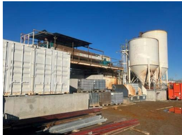
WTP set-up ongoing
