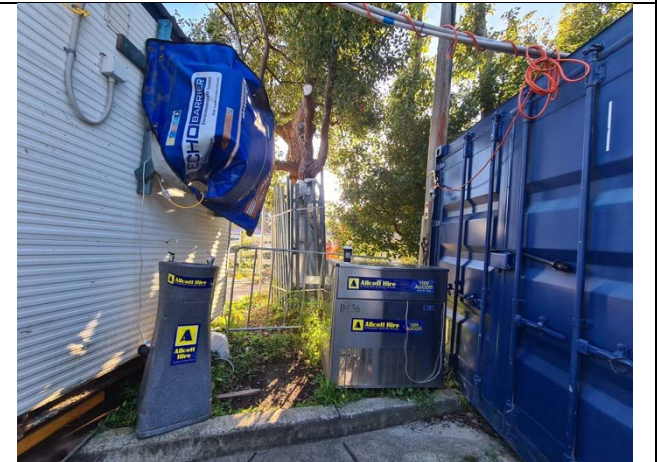
Dulwich Hill TSS: Noise blanket installed around AC unit of site shed and tree protection remains in place
