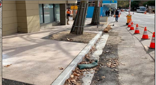
Clark Street – Asphalt repair works provided by AWE
