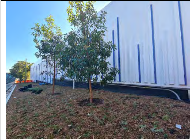
Punchbowl TSS: Landscaping works progressing.
