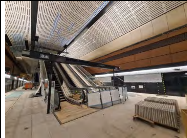
Station Cavern: Escalator installation/ testing continuing.
