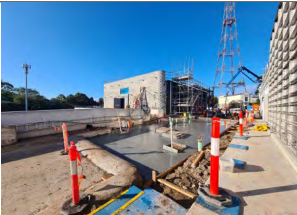
CDS: Concrete pour for driveway, to access track.
