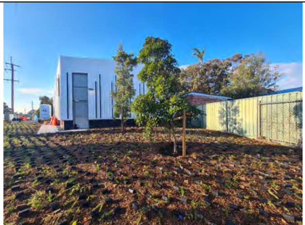
Dulwich Hill TSS: Landscaping works progressing.
