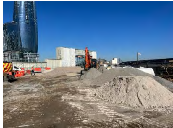
Hardstand to be scraped back where possible to reduce dust risk
