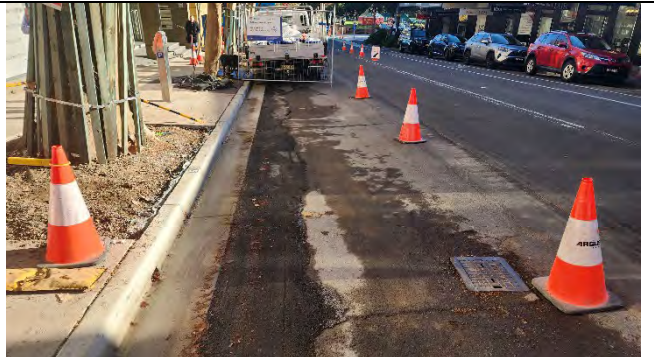
Clarke Street – asphalt tie-in work to gutter
