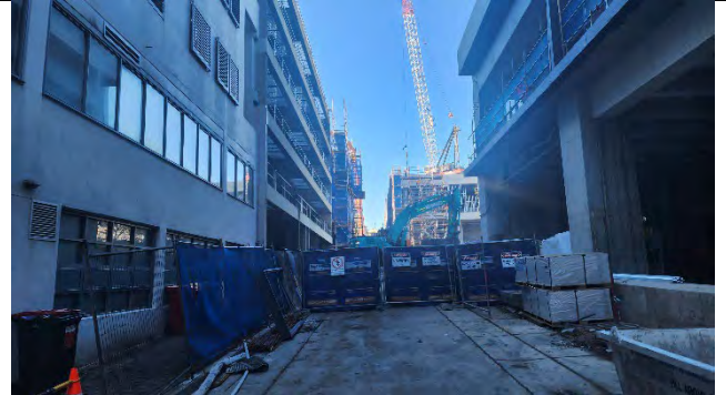
Clark Lane North removal of capping beam noise mitigation
