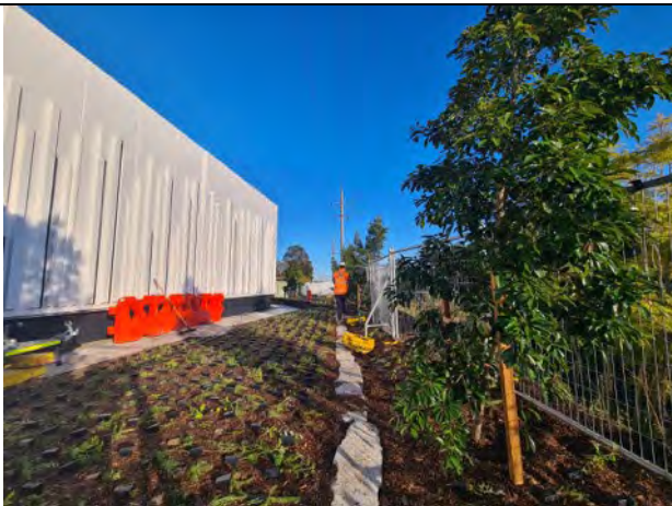
Dulwich Hill TSS: Landscaping works progressing.
