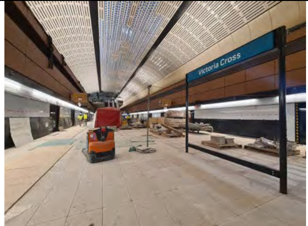
Station Cavern: Victoria Cross signage installed on Station Platform.
