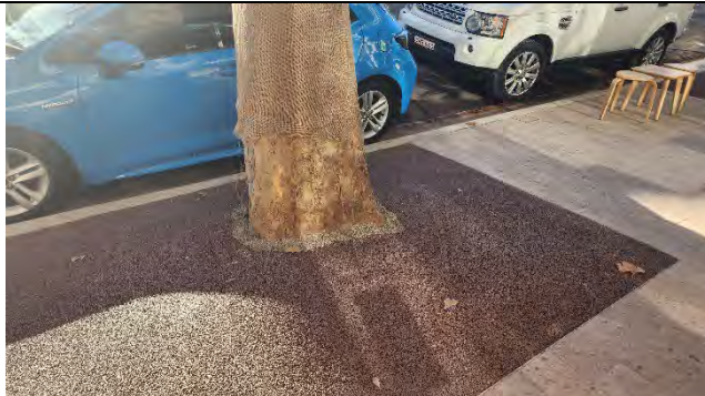
Clark Street Paving – completed areas
