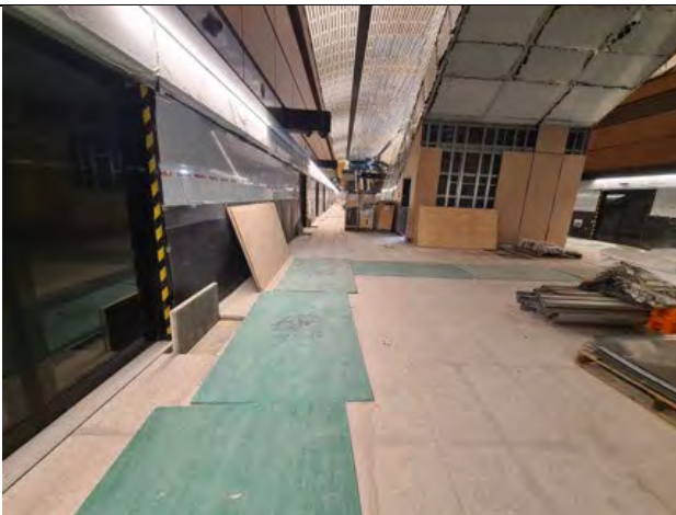
Station Cavern: Platform tiling works underway
