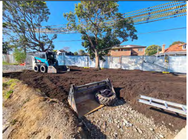
Lakemba TSS: Trimming and preparatory works for landscaping underway.
