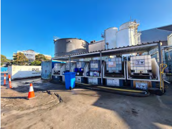
CDS: Construction WTP disconnected with tunnel water being directed to Marrickville.
