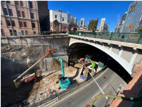
Demolition of the remaining eastern sections of the acoustic shed – investigation for potential damage to be conducted
