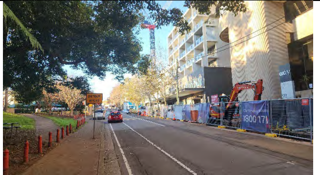
Clarke Street utility works
