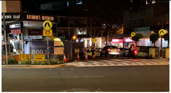
Clark Street – noise mitigation for OOH paving work
