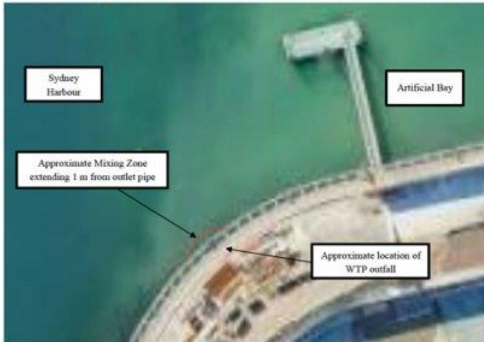
Figure 2 WTP discharge location at Nawi Cove
