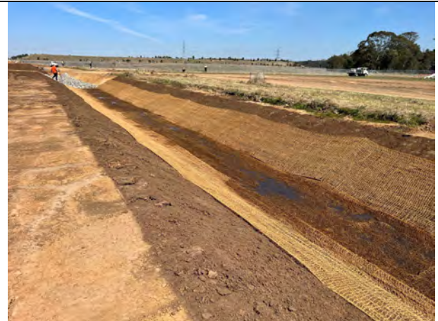
Blaxland Creek - Jute mat has been used effectively as scour protection in drainage lines at Blaxland's Creek.
