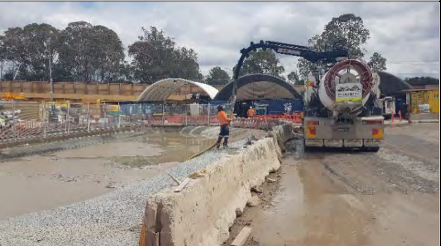
View west.– CPBG proactively implementing settling/holding ponds to manage water runoff.
