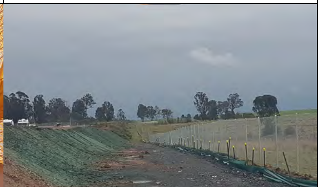
Aerotropolis view north: Eastern embankment batter stabilised and sed . fence improved.
