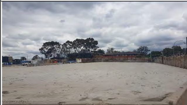
View south east along Phillip St.: Plaza laydown demobilised and cleaned.
