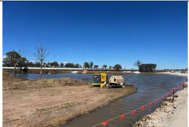
Defence - Water is still being drawn down from the pondage near the Warragamba pipeline
