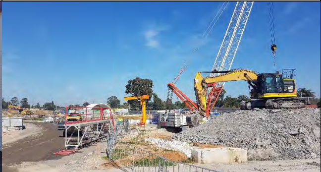
Claremont Meadows: View south west with final spoil pile in foreground.
