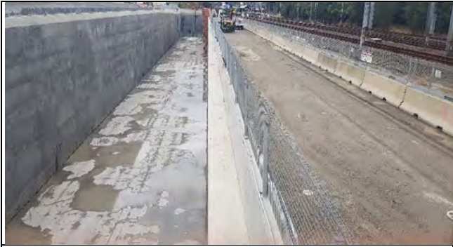
St Marys: view east of completed station box
