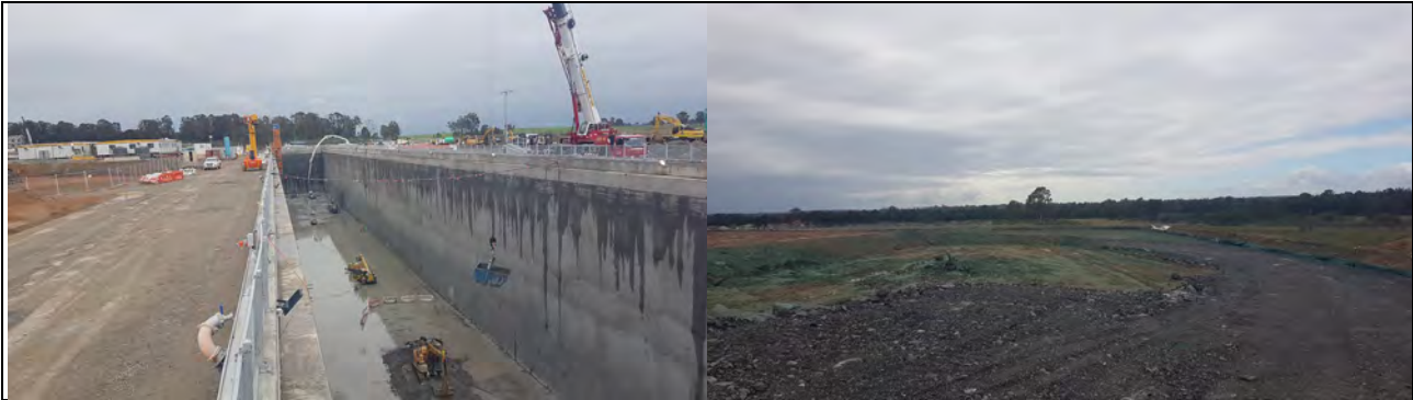
Aerotropolis view north: Station box completed.
