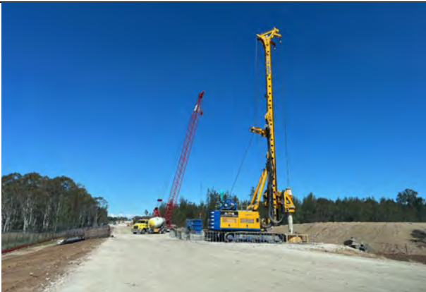
Defence - Piling has progressed and is almost complete on Defence land
