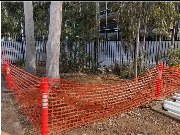
Tree protection zones were in place with paraweb fencing
