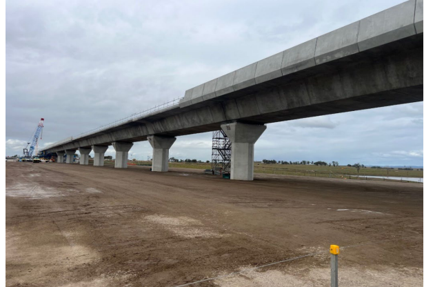
Viaduct works are progressing
