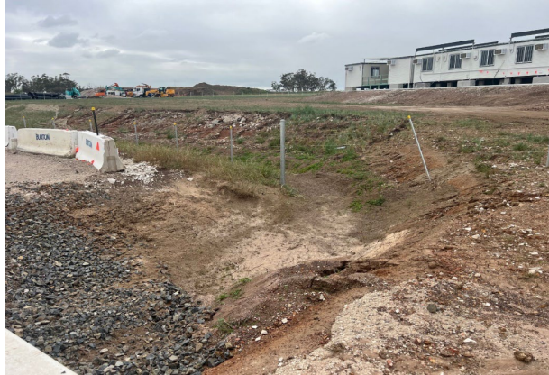
Parts of the SSTOM batter have slipped. SCAW to determine who is responsible for fixing this
