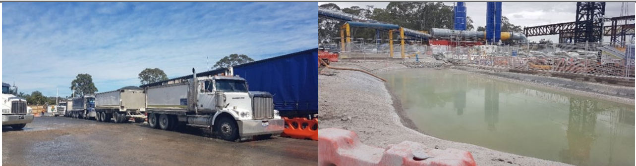
Orchard Hills: TBM spoil materials haulage intensifying - 7 am to 10 pm.
