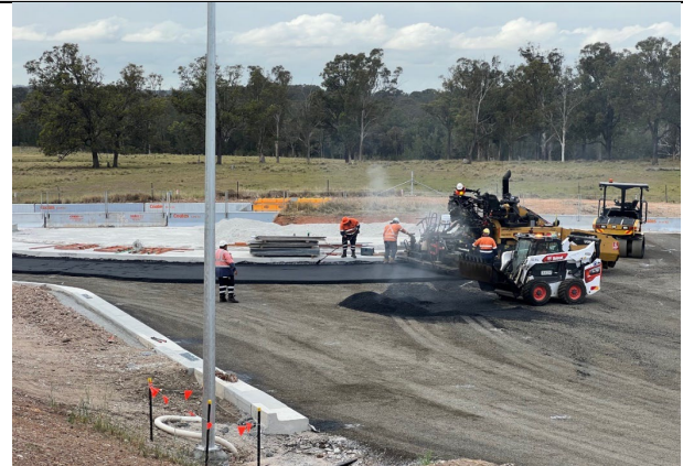
Works continue on the roundabout prior to the lane possession
