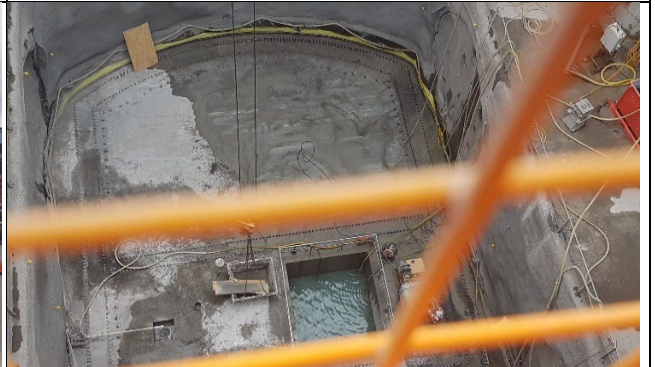
Bringelly: Shaft base slab and sump completed with dewatering ongoing.
