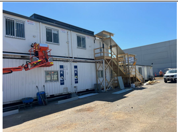
The site compound continues to be built
