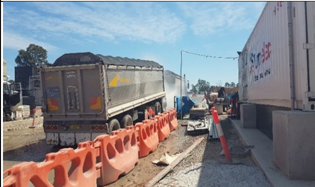
Orchard Hills– Wheel wash in operation.
