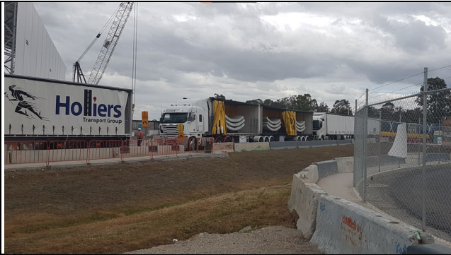
Orchard hills view west: Queuing of segment delivery heavy vehicles onsite.
