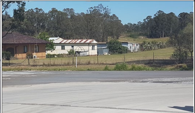
Orchard Hills – Tracking noted from site access on Kent Rd.
