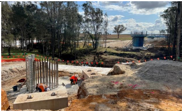
Cosgrove's Creek - Structures works have crossed south of Cosgrove's Creek
