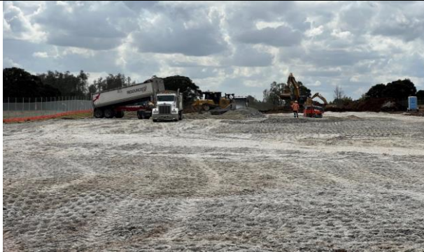
Defence Land - Sandstone import continues on the Defence site
