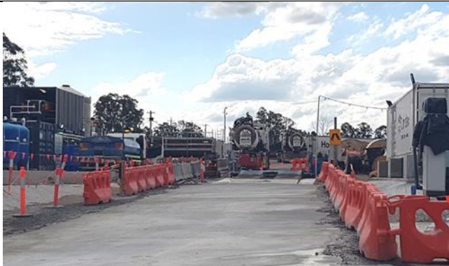
Orchard Hills view north from station box: Automated wheel-wash being installed
