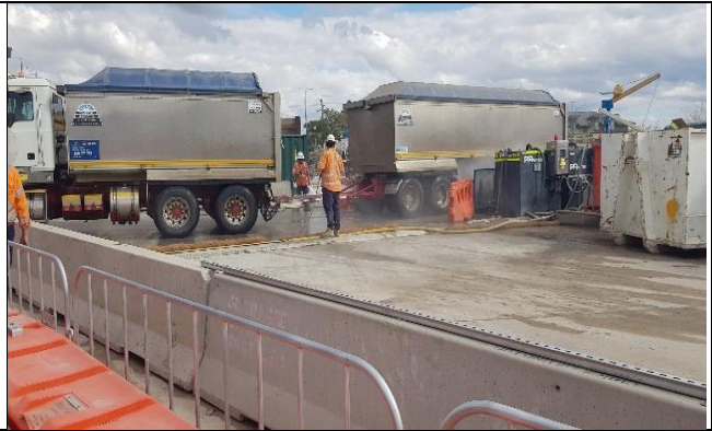
St Marys: Manual wheel washing following automated wheel wash.
