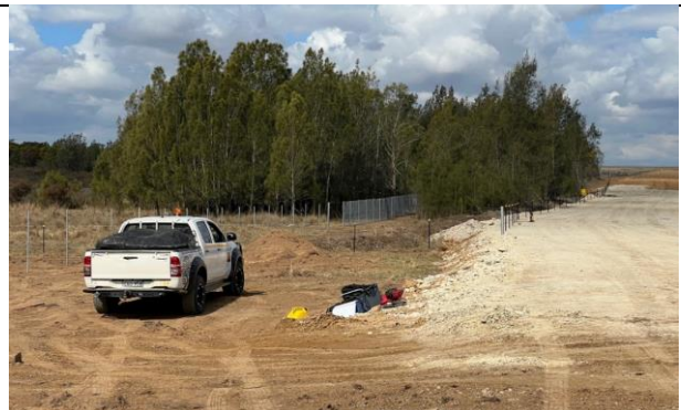
Cosgrove's Creek - Fencing works is ongoing south of Cosgrove's Creek
