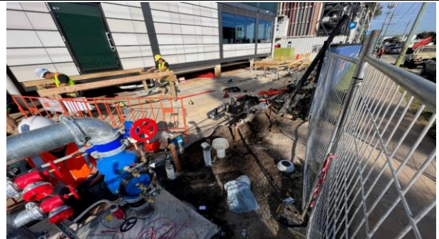
SPO - The sewer backfill is progressing, posing a minimal environmental risk
