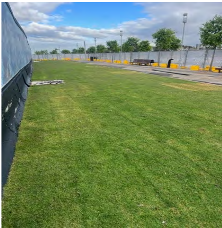
Landscaping works ongoing
