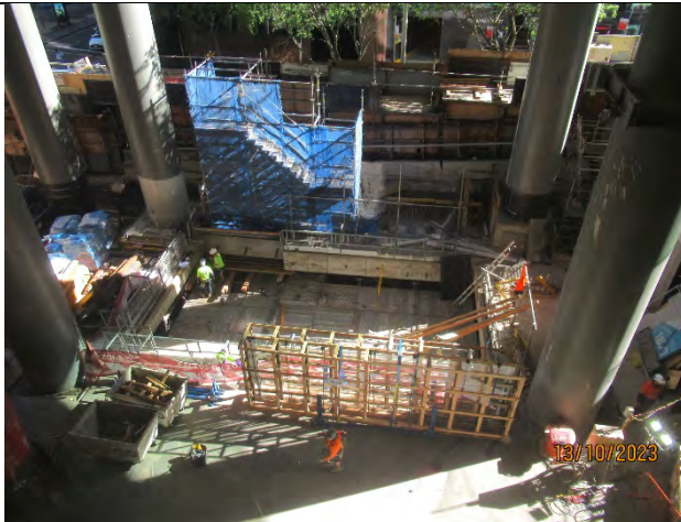
Martin Place North: Foyer area.
