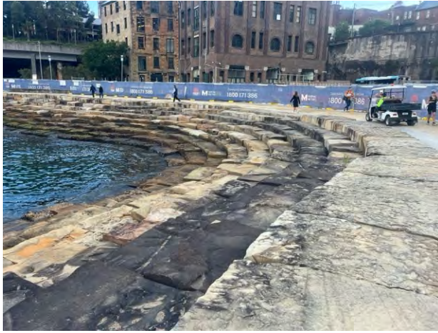
Pedestrian scaffold bridge removed from over Nawi Cove steps
