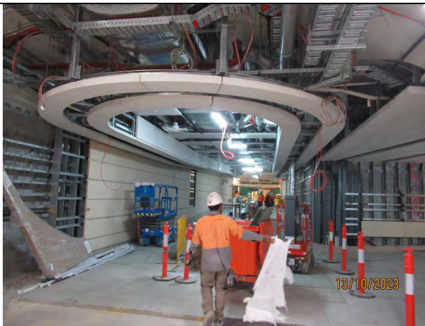
Caverns: Ongoing fit out.
