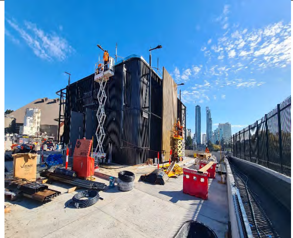
Northern Dive Building: Façade installation progressing.
