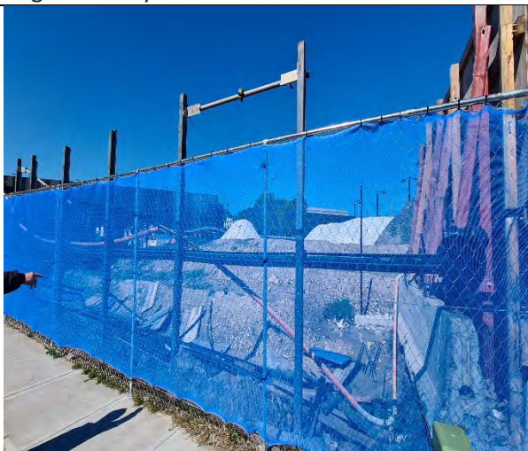
SMTF S: Hoarding removal in progress on Edinburgh Rd.
