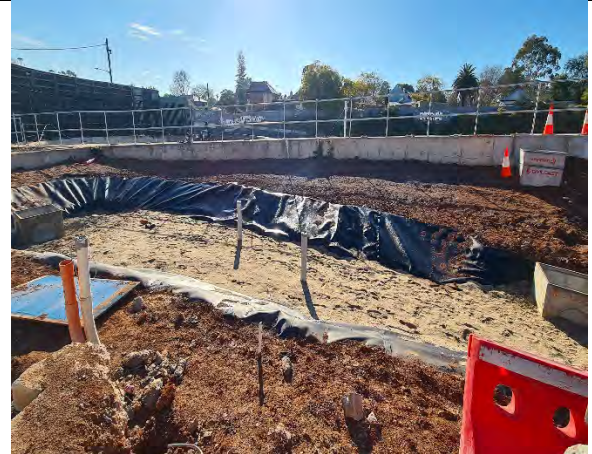
CDS: Detention basin works in progress.
