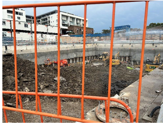
Figure 2-6 Ongoing excavation of the west shaft (FD).
