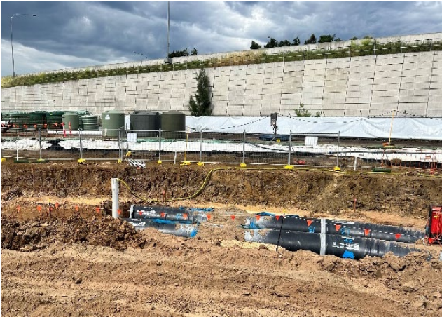
Figure 4.9: Clyde MSF Site – New Watermain being installed in the Utilities Trench
