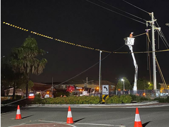
Figure 3.1: North Strathfield Station – OH Wire removal
