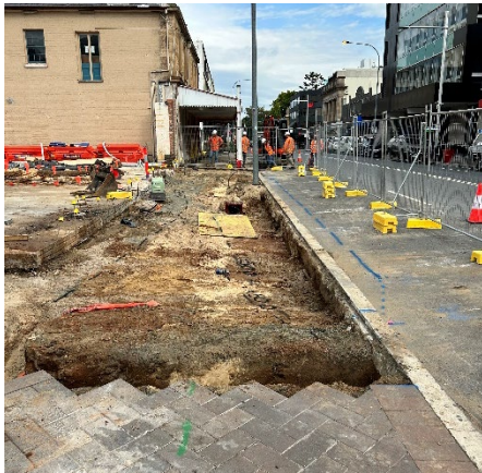
Figure 4.3: Parramatta Site – Footpath restoration works
