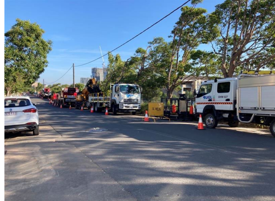
Figure 3.2: North Strathfield Station – Site set up
