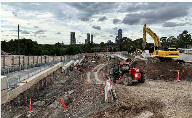
Figure 4.1: Westmead Site – Station Box excavation
