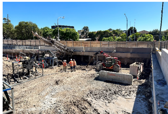
Figure 4.2: Westmead site – Station box excavation and soil nail installation
