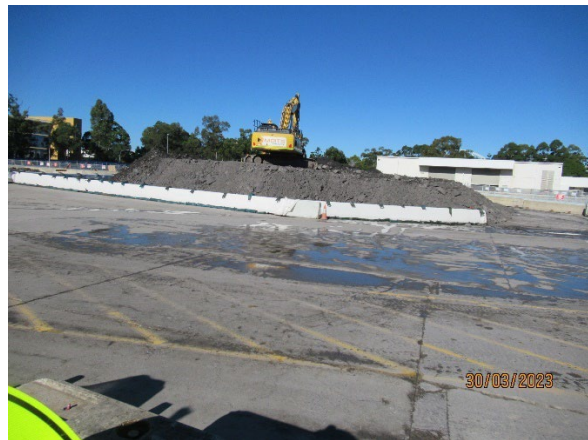
Figure 2-8 Loadout of spoil from the excavation of the Station Box (SOP)
