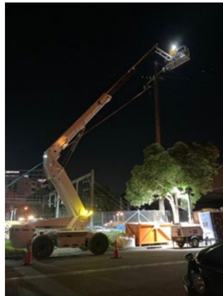
Figure 3.4: North Strathfield Station – OH Wire removal
