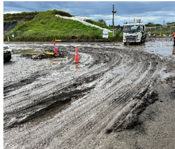
Figure 4.10 – On site Haul Road improvements required at Clyde MSF
