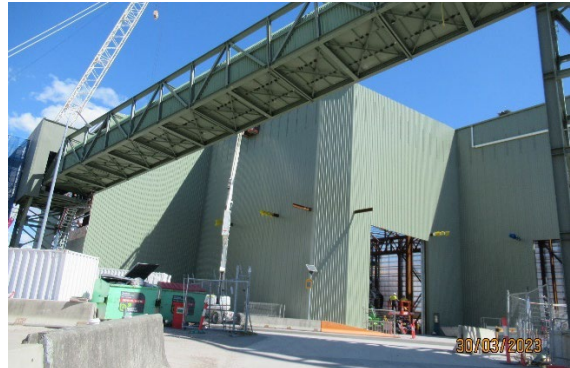
Figure 2 2 Placement of acoustic panelling on the Segment shed ongoing. (The Bays).
