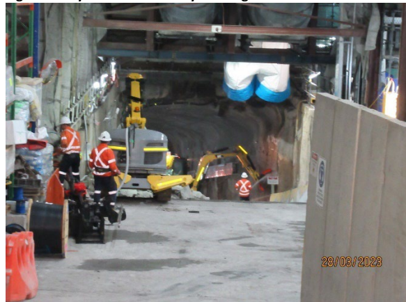
Figure 5 6 Hunter Street East: Works within the acoustic shed
