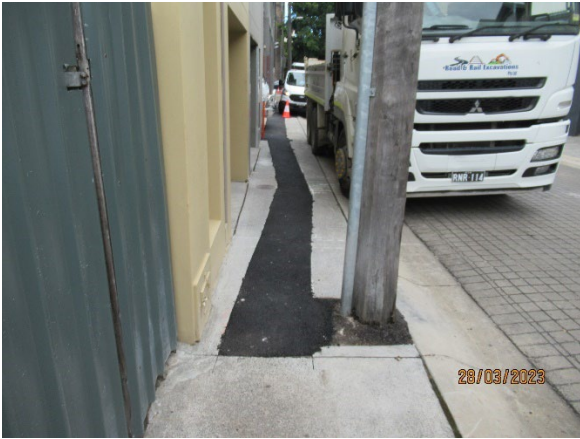
Figure 5 1 Pyrmont West: Undergrounding of electrical cables on Paternoster Row
