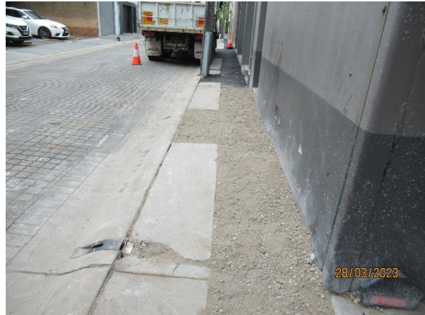
Figure 5 2 Pyrmont West: Undergrounding of electrical cables on Paternoster Row
