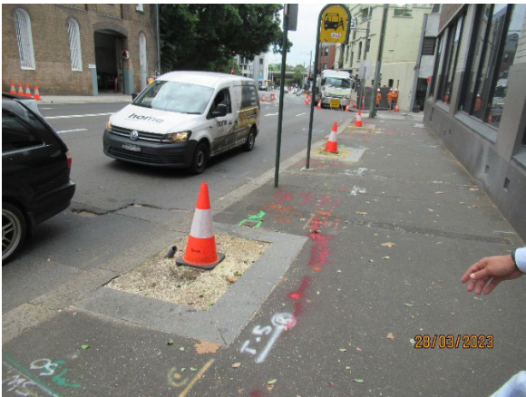
Figure 5 3 Pyrmont West: Tree removal along Pyrmont Bridge Road
