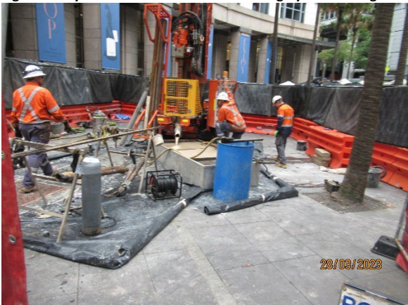
Figure 5 5 Geotechnical Borehole drilling; Chifley Square
