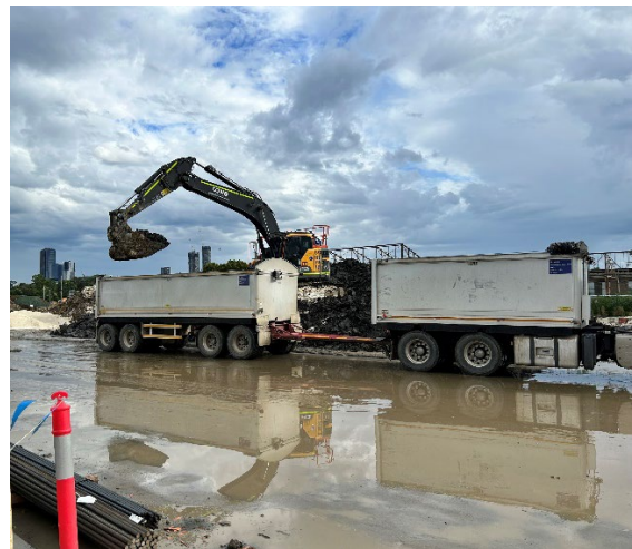
Figure 4.8: Rosehill Site – Treated ASS Spoil load out.
