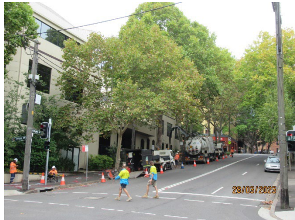
Figure 5 4 Pyrmont East: Utility Investigations
