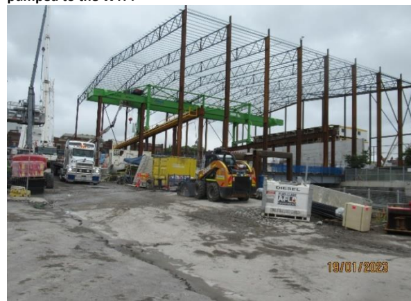
Figure 2 4 Ongoing construction of frame of the acoustic shed (Burwood North)
