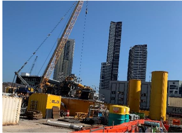
Figure 4.4: Parramatta site – Bentonite Plan mobilisation
