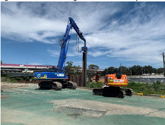
Figure 4.11: Clyde MSF site – Duck River sheet piling
