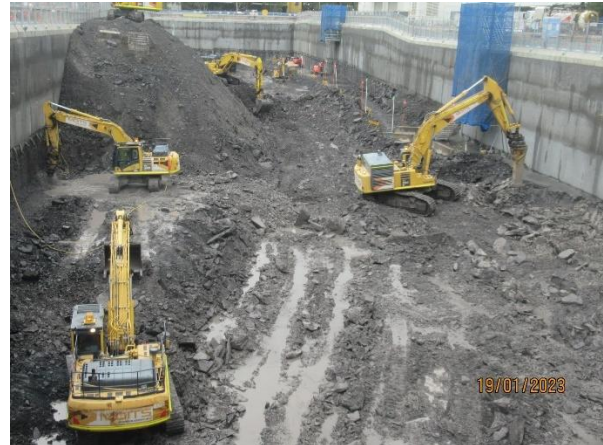
Figure 2-6 Ongoing excavation of the station box (SOP) using dozers and excavators
