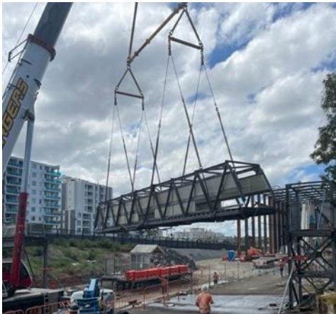
Figure 4.7: Clyde Dive site – heritage bridge relocation
