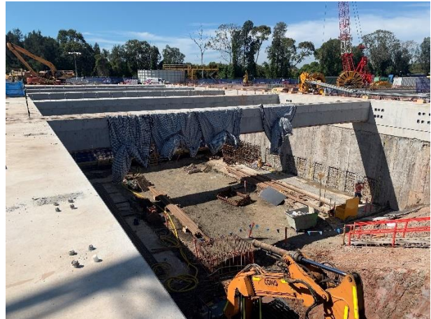
Figure 4.10: Rosehill site – TBM launch box excavation
