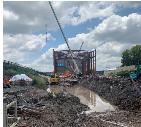
Figure 4.8: Clyde Dive site - Acoustic Shed construction
