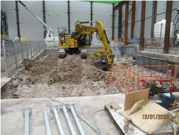
Figure 2-5 Ongoing excavation of the eastern shaft within the acoustic shed (Five Dock-east).
