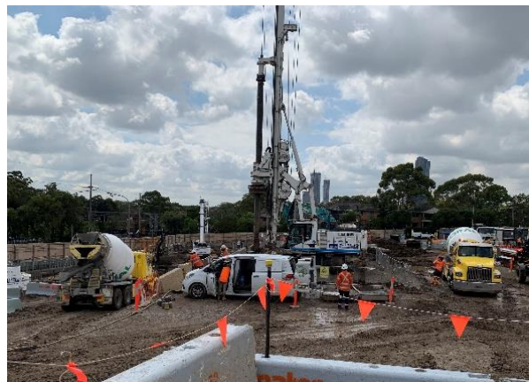
Figure 4.2: Westmead – Station box piling
