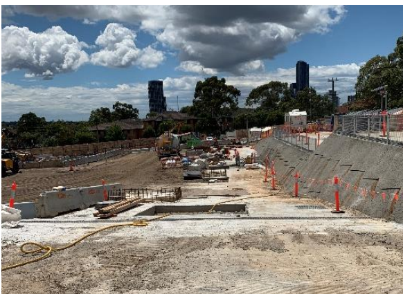
Figure 4.1: Westmead Site - Haul Road Construction
