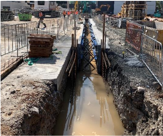
Figure 4.3: Parramatta site – Guide Wall excavation and concrete works.
