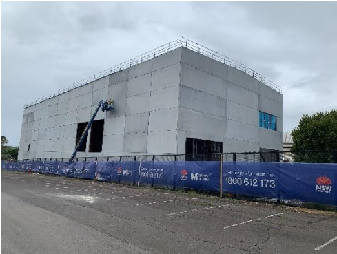
Figure 4.5: Clyde Dive site – Acoustic shed construction
