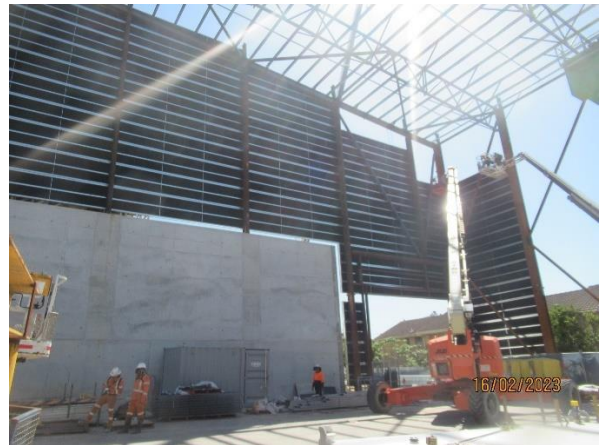
Figure 2-4 Installation of panels for the acoustic shed (Burwood North)
