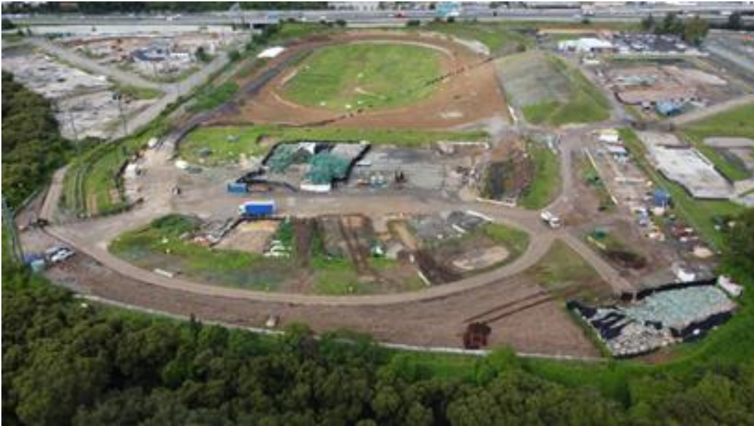
Figure 4.11: Clyde MSF – waste and spoil storage
