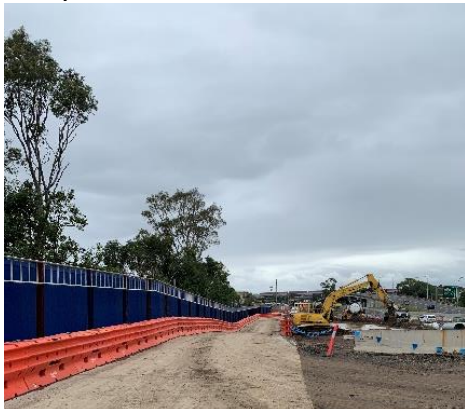
Figure 4.7: Clyde Dive – Noise wall along ATC boundary completed
