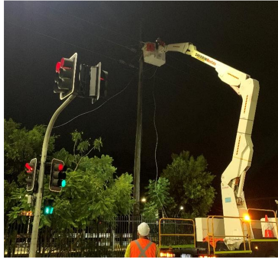
Figure 3.2: Westmead Station– cables and insulators being removed
