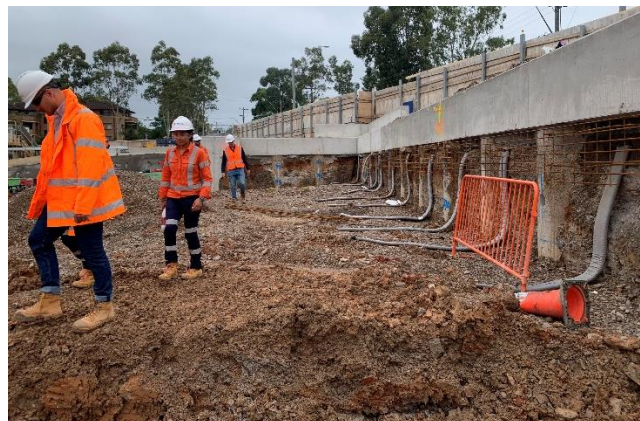
Figure 4.2: Westmead site – Station box excavation has commenced
