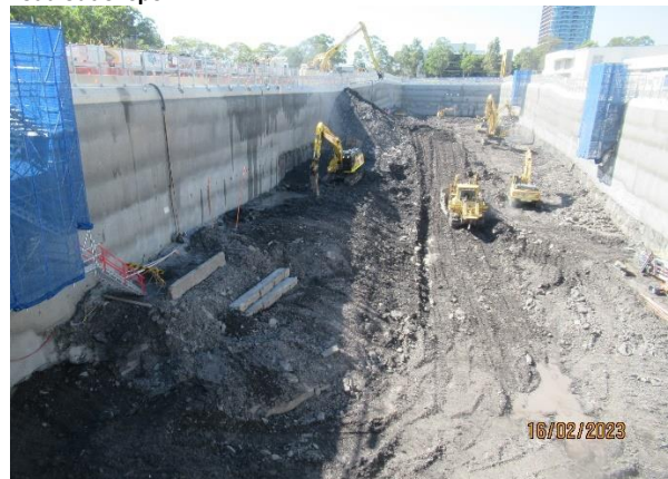
Figure 2-8 Ongoing excavation of the Station Box using dozers and excavators (SOP)
