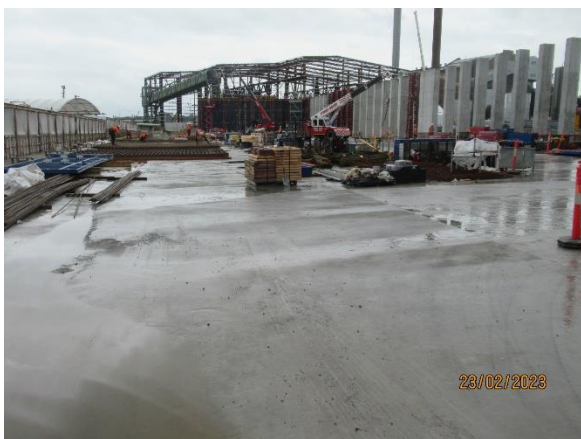
Figure 2 1 Ongoing large concrete pours for the Spoil shed foundations and wall supports (The Bays)
