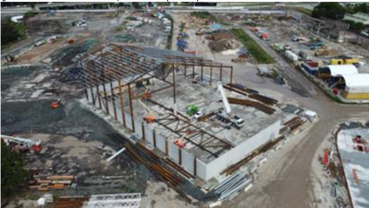
Figure 4.10: Rosehill – Spoil shed
