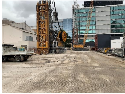
Figure 4.4: Parramatta Site – D-wall excavation
