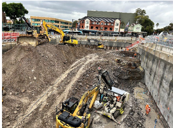
Figure 1.6 Ongoing excavation of the west shaft (FD).
