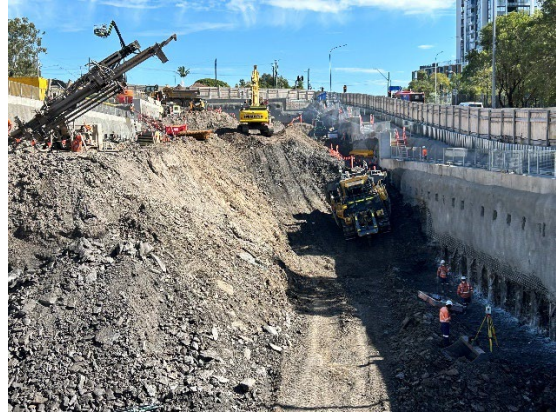
Figure 3.2: Westmead site – Station box excavation and soil nail installation
