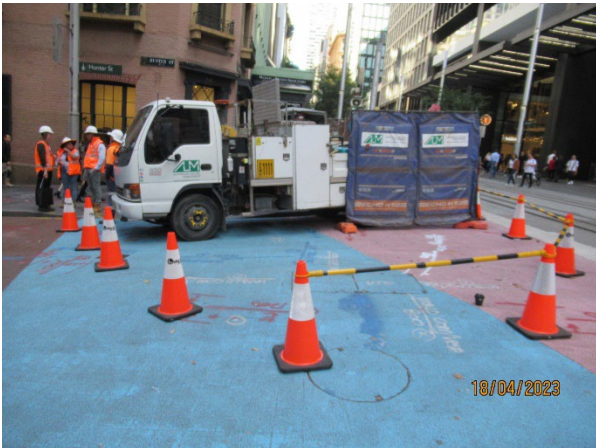
Figure 5 3 Hunter St West: Coring in preparation for geotechnical drilling.
