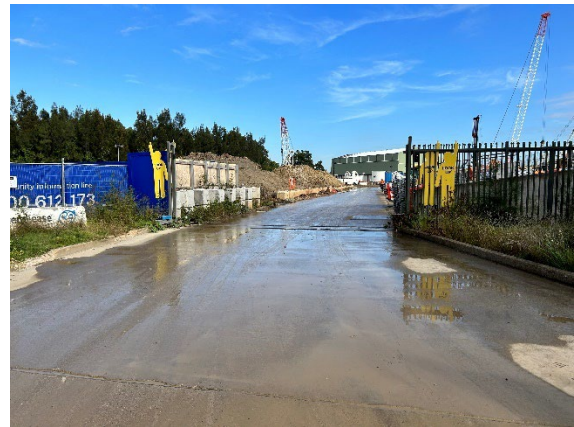
Figure 3.8: Rosehill Site – Hard stand requiring cleaning to prevent mud tracking
