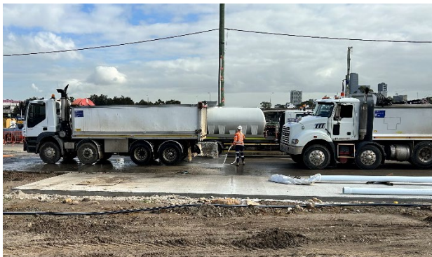
Figure 3.9: Clyde MSF Site – Wheel washing prior to entering Wentworth Street
