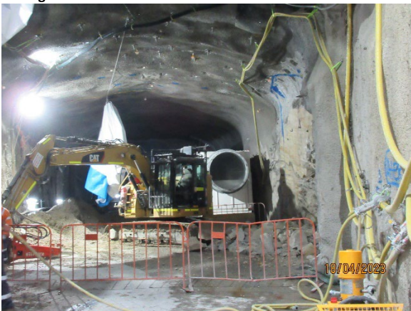
Figure 5 5 Tunnel decline: Setting up for road header to commence the tunnel.
