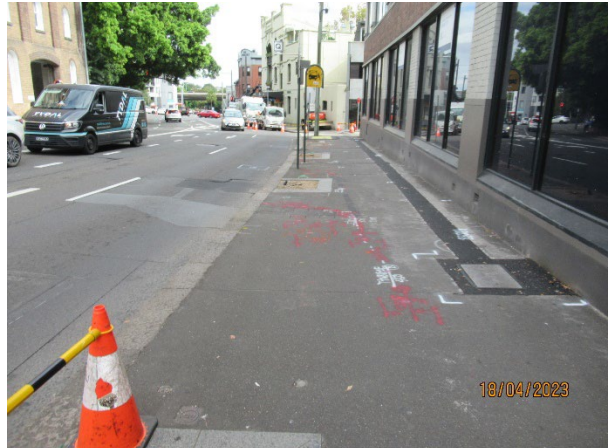
Figure 5 2 Pymont West: Utilities works on Pymont Bridge Road
