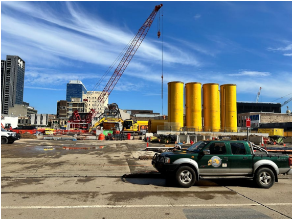
Figure 3.3: Parramatta Site – Bentonite Plant assembly and hardstand cleaning
