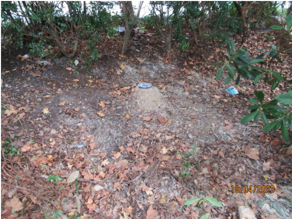
Figure 5 1 Pymont East: Installation of a groundwater monitoring well inside a borehole.
