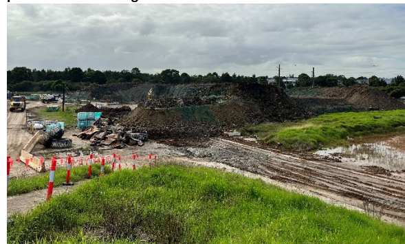
Figure 3.10 – Spoil stockpiling awaiting Speedway backfilling
