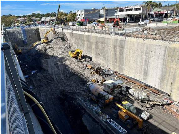
Figure 1 3 Excavation of the eastern end of the station box (Burwood North).
