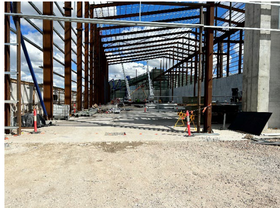
Figure 1 2 Ongoing construction of the frame of the spoil shed. (The Bays).
