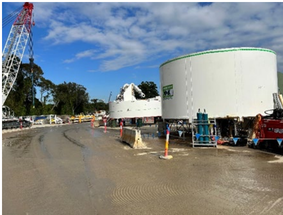
Figure 3.7: Rosehill Site – TBM assembly
