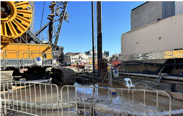
Figure 2.5: Parramatta Site – D-Wall excavation with cutter adjacent to Roxy Theatre
