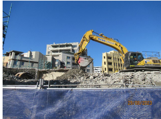
Figure 3.2 Pyrmont East: Sorting of demolition wastes in preparation for load out
