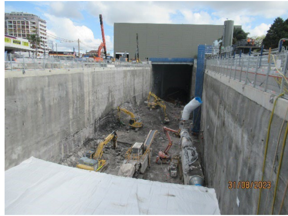
Figure 1.4 Station Box excavation works. (Burwood North)
