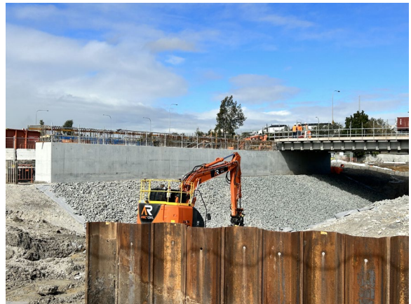
Figure 2.12 – Clyde MSF Site – Duck Creek diversion construction with rock armour
