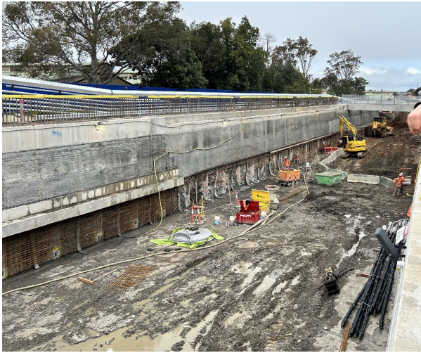
Figure 2.7: Clyde Dive site – Dive Structure excavation along the ATC boundary
