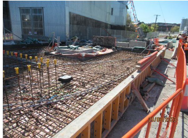
Figure 3.8 The Bays: FRP works for the sub-station footing
