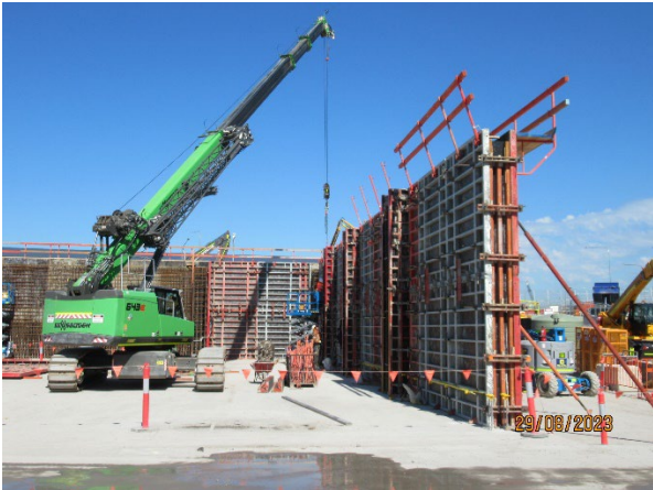
Figure 3.7 The Bays: FRP activities for the Spoil Shed
