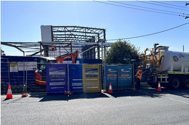
Figure 2.3: Westmead Site – layback removal on Bailey Street with inadequate noise mitigation
