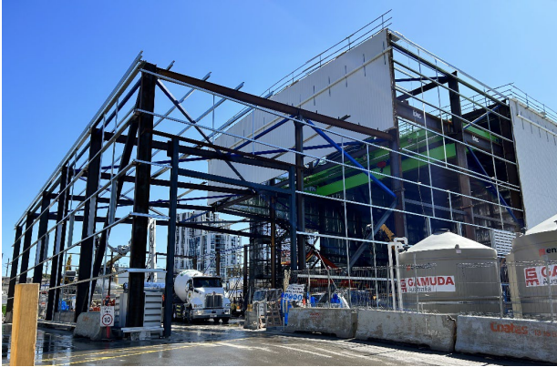
Figure 2.1: Westmead Site –Acoustic shed construction nearing completion
