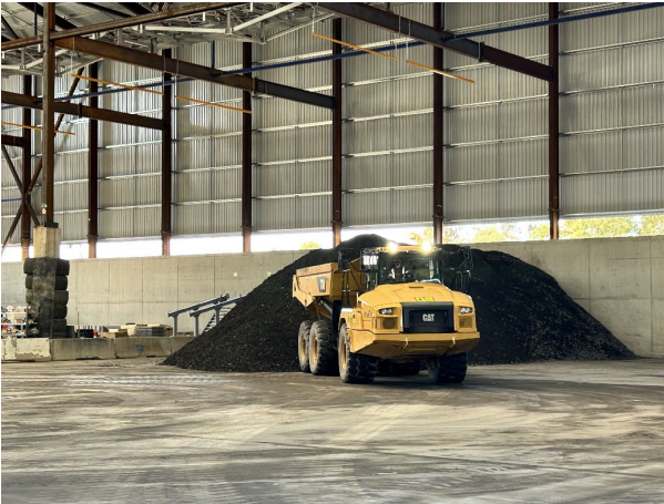
Figure 2.9: Rosehill Site – TBM spoil being stored in spoil shed
