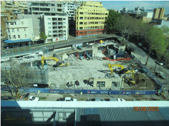
Figure 3.1 Pyrmont East: Ongoing hard demolition works
