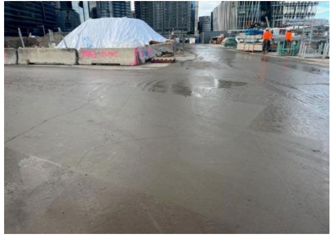
Sweeper in use and stockpiles covered
