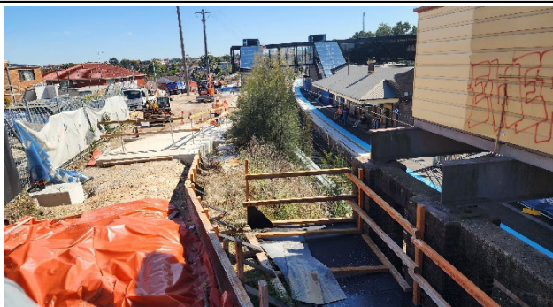
Dulwich Hill Plaza – Footpath tie in work ongoing
