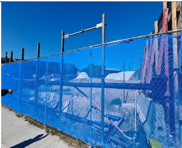
SMTF S: Hoarding removal in progress on Edinburgh Rd.
