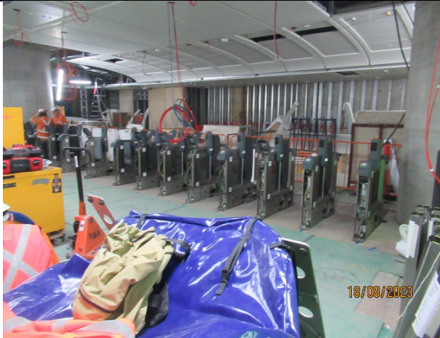
Martin Place North: Ticket gates being installed.
