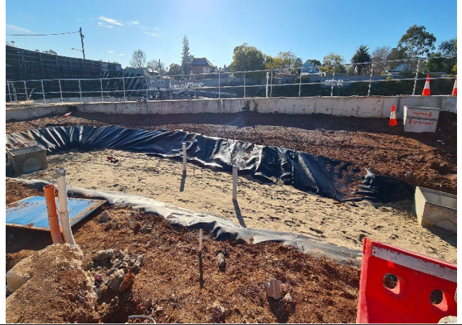
CDS: Detention basin works in progress.
