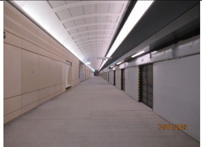
Stations: Completion of works at station platforms.
