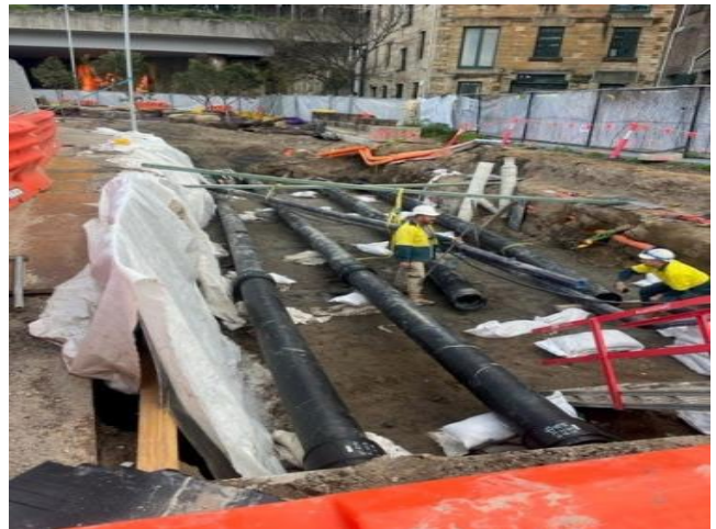
Condensed water pipework installation
