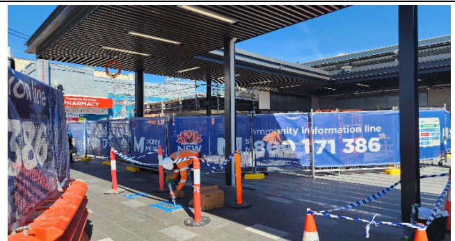
Campsie – Installation of concourse lighting
