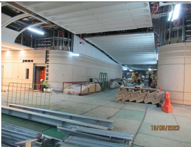
Caverns: Ongoing fit out works.
