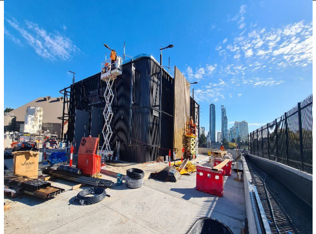
Northern Dive Building: Façade installation progressing.
