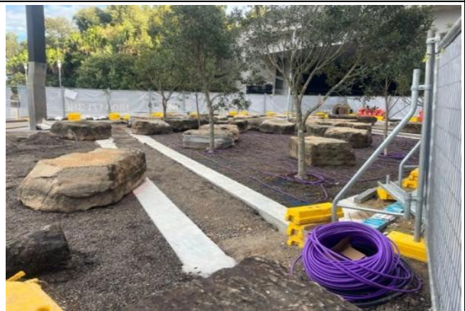
Landscaping including tree replacement ongoing in Zone 5
