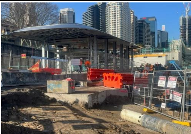
Lift and escalator canopy construction
