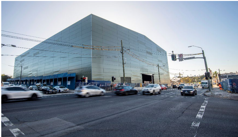
Figure 2-1: Burwood North construction site showing the existing acoustic shed
