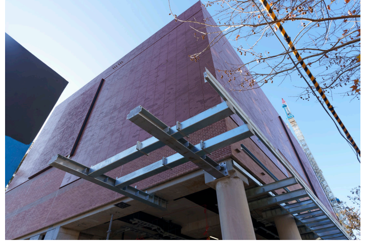
Façade of the Victoria Cross northern entrance building.
