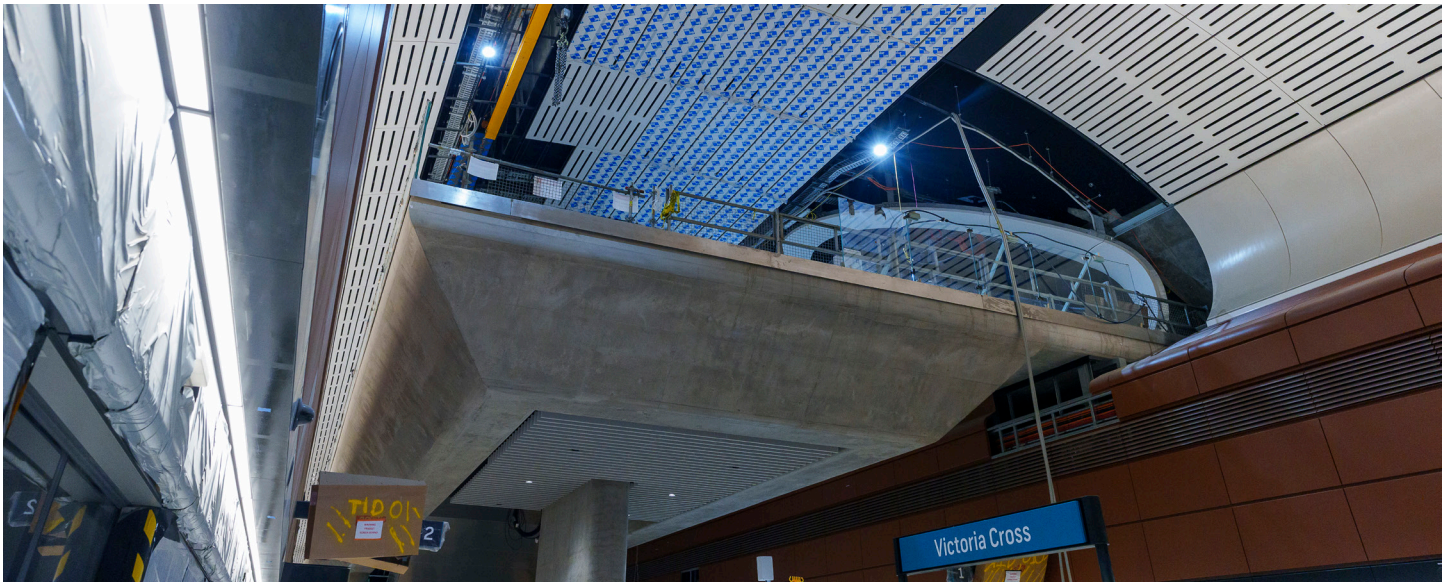
Fit out underway in Victoria Cross Station.
