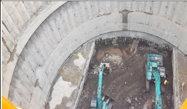
Bringelly Services Facility: Services shaft excavation nearing completion.
