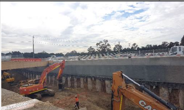
Orchard hills:View north east of excavation under Lansdowne Rd. bridge.
