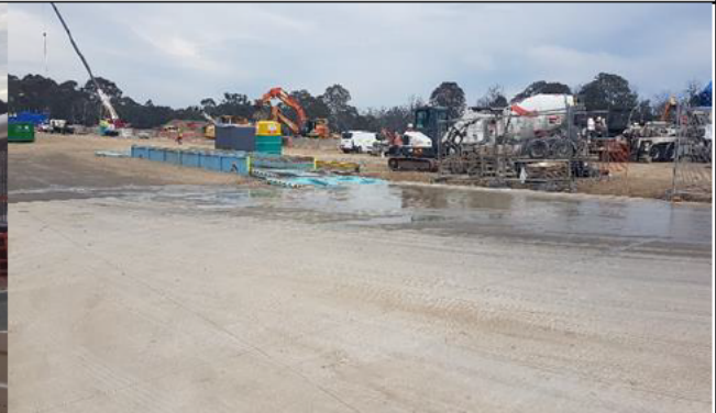
Lansdowne Rd. view south west – Wheel wash installed at eastern access.
