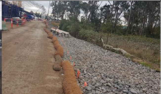
View north of Orchard Hills eastern haul Rd: Good ErSed controls noted but storage in swale to cease
