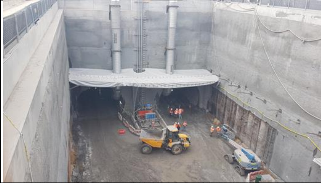
St Marys east: Stub tunnel excavation using roadheader.
