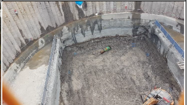
Claremont Meadows Services Facility: Services shaft excavation nearing completion.
