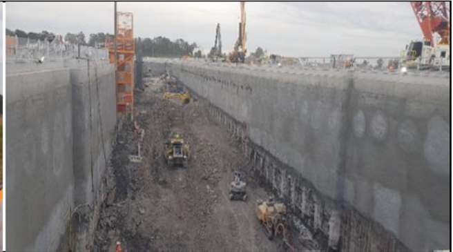
Aerotropolis station box: View north of excavation anchor and shotcrete works.
