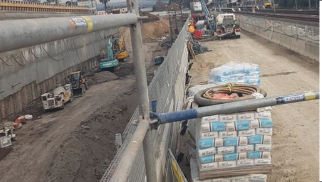
St Marys: Central to West station box excavation and shotcreting.
