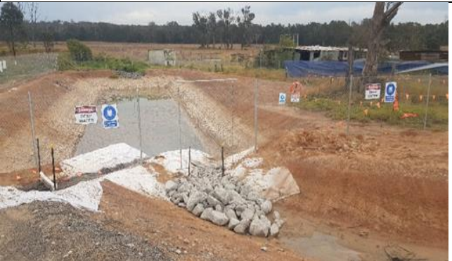
Bringelly Services Facility: Sediment basin and inlets well installed and managed.
