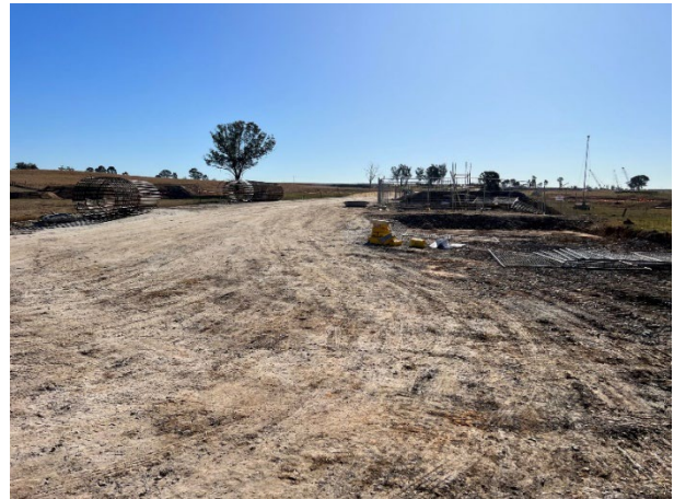
Luddenham South - Piling works continue at Luddenham South
