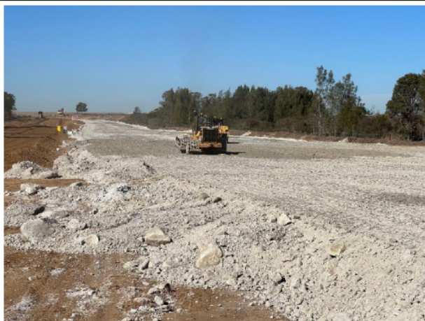
Cosgroves Creek - Sandstone is being used as fill for the formation
