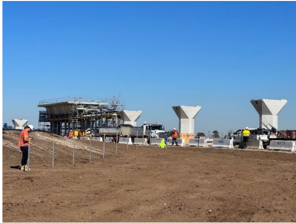
Luddenham North - Precast elements have been installed on the viaduct
