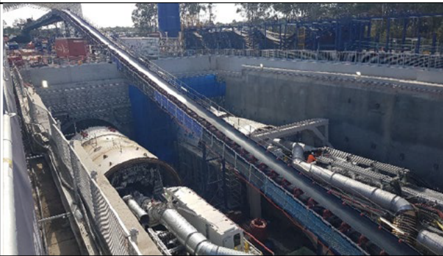
Orchard hills: View north at tunnel portal with TBM1 tunneling and TBM2 preparation.
