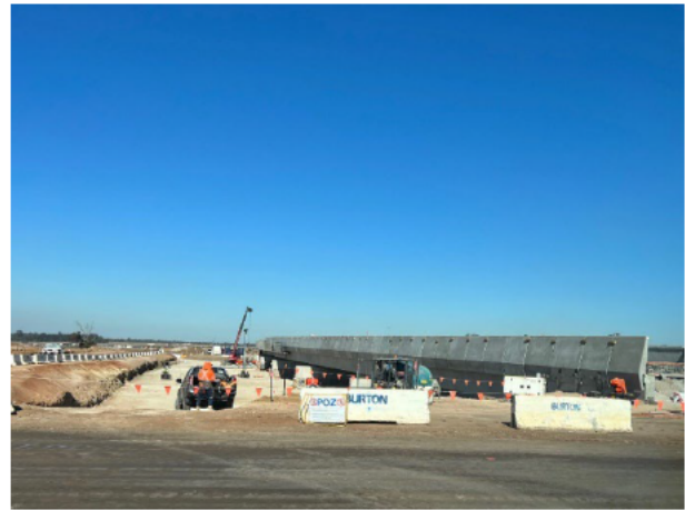
M12 Bridge - The parapets have been completed on the M12 bridge
