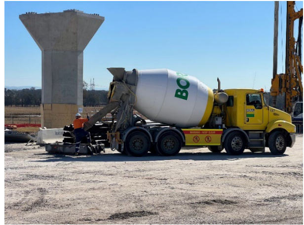
Luddenham North - Concrete washout trays have been used at Luddenham North
