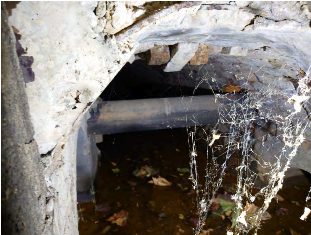
Figure 10 View north showing a sandstock brick barrel section of drain toward Parramatta River, visible beneath the modern stormwater grate shown in Figure 9.
