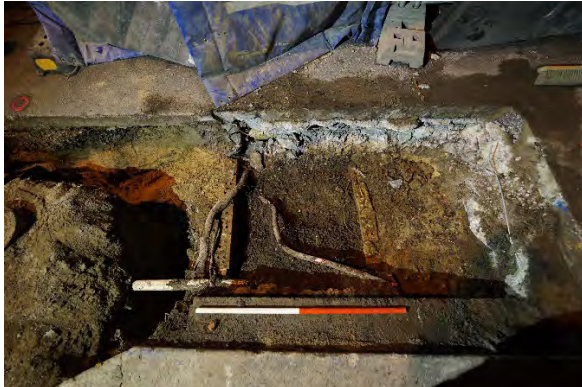
Figure 8 View south showing a machine-made brick section of drain, filled with a modern mix of historic topsoil and clay to the west and within the drain, and builder's sand to the east.
