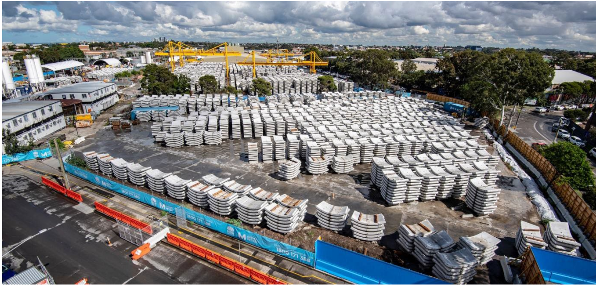
Figure 4-2 Photo of the tunnel segment storage area at Marrickville for the Sydney Metro City & Southwest project (indicative example of the proposed facility within Western Sydney International)
