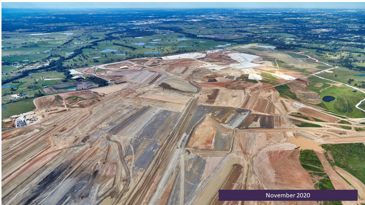
Figure 5-1 Major Earthworks progress on WSA CIZ
