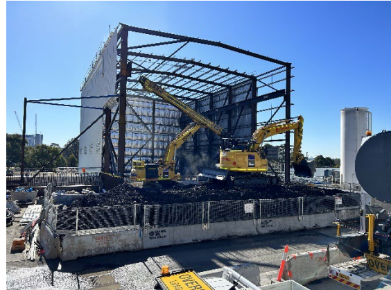
Figure 2.2: Westmead site – Station Box excavation with acoustic shed construction
