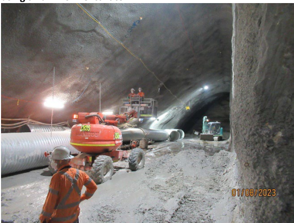
Figure 3.5 Station Cavern: Ongoing excavation by road headers.
