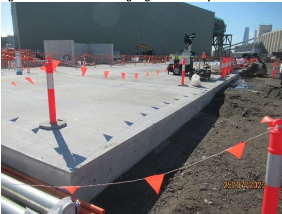
Figure 3.7 The Bays: Concrete works for the Spoil Shed
