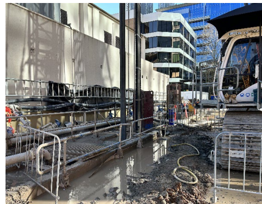
Figure 2.6: Parramatta Site – D-Wall excavation with cutter adjacent to Roxy Theatre
