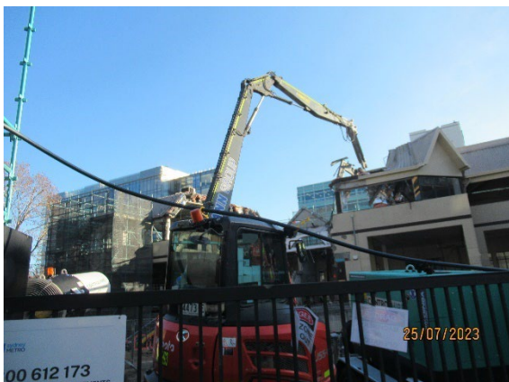
Figure 3.1 Pyrmont East: Ongoing hard demolition works
