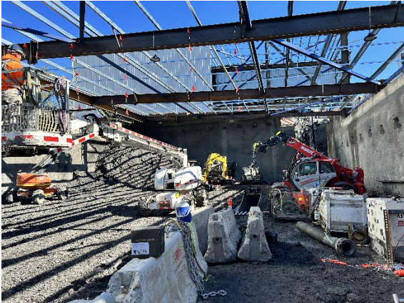
Figure 2.1: Westmead Site –Acoustic shed construction at western end of Station Box
