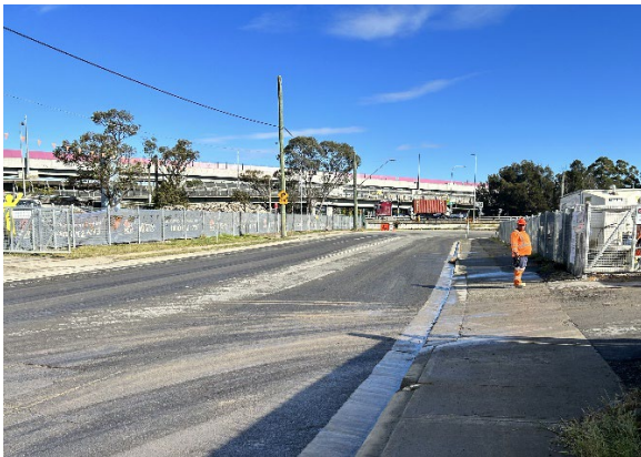
Figure 2.12 – Clyde MSF Site – One of the Duck Creek diversion excavations progressing
