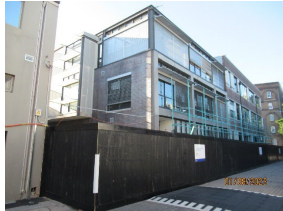
Figure 3.4 Pyrmont St West: A Class Hoarding constructed on Paternoster Row
