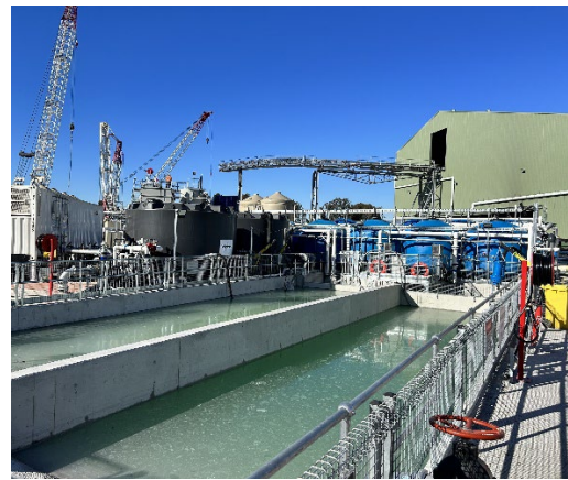
Figure 2.10: Rosehill Site – 50L/s Water Treatment Plant commissioning
