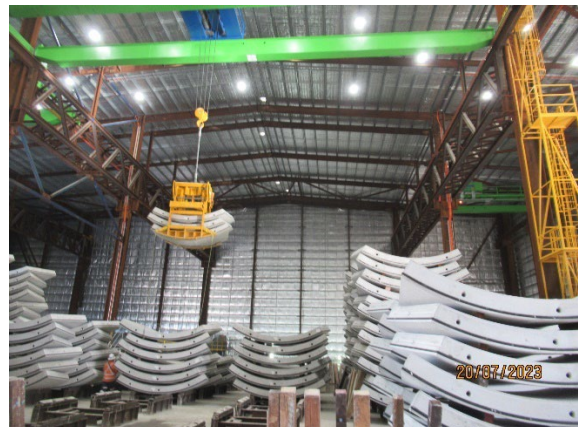
Figure 1 2 Loading of segments into the station box for delivery to the TBM. (The Bays).
