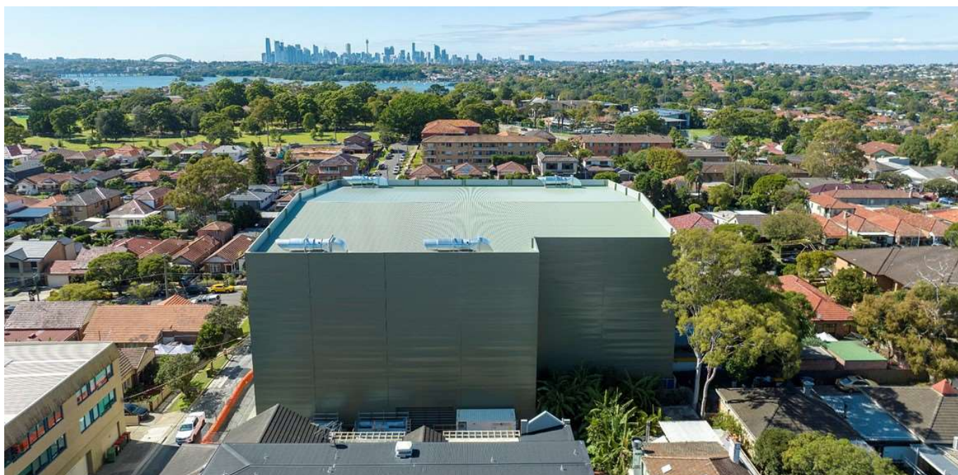
Figure 5-4 Five Dock east acoustic shed and surrounding buildings.
