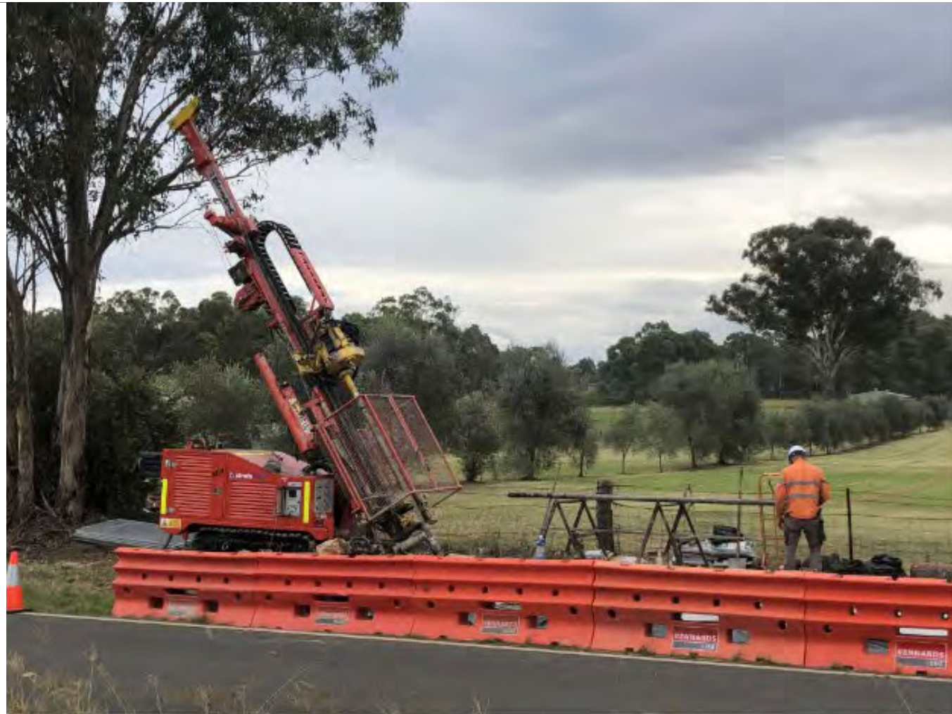
Figure 3: Example of a borehole/monitoring well set-up required for the proposed geotechnical services
