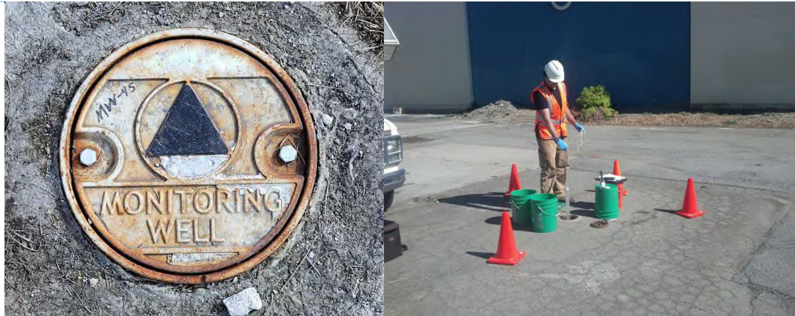
Figure 4: Example of an installed monitoring well (left) and periodic monitoring well sampling (right)
